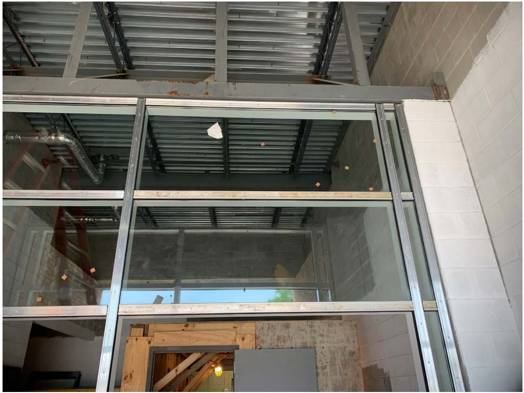
Figure 3 – Curtain Wall Installed (awaiting aluminum covers)
