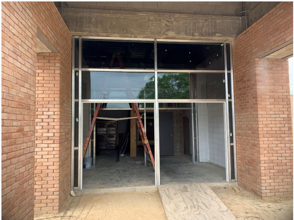
Figure 2 – Curtain Wall Installed (awaiting aluminum covers)
