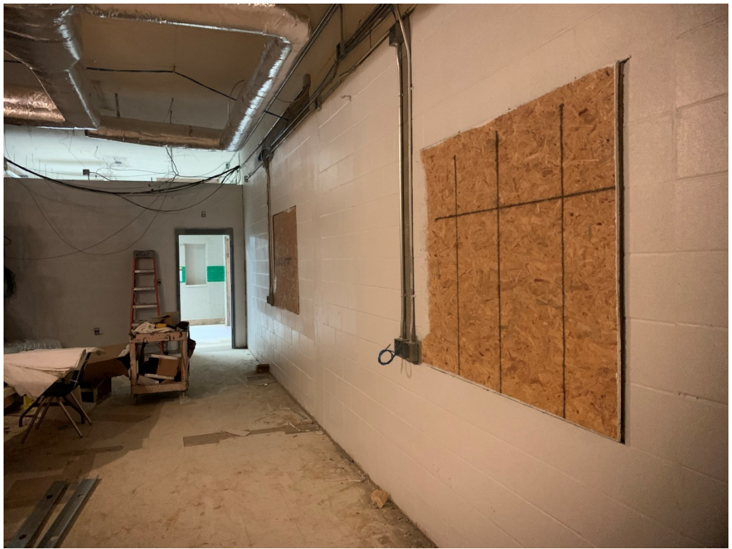
Figure 6 – Concessions Area Conduit Rerouted
