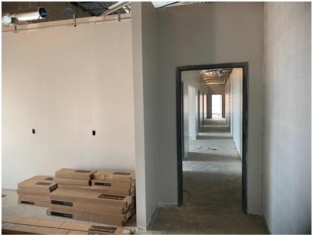
Figure 4 – Office Area Progress
