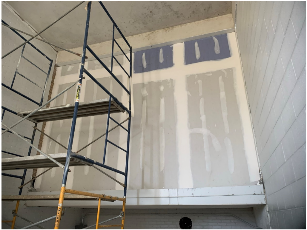
Figure 5 – Drywall Installed at Stair Upper Wall
