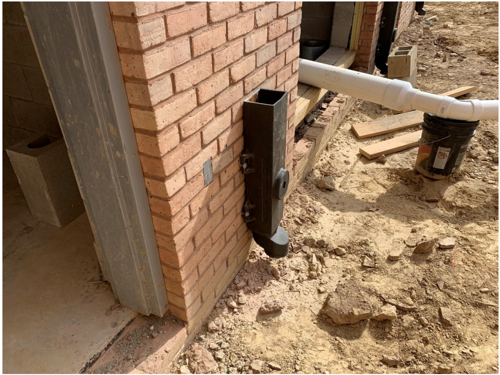
Figure 5 – Cast Iron Boots Installed
