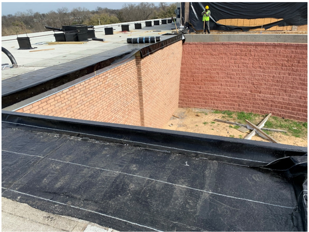
Figure 8 – Roof Work at Remodeled Wall
