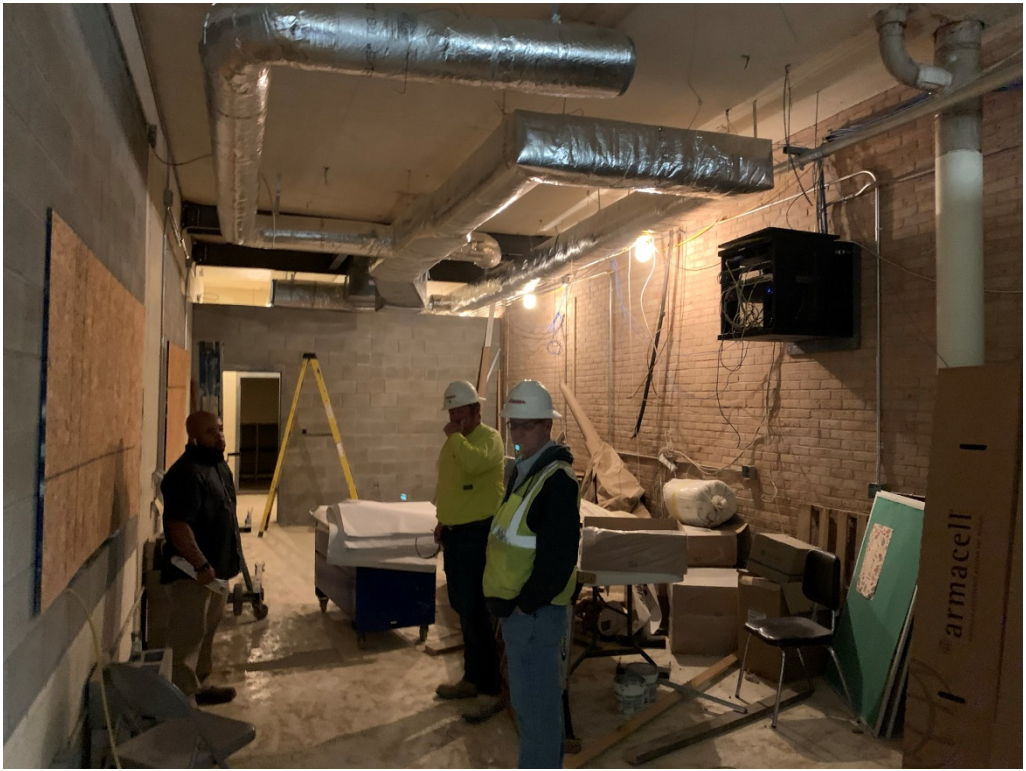
Figure 9 – Interior at Concessions
