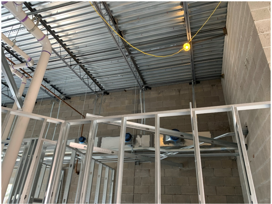
Figure 4 – Interior Service work is Ongoing
