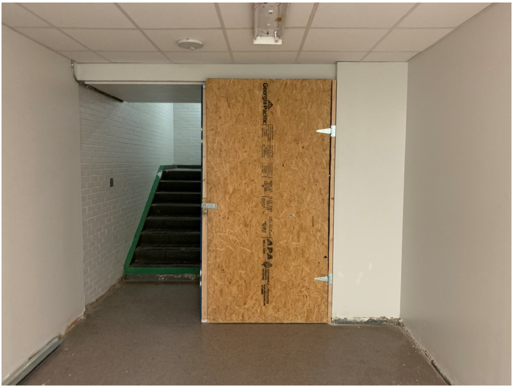
Figure 10 – Elevator work to wrap up ASAP
