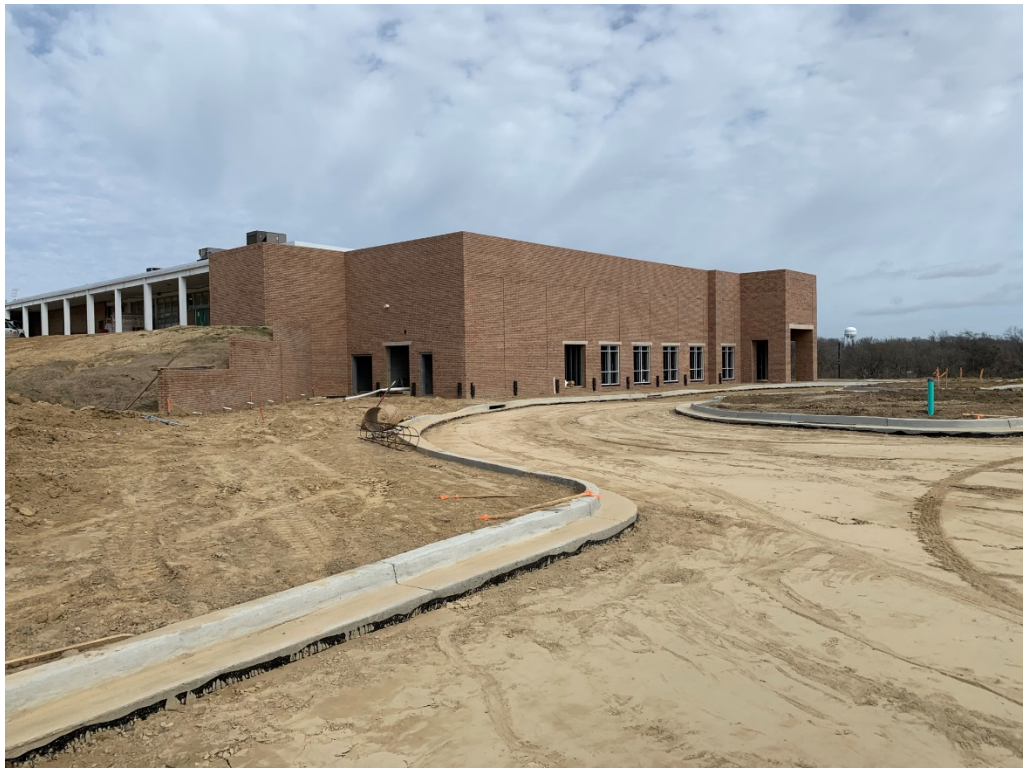
Figure 1 – Southeast Looking NW
