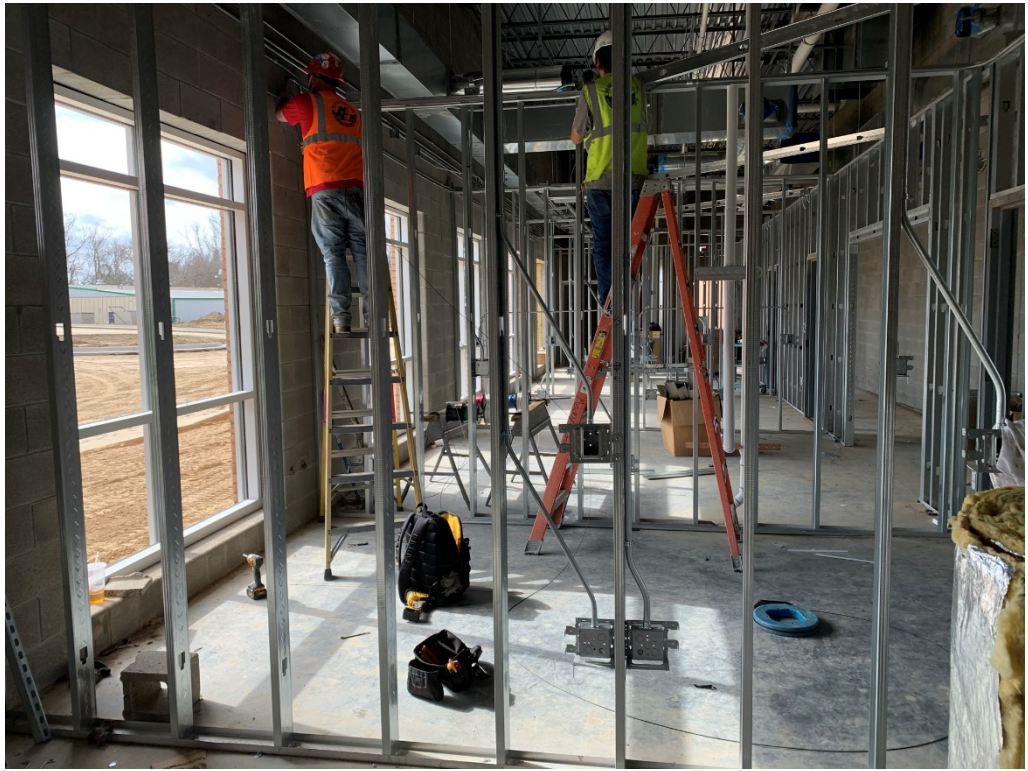
Figure 3 – Interior Service work is Ongoing
