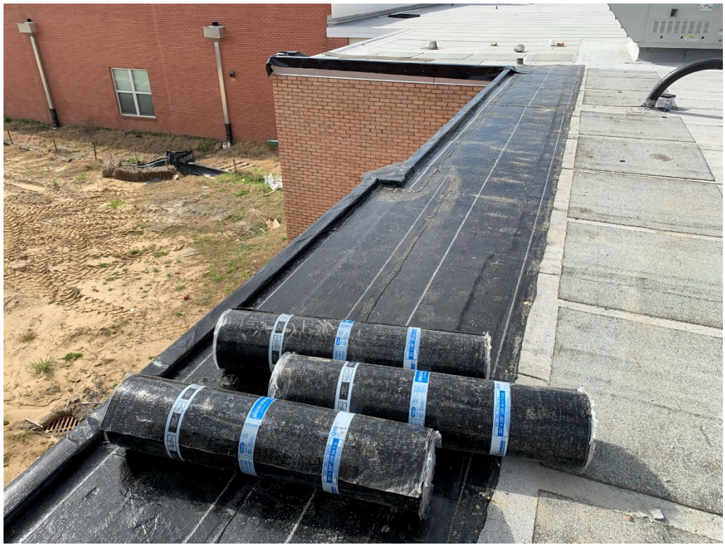
Figure 7 – Roof Work at Remodeled Wall
