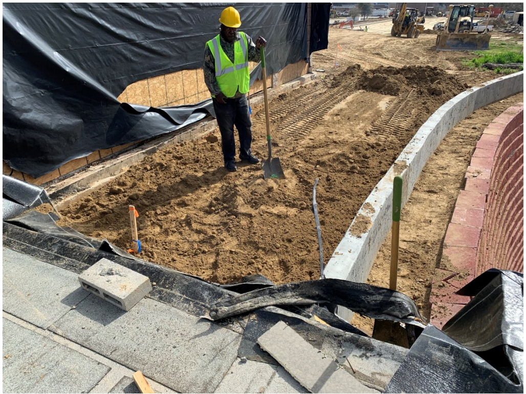
Figure 6 – Grading near Roof Edge
