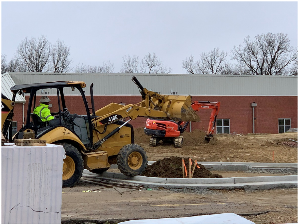
Figure 4 – Fill Dirt Installation
