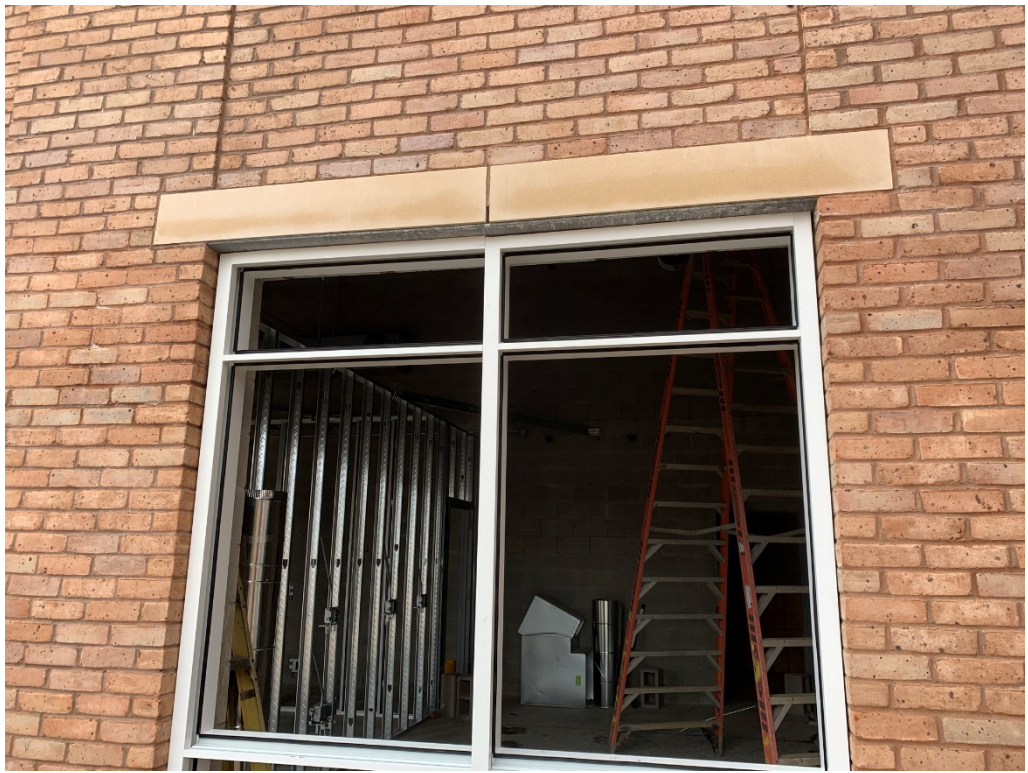
Figure 3 – Storefront Window Installed
