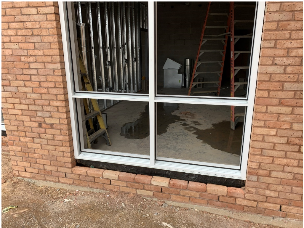
Figure 2 – Storefront Window Installed
