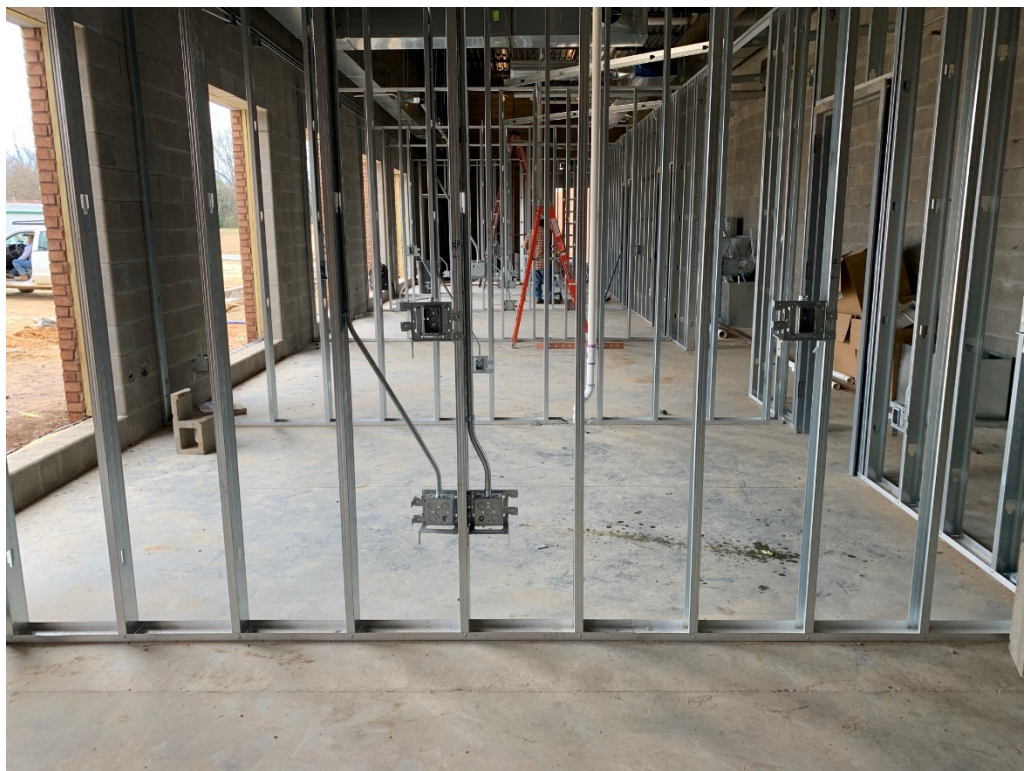
Figure 4 – Electrical Rough In is Ongoing
