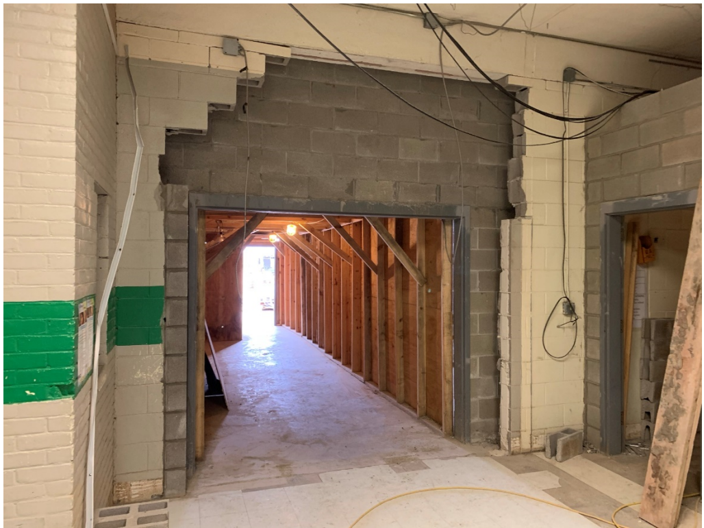
Figure 11 – Addition Entry from Main building
