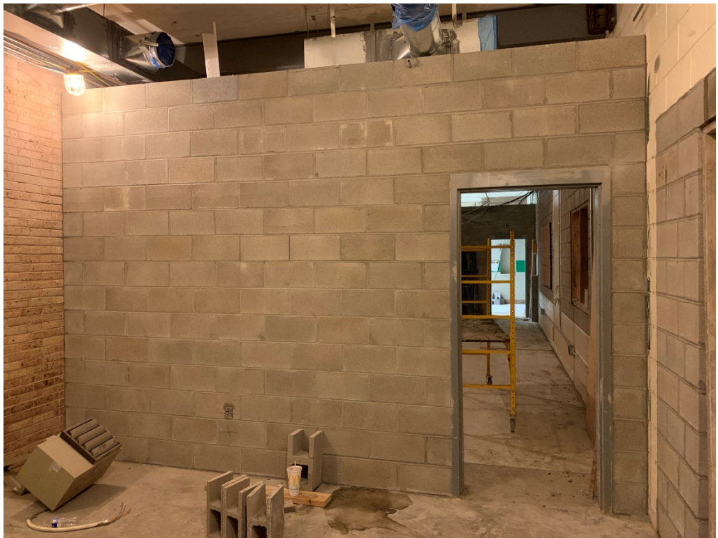
Figure 7 – Block work at new concessions area
