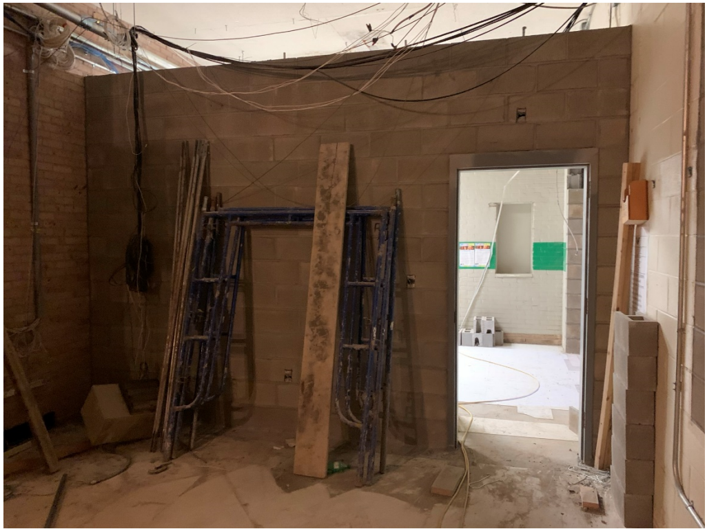
Figure 9 – Block work at new concessions area
