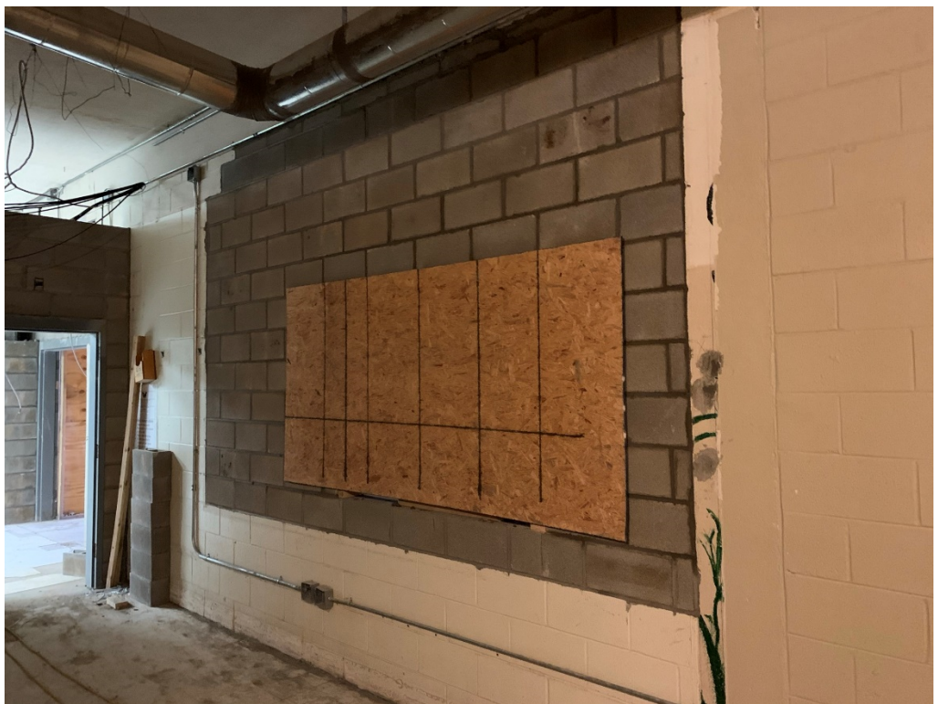
Figure 8 – Block work at new concessions area
