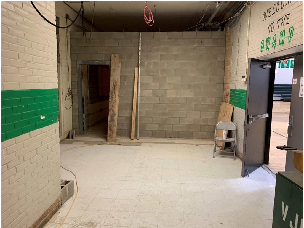
Figure 10 – Block work at new concessions area
