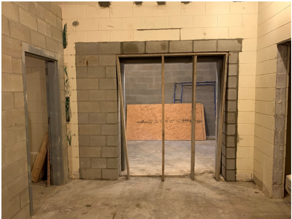
Figure 6 – Block work at new concessions area
