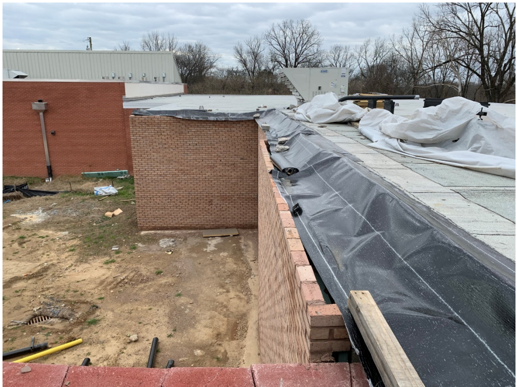
Figure 14 – Roof Awaiting Tie In
