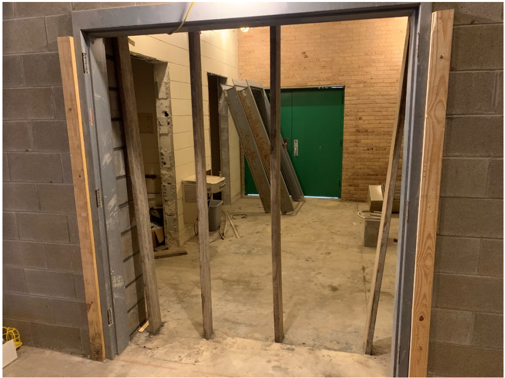
Figure 5 – Block work at new concessions area
