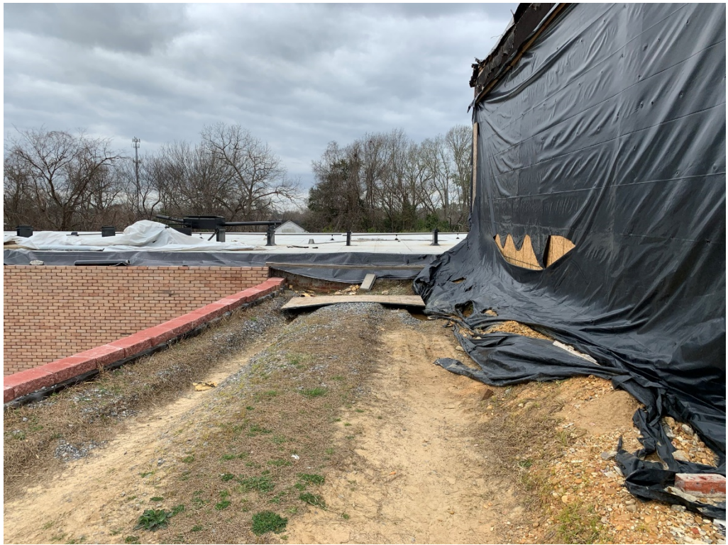
Figure 13 – Roof Awaiting Tie In
