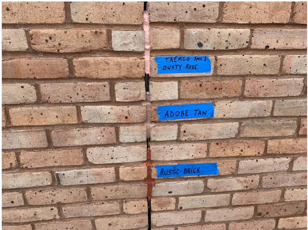
Figure 3 – Test Sealant Colors at Exterior Brick
