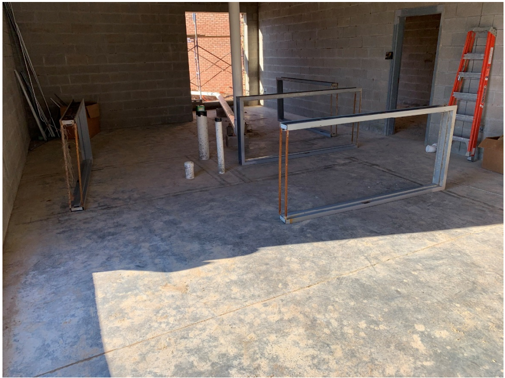
Figure 5 – Interior Doors Ready to be Set
