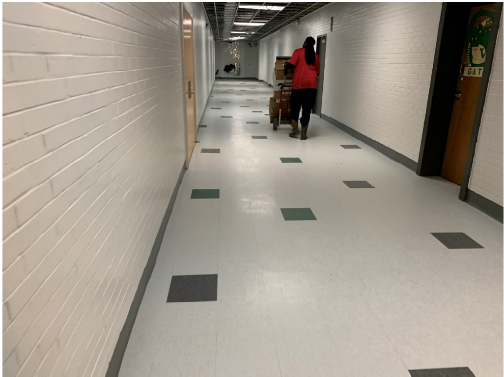
Figure 7 – New Flooring Installed
