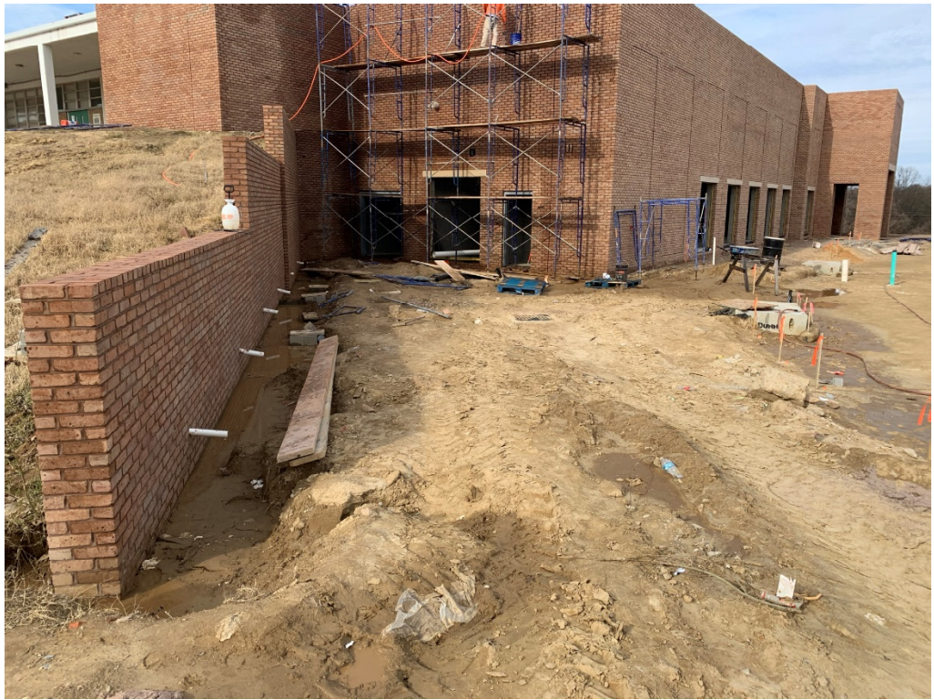
Figure 1 – Brick Work Appears Complete and Acceptable
