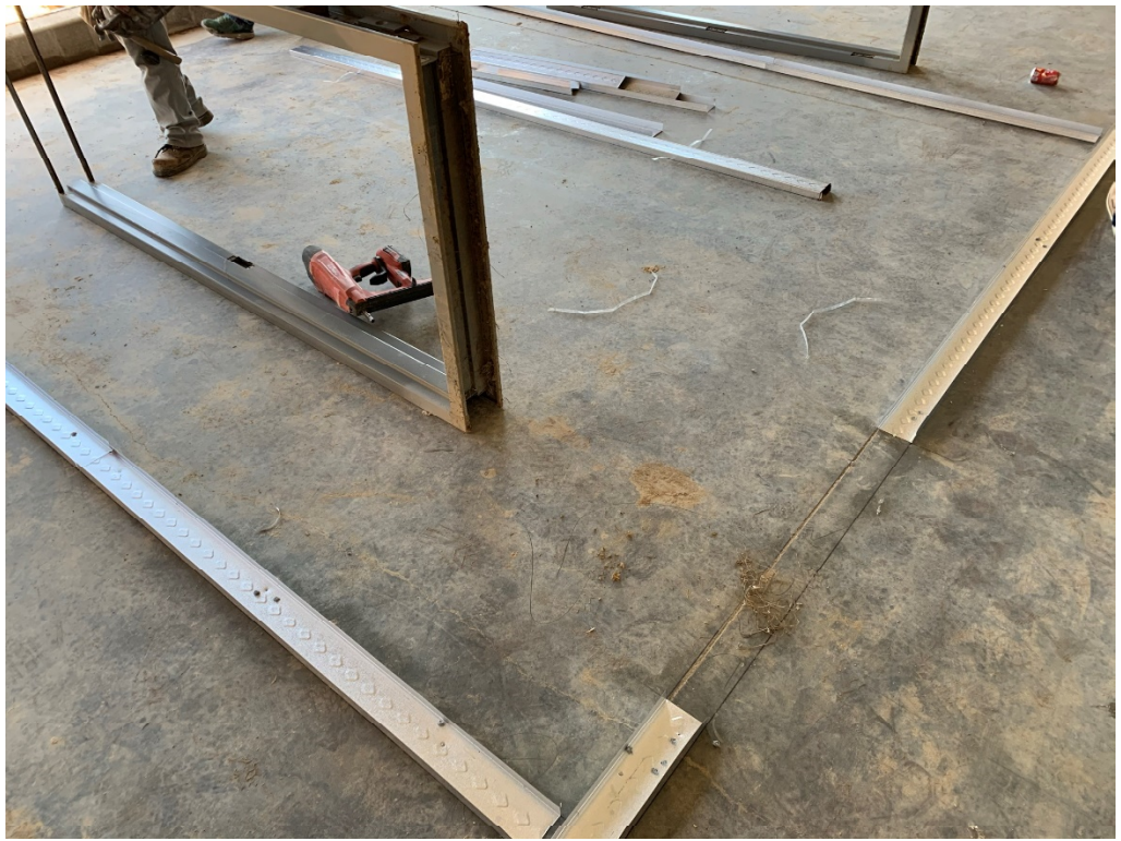
Figure 4 – Interior Framing Has Begun
