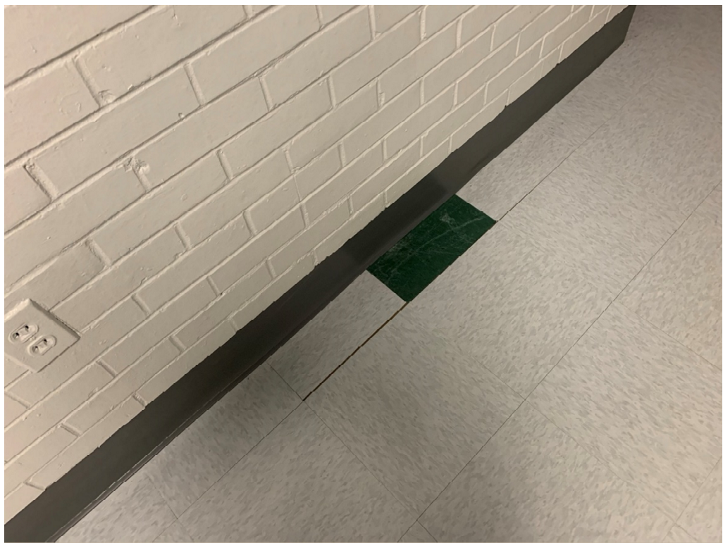
Figure 8 – Some Tiles need to be reset so that there is no gap
