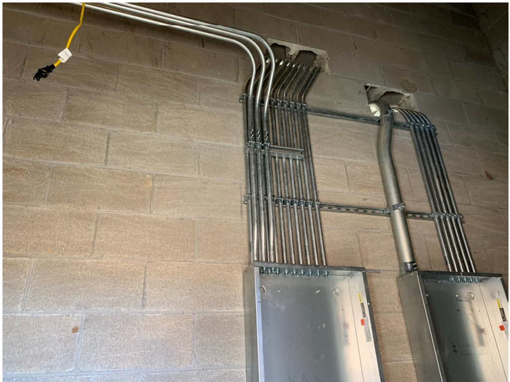
Figure 6 – Panel Boxes Installed with Conduit
