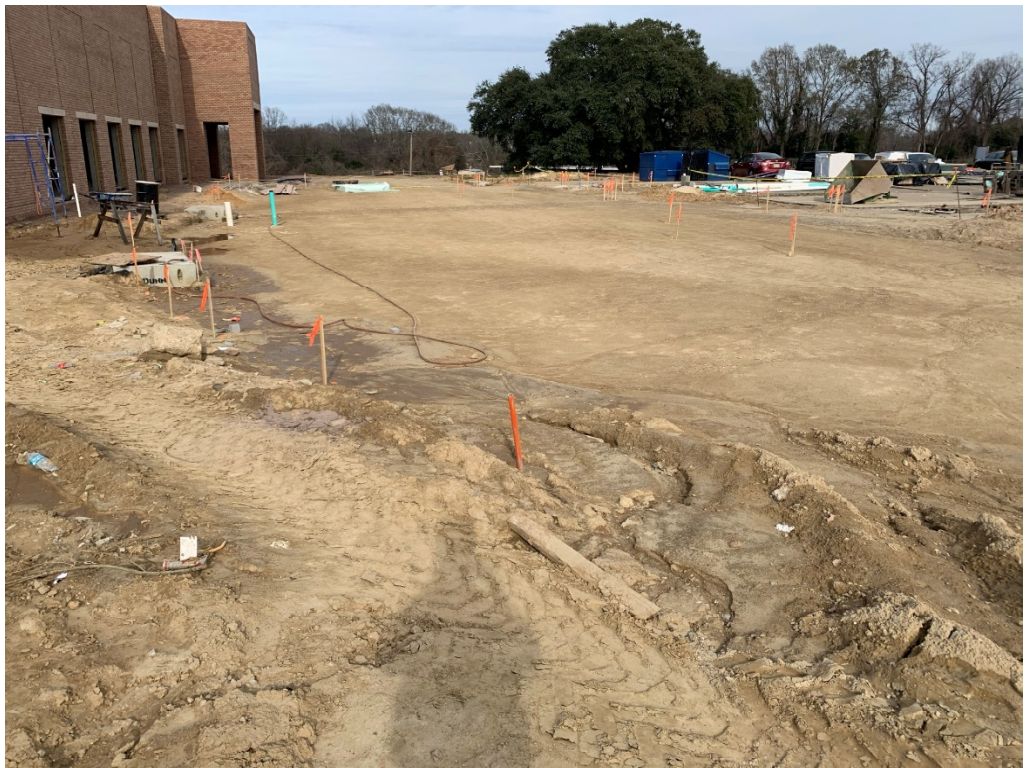
Figure 2 – Curbs Staked Out and Ready for Concrete
