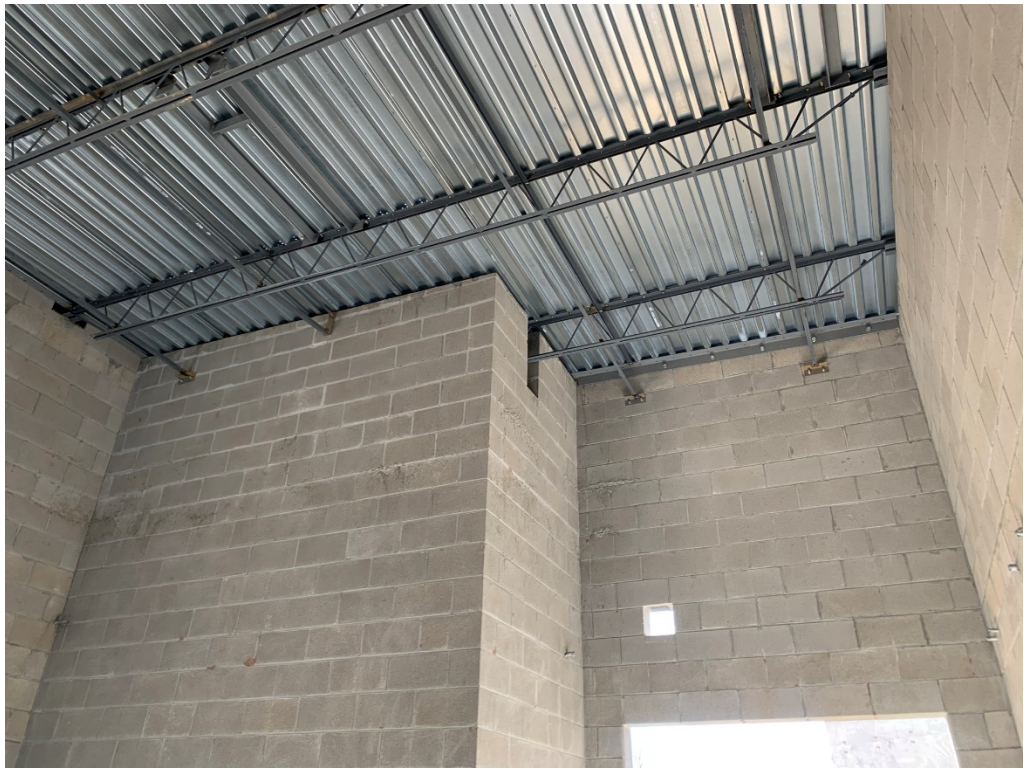
Figure 13 – Structure above Councs./Vault Area
