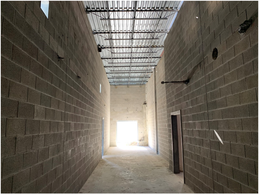
Figure 11 – Corridor 202 Structural Work
