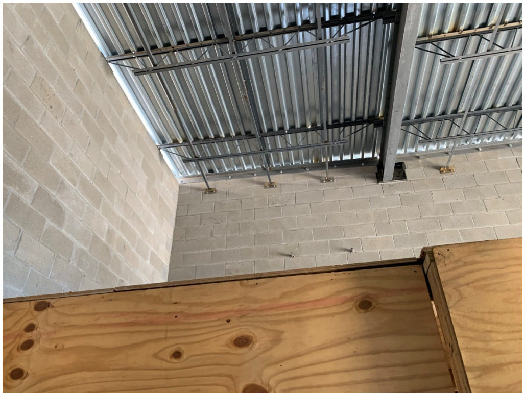
Figure 10 – Corridor 202 Structural Work
