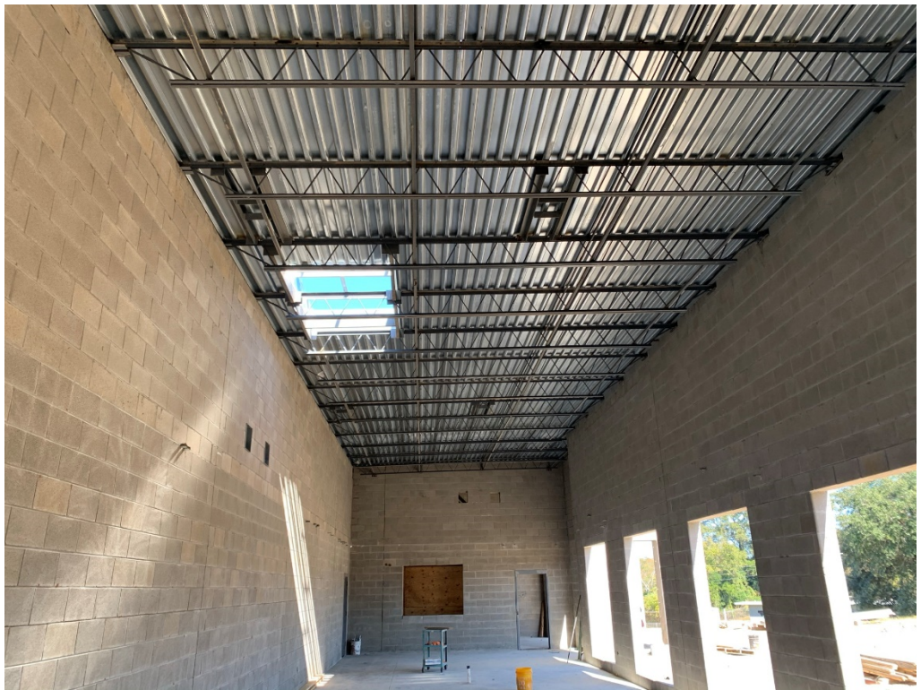
Figure 14 – Structure above Office Admin Area
