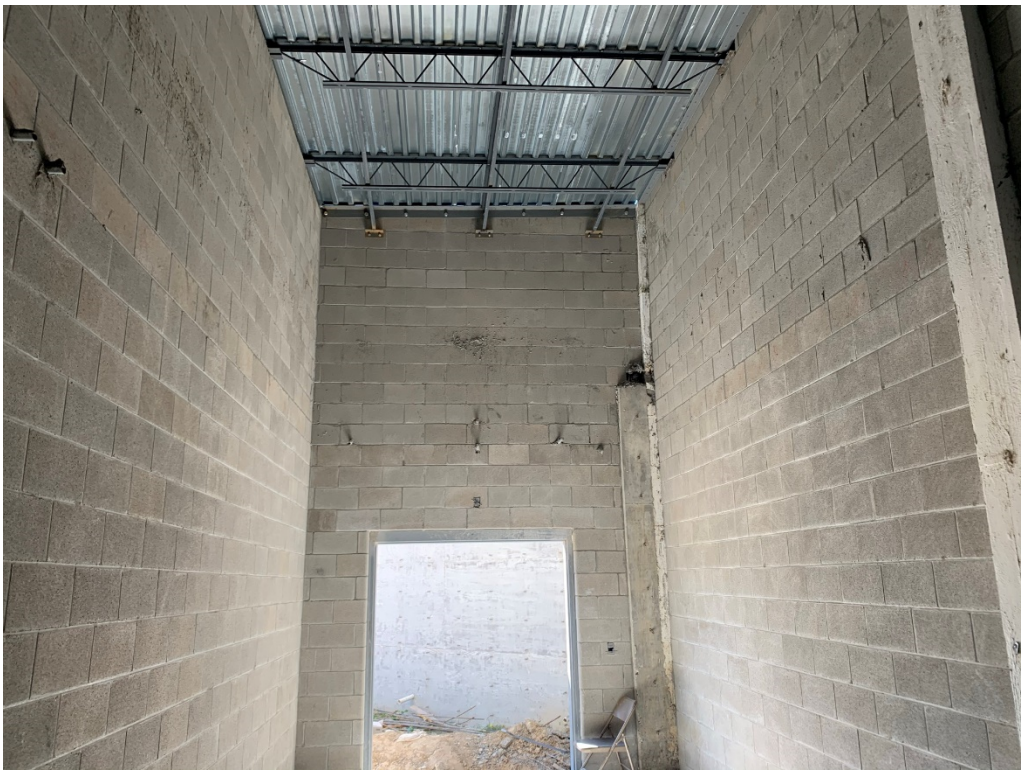
Figure 12 – Corridor 202 Structural Work
