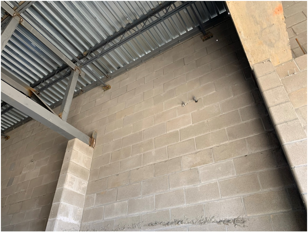
Figure 7 – Corridor 202 Structural Work
