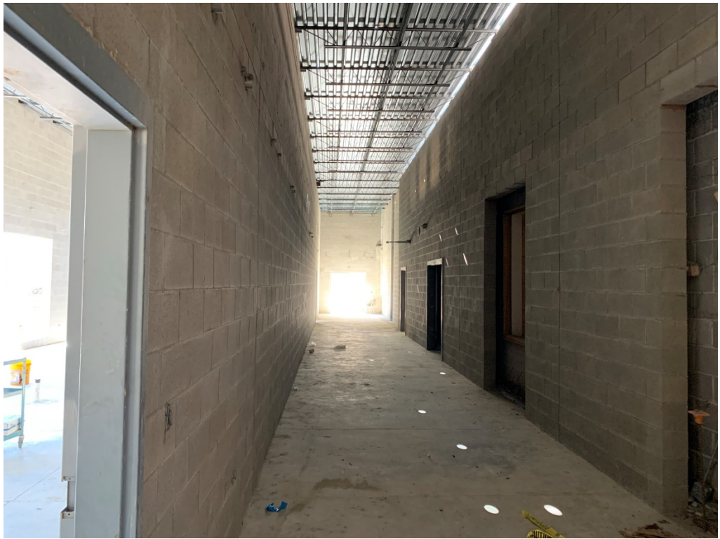
Figure 9 – Corridor 202 Structural Work
