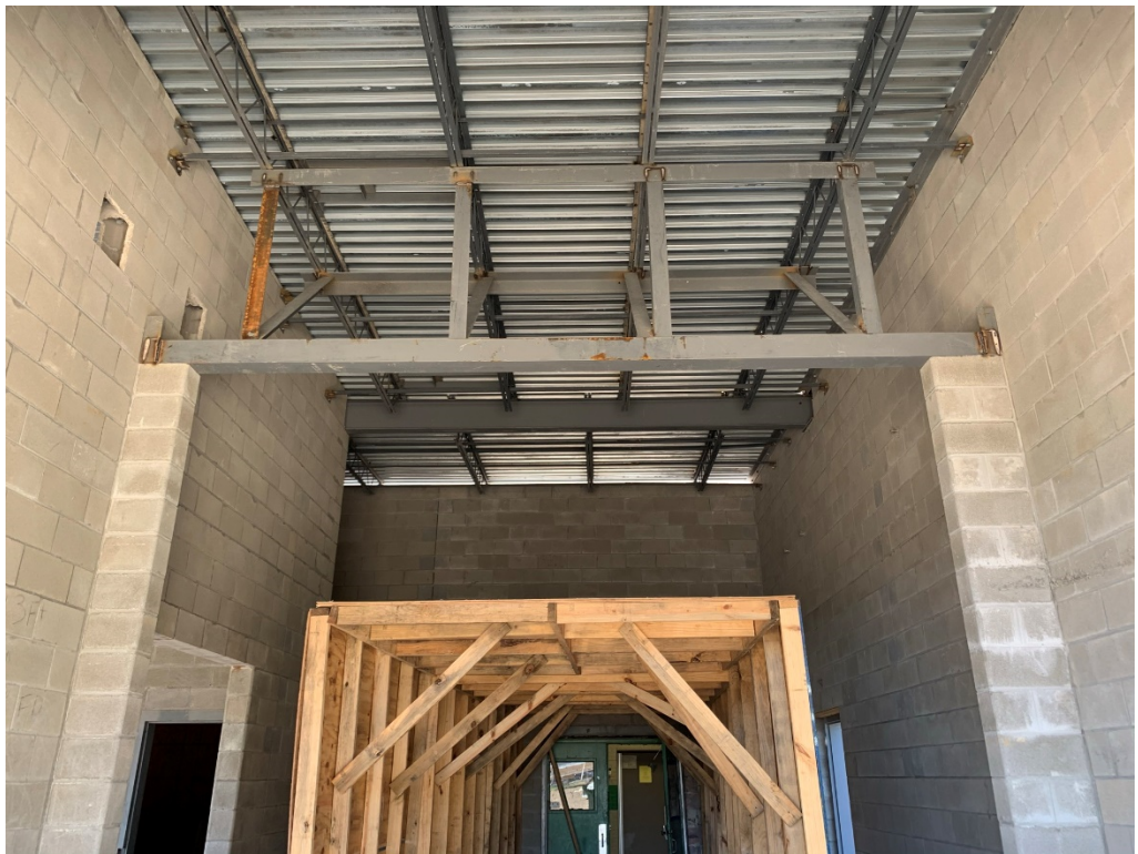
Figure 6 – Corridor 202 Structural Work
