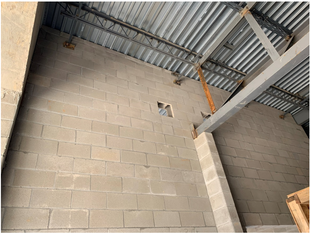
Figure 8 – Corridor 202 Structural Work
