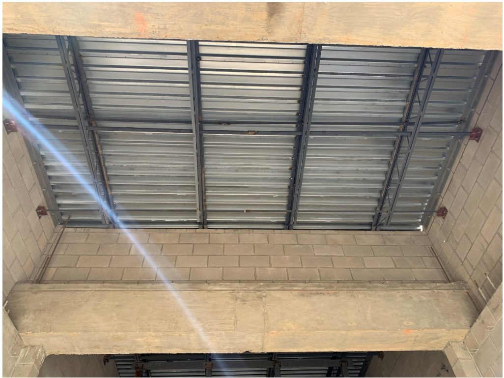
Figure 5 – Entrance Foyer Structure Installed
