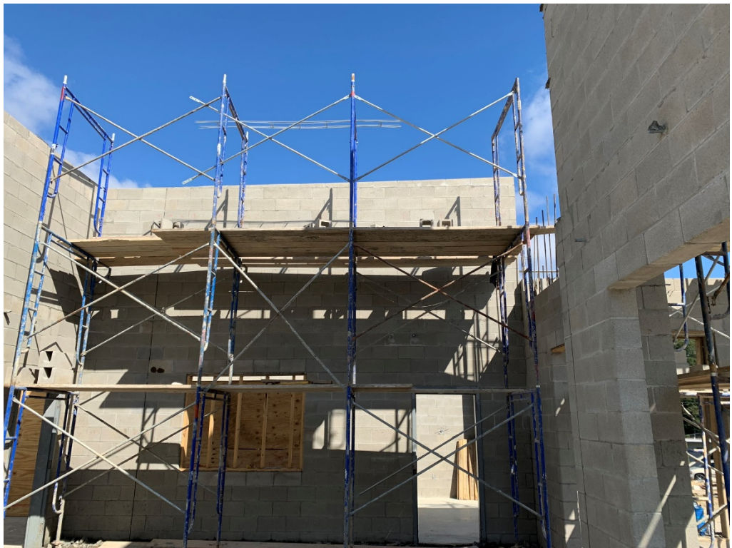
Figure 10 – Sloped CMU Block at Top of Wall
