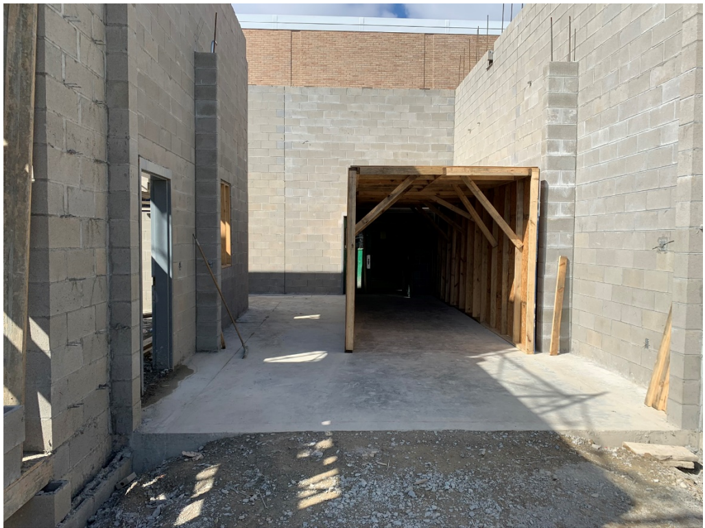
Figure 11 – Temporary Enclosure for Useable Entry at Existing Building
