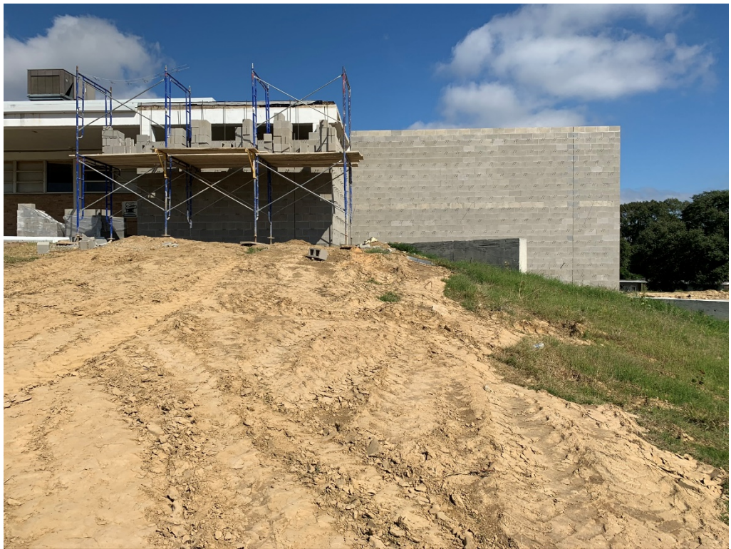
Figure 2 – South Side of the Addition Looking North
