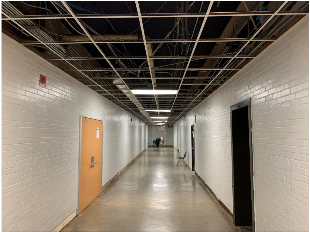
Figure 13 – Interior Grid Installed at Corridor E-200
