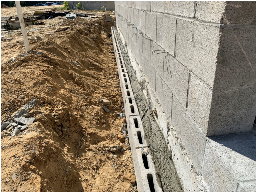
Figure 9 – Block Cavity Filled Below Grade
