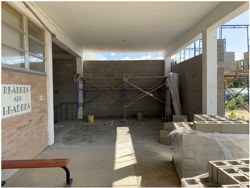
Figure 3 – Existing Stair 301A Enclosure
