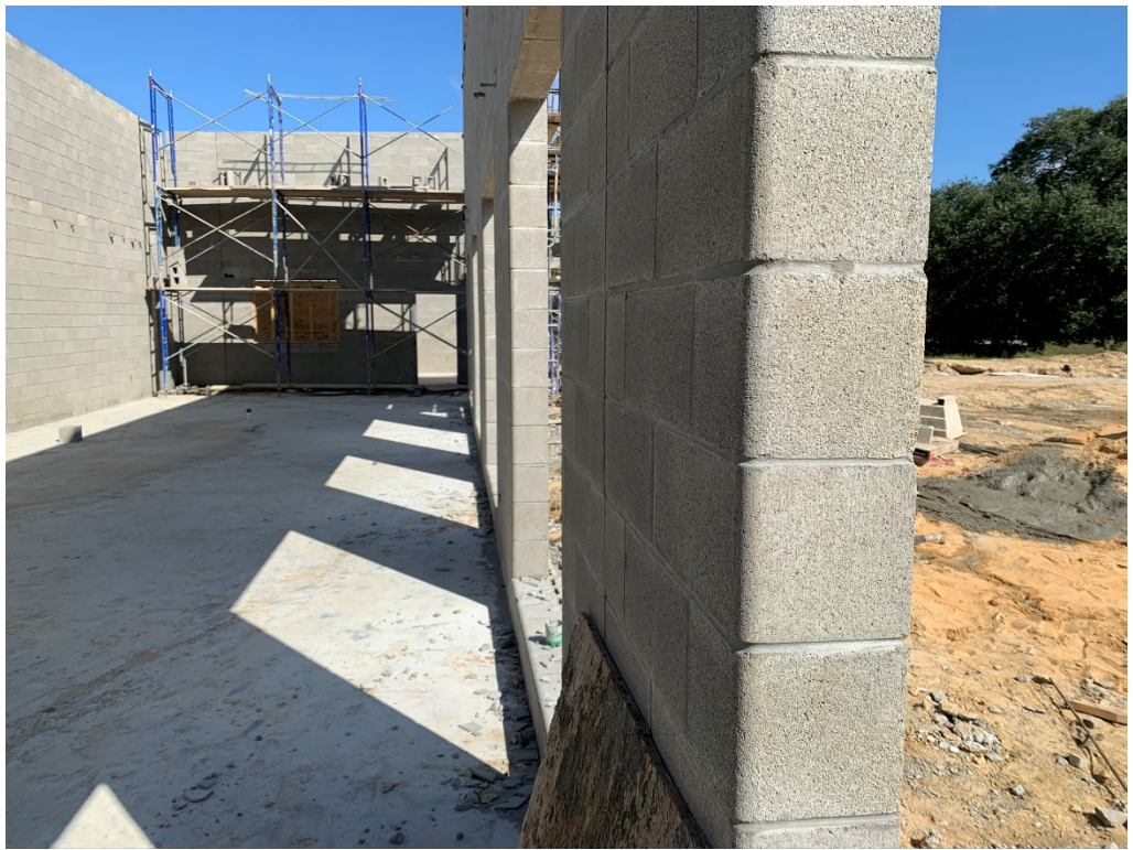
Figure 8 – Exterior Window Block Detail
