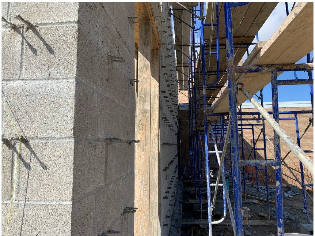
Figure 12 – Exterior Blocking at North of Addition
