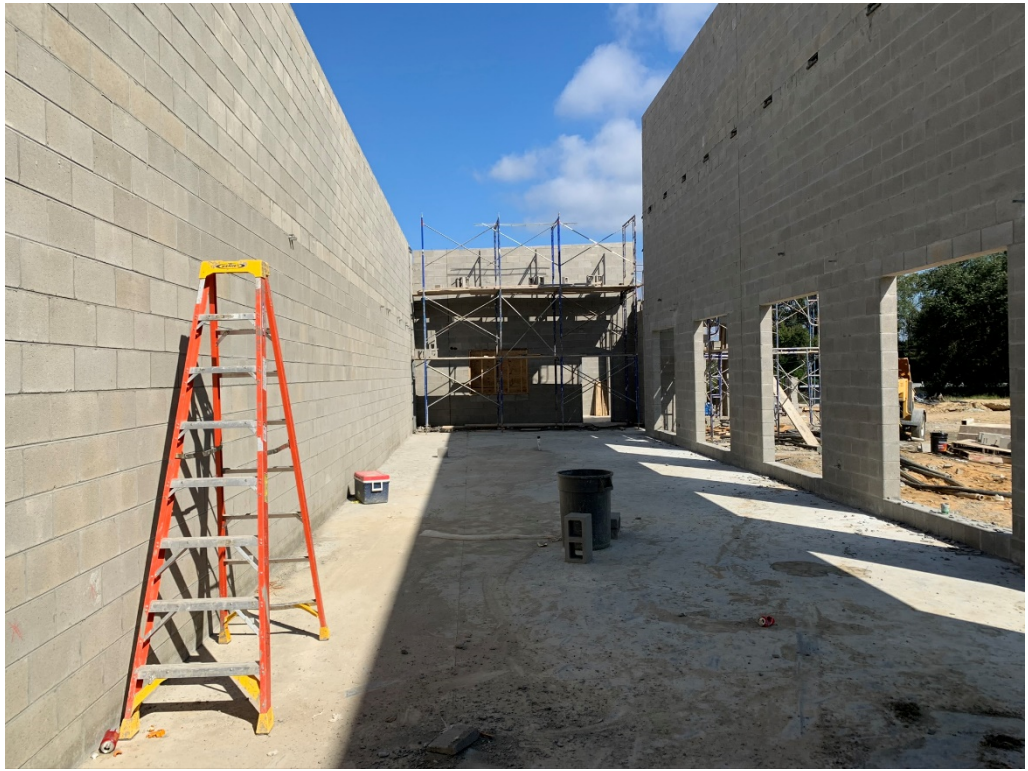
Figure 7 – Main Office Area Blocked IN
