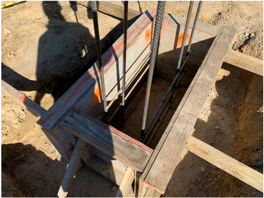
Figure 3 – Footing Reinforcing
