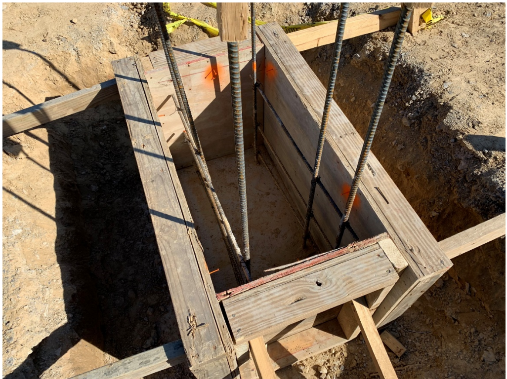
Figure 2 – Footing Reinforcing
