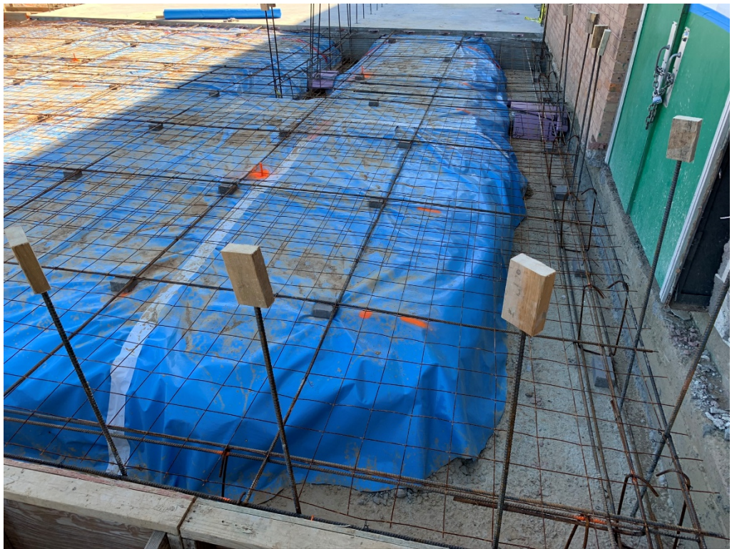
Figure 6 – Northwest Edge of Slab
