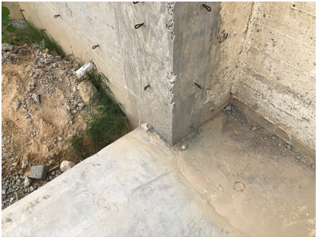
Figure 4 – Footing Install Ongoing
