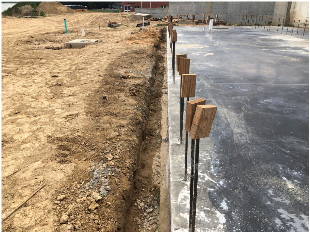
Figure 6 – Concrete Slab Poured
