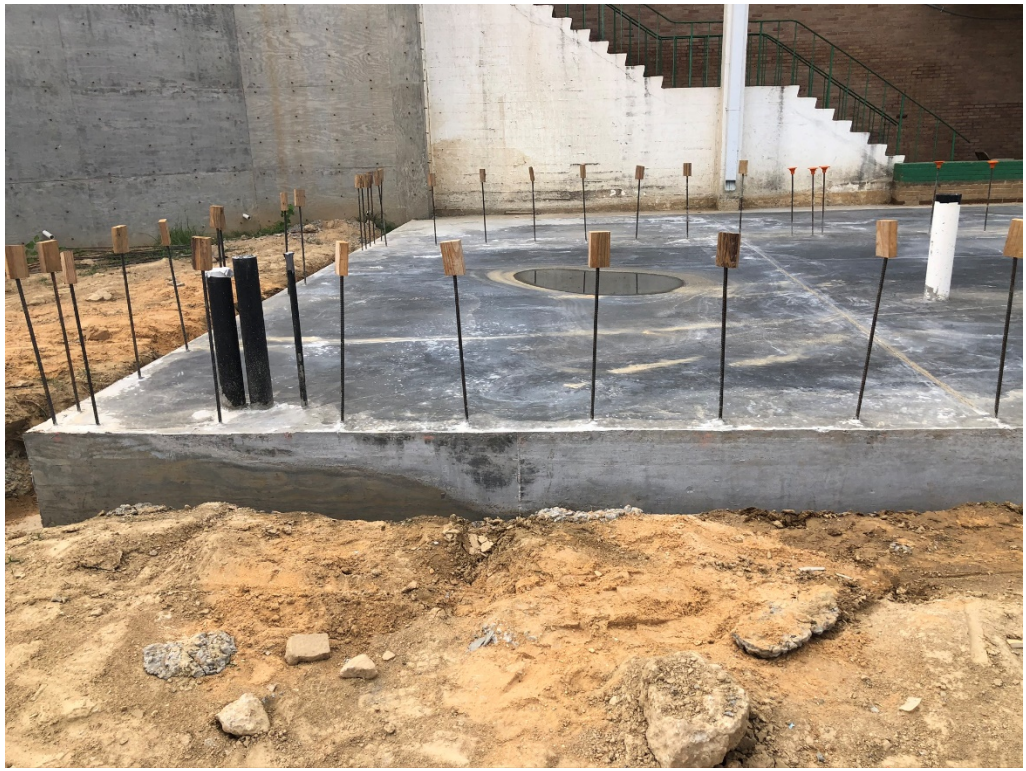
Figure 1 – Concrete Slab Poured
