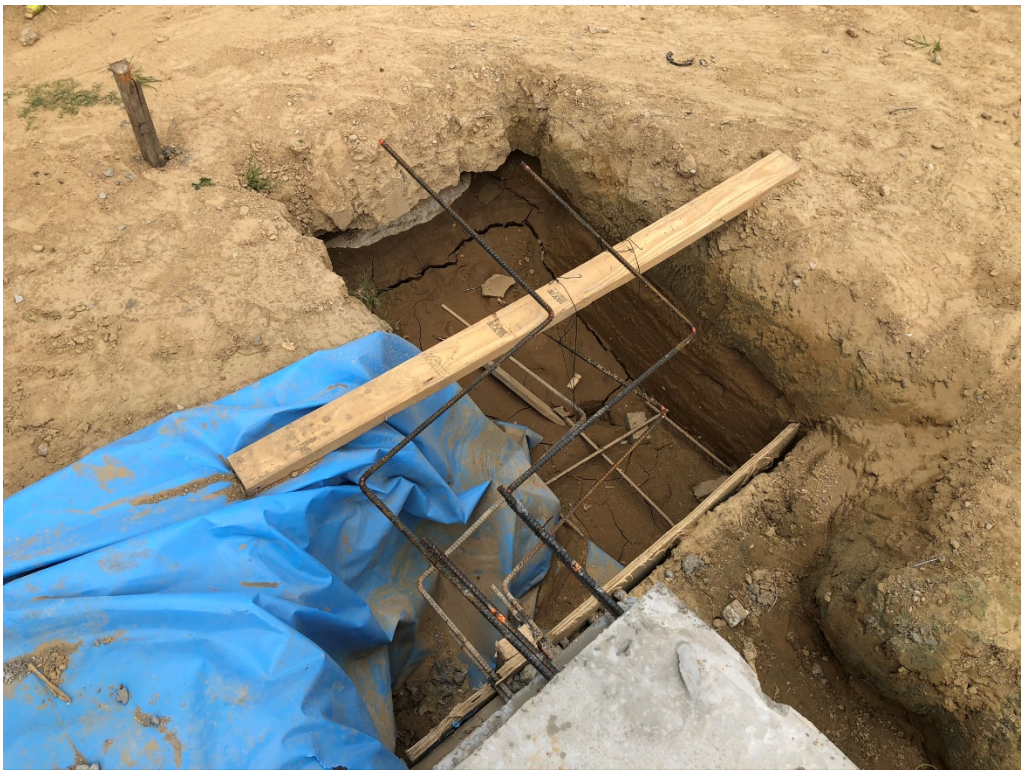
Figure 8 – Slab to be Continued
