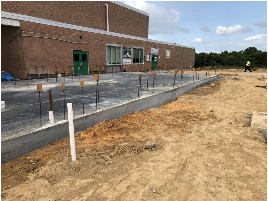
Figure 2 – Concrete Slab Poured
