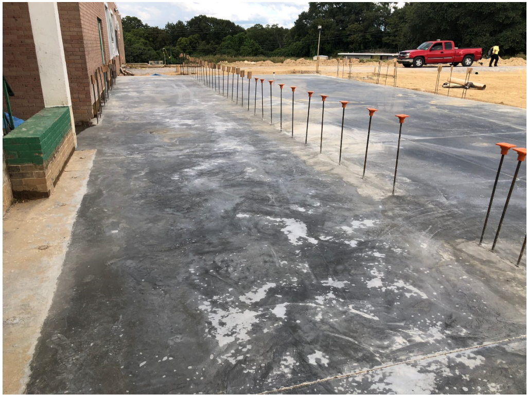
Figure 3 – Concrete Slab Poured
