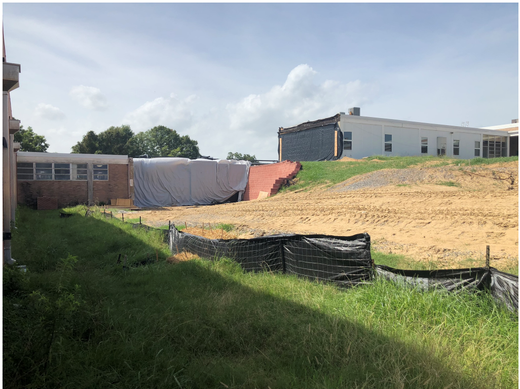
Figure 14 – Exterior Build Site
