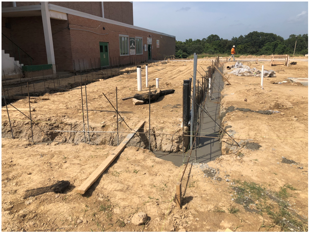
Figure 1 – Footing Install Ongoing
