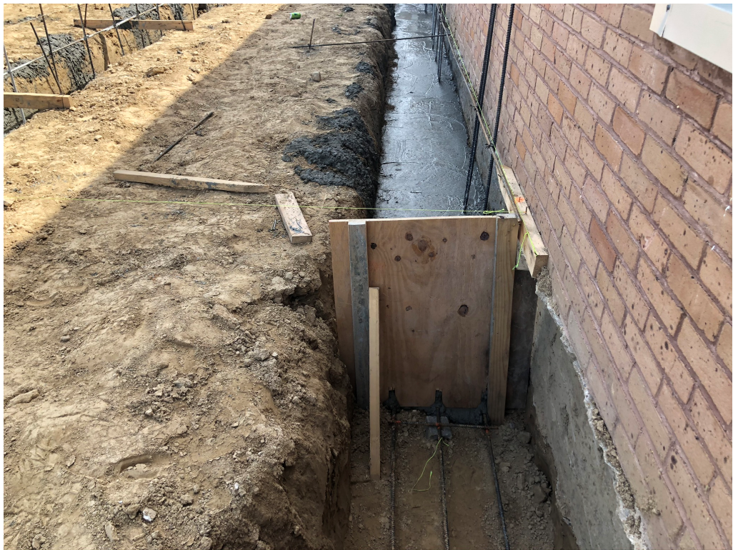
Figure 4 – Footing Install Ongoing
