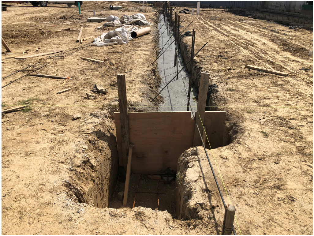
Figure 5 – Footing Install Ongoing
