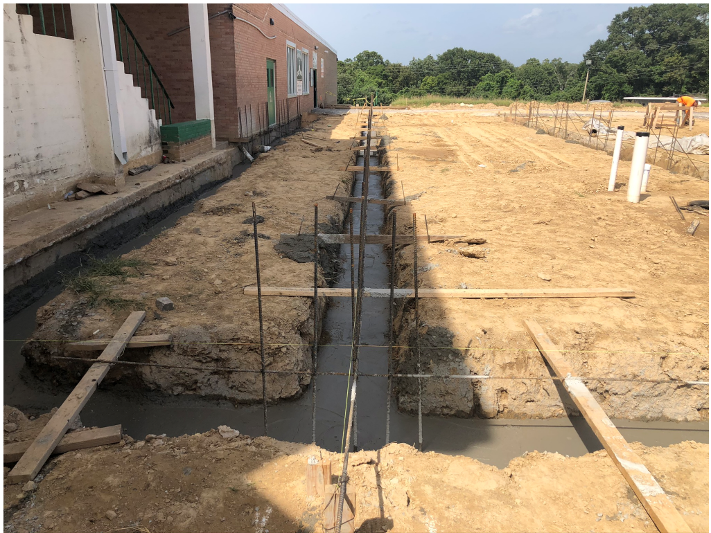
Figure 2 – Footing Install Ongoing
