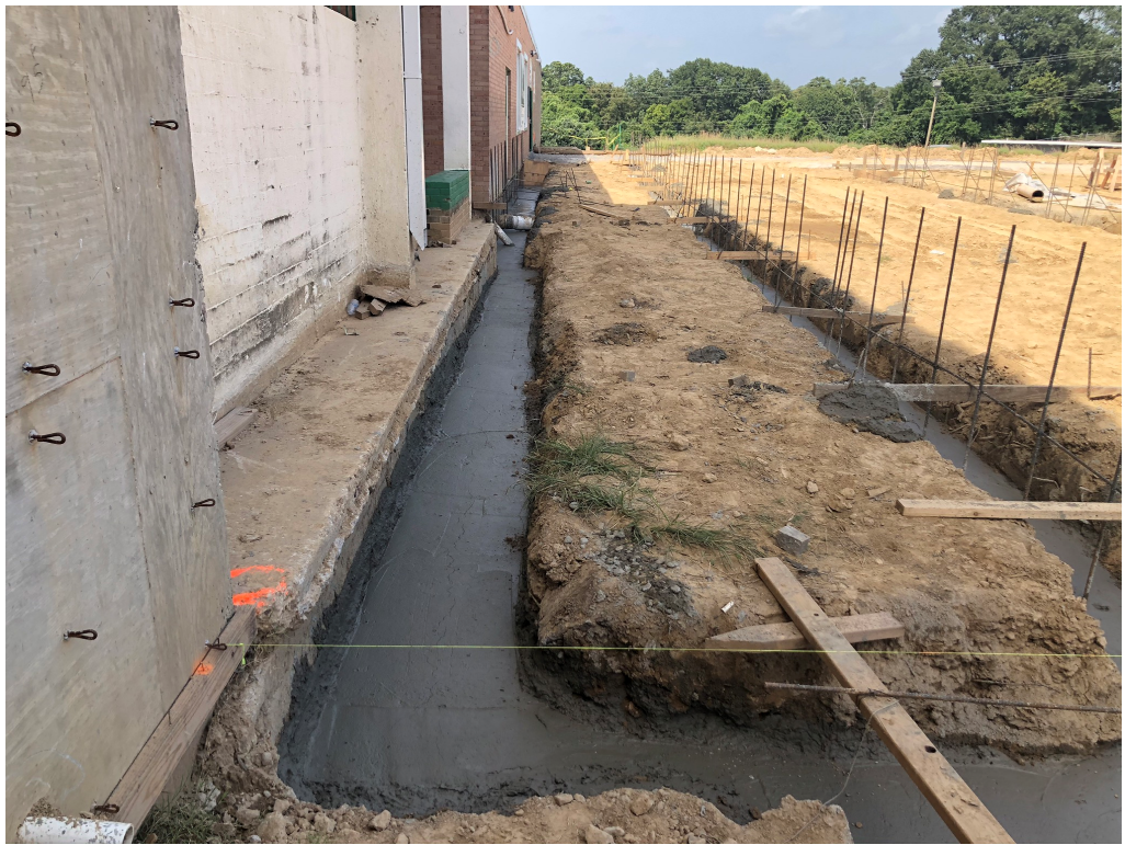
Figure 3 – Footing Install Ongoing
