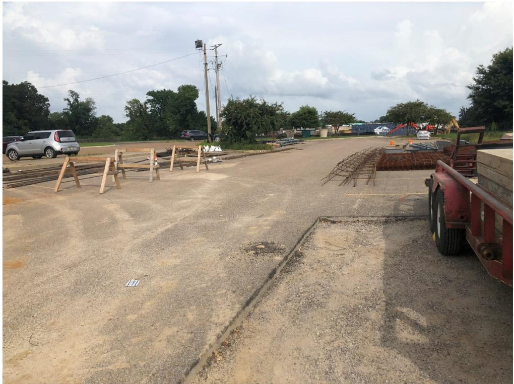
Figure 1 – Rebar and Structural Steel Stored on Site
