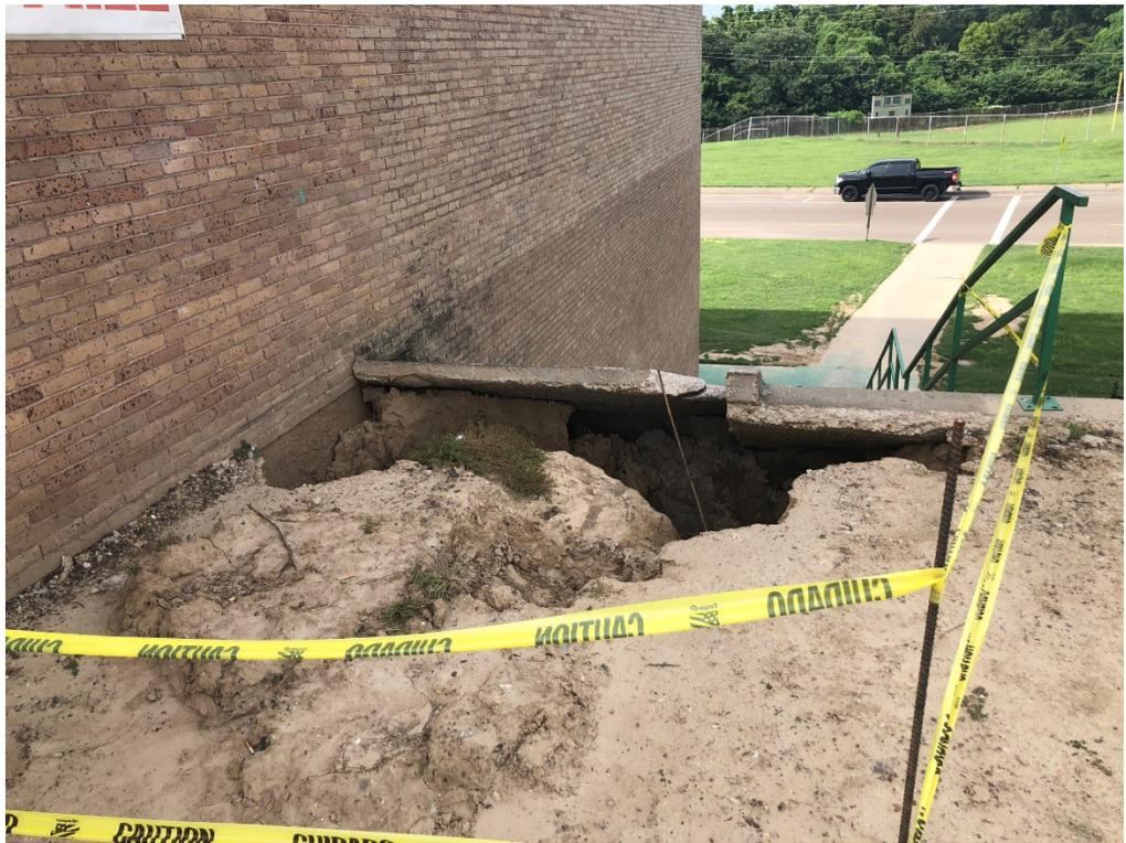
Figure 6 – Erosion at North Side of Addition
