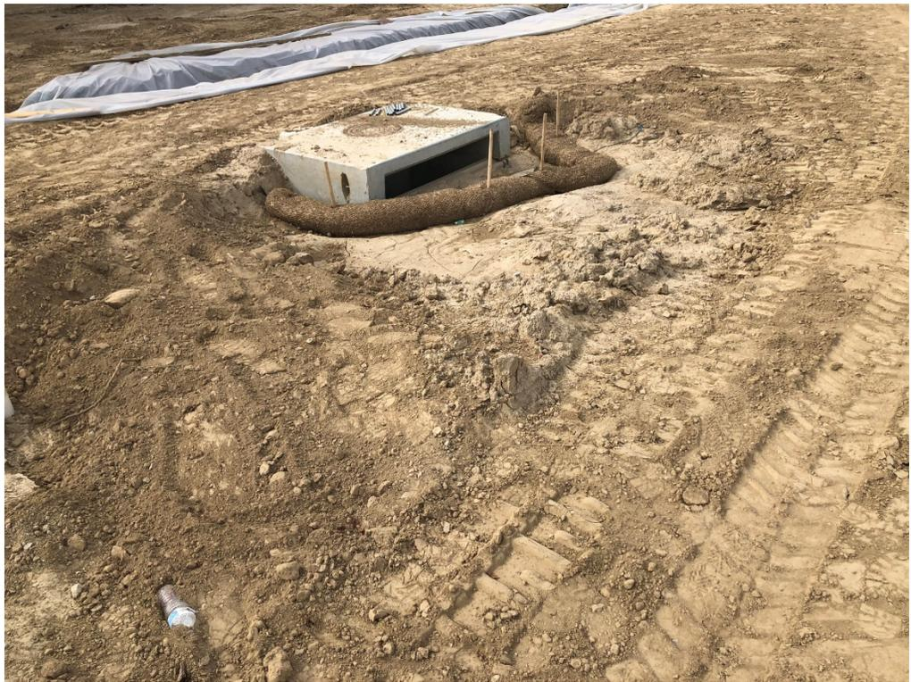
Figure 2 – Waddles in Place at Storm Sewer
