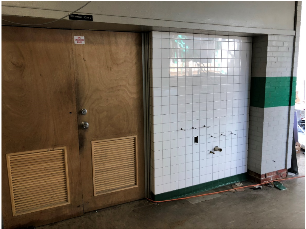
Figure 11 – New Tile at EDF's
