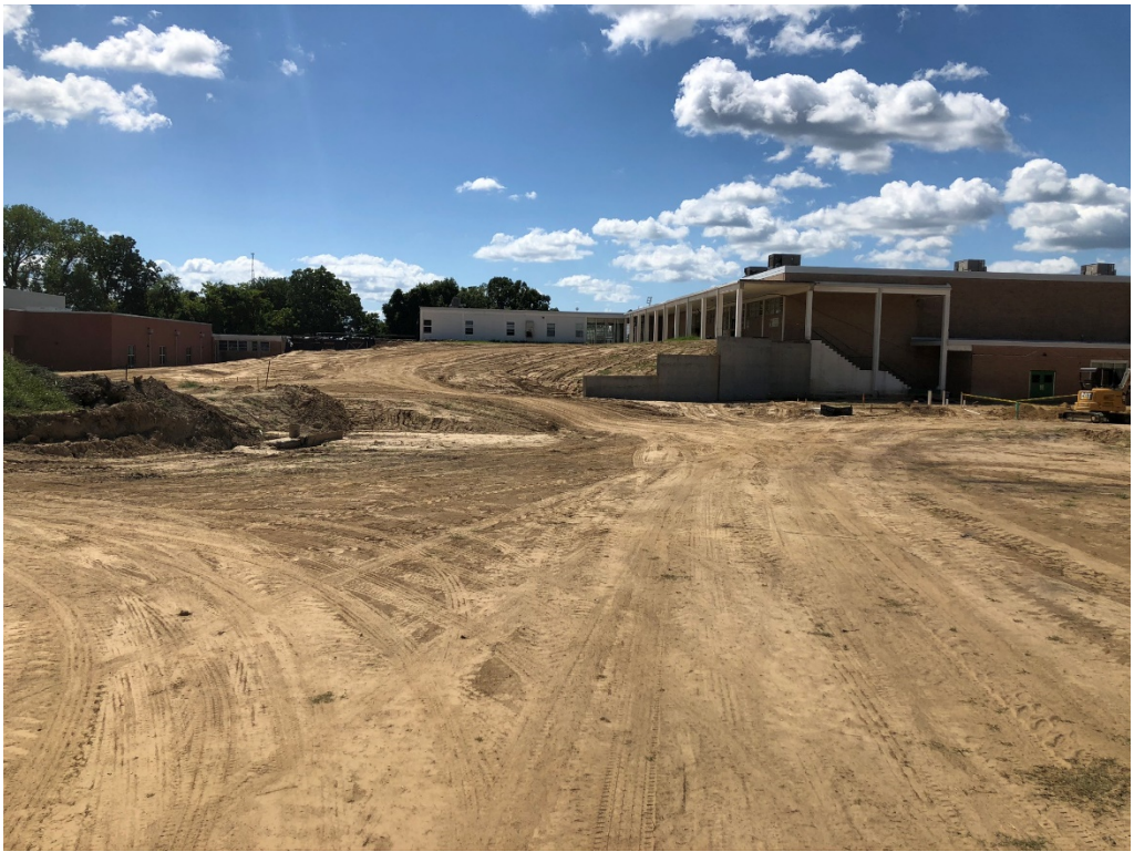
Figure 1 – Site from Job Site Trailer
