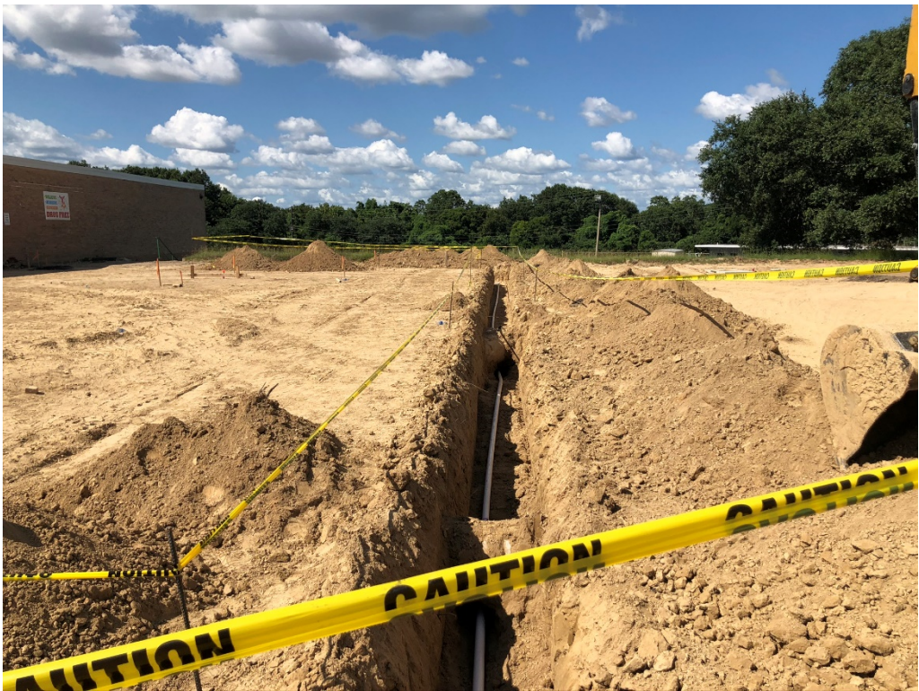
Figure 22 –Pipe Installed
