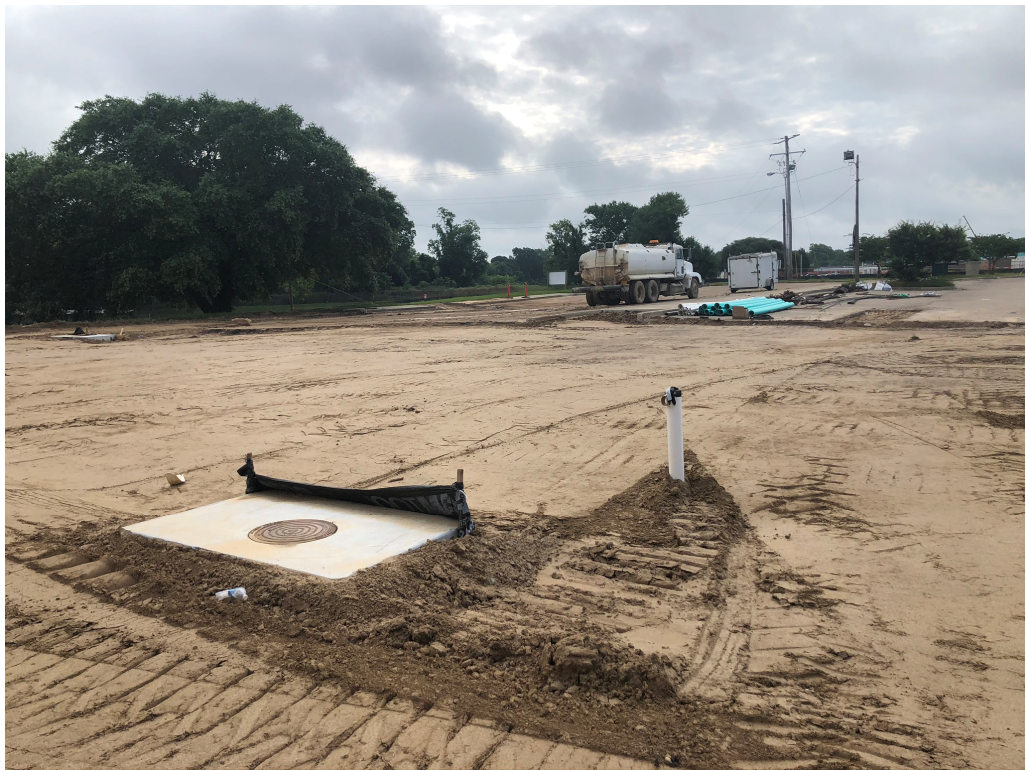
Figure 8 – Compacted Earth at New Addition
