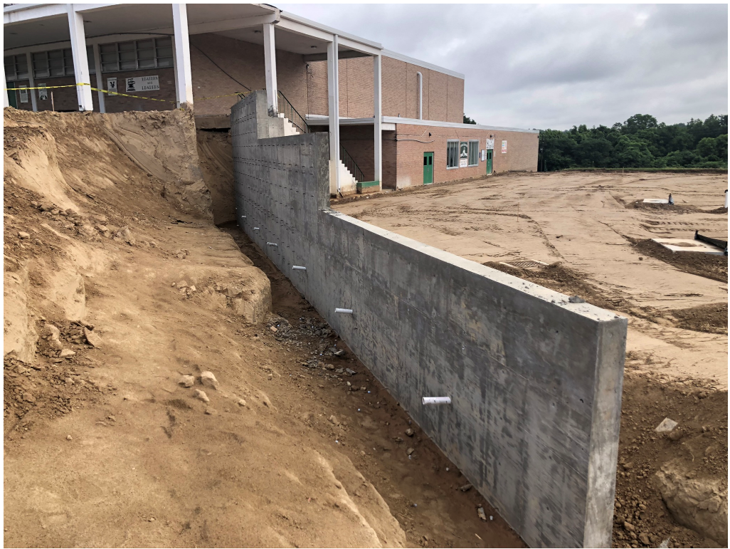
Figure 5 – Foundation Retaining wall Uncovered
