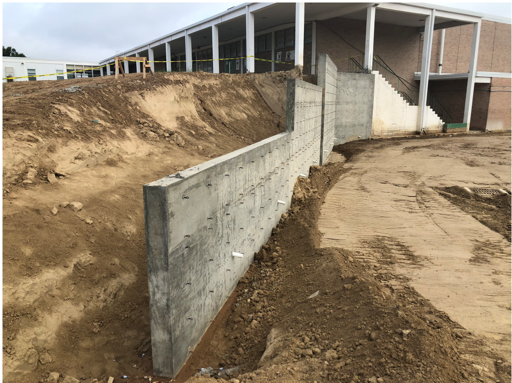
Figure 4 – Foundation Retaining wall Uncovered
