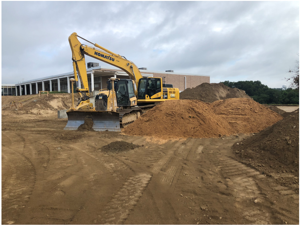
Figure 3 – Select Fill On Site; Dirt Work is Ongoing
