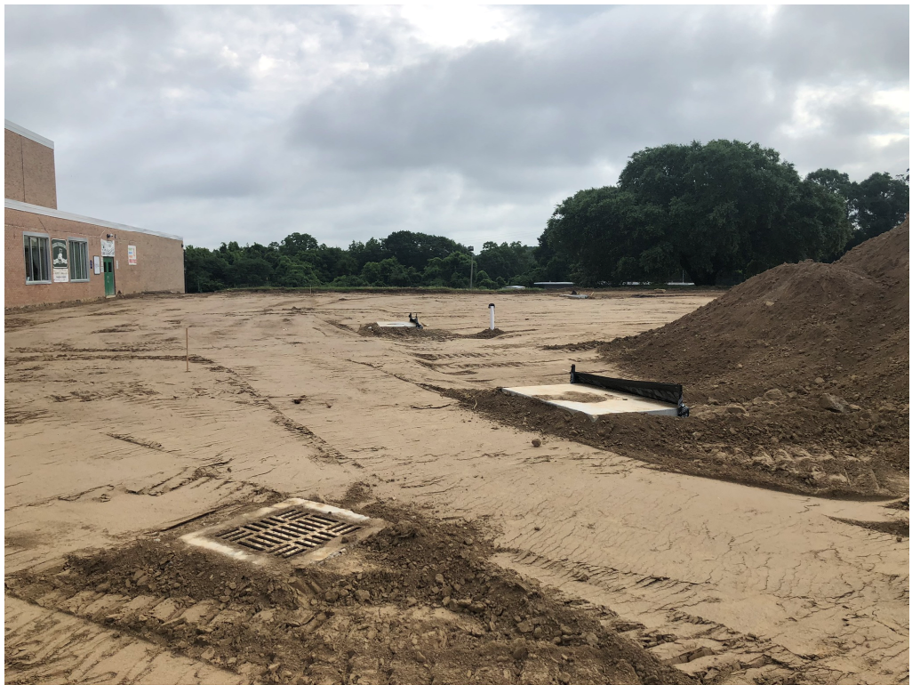
Figure 6 – Compacted Earth at New Addition
