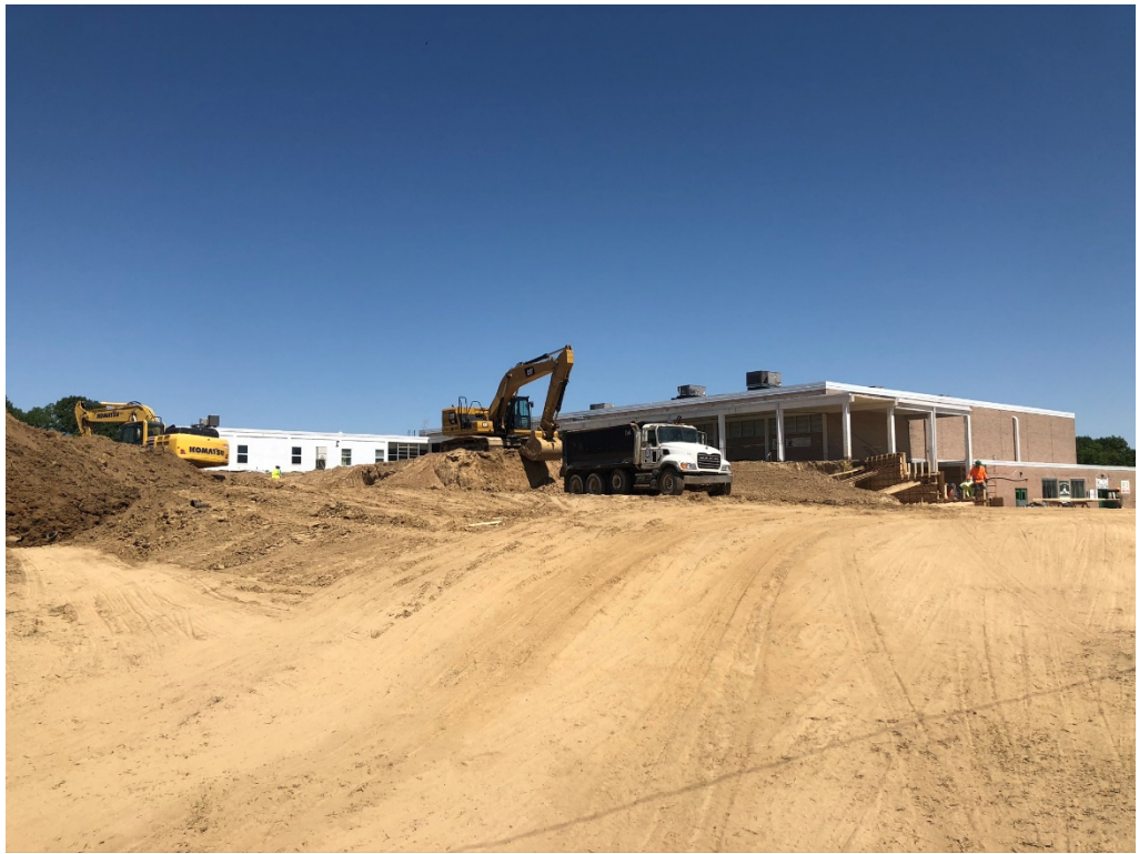
Figure 1 – Continued Dirt Work
