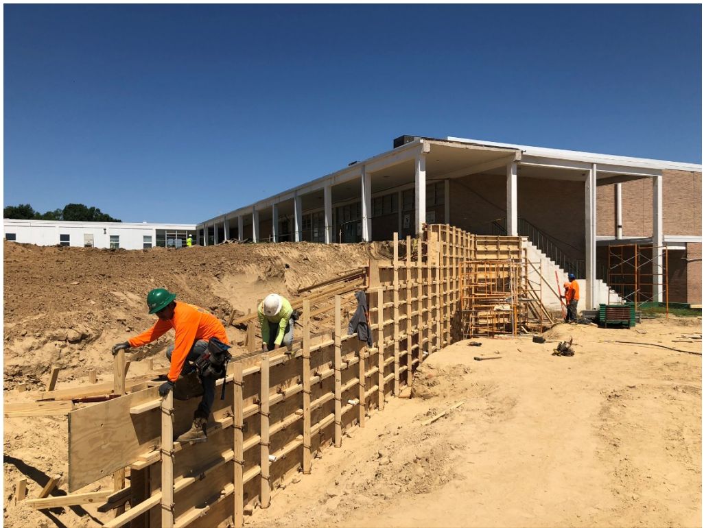
Figure 2 – Retaining Wall Formwork
