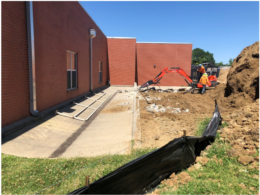
Figure 3 – Demo on Concrete Wall
