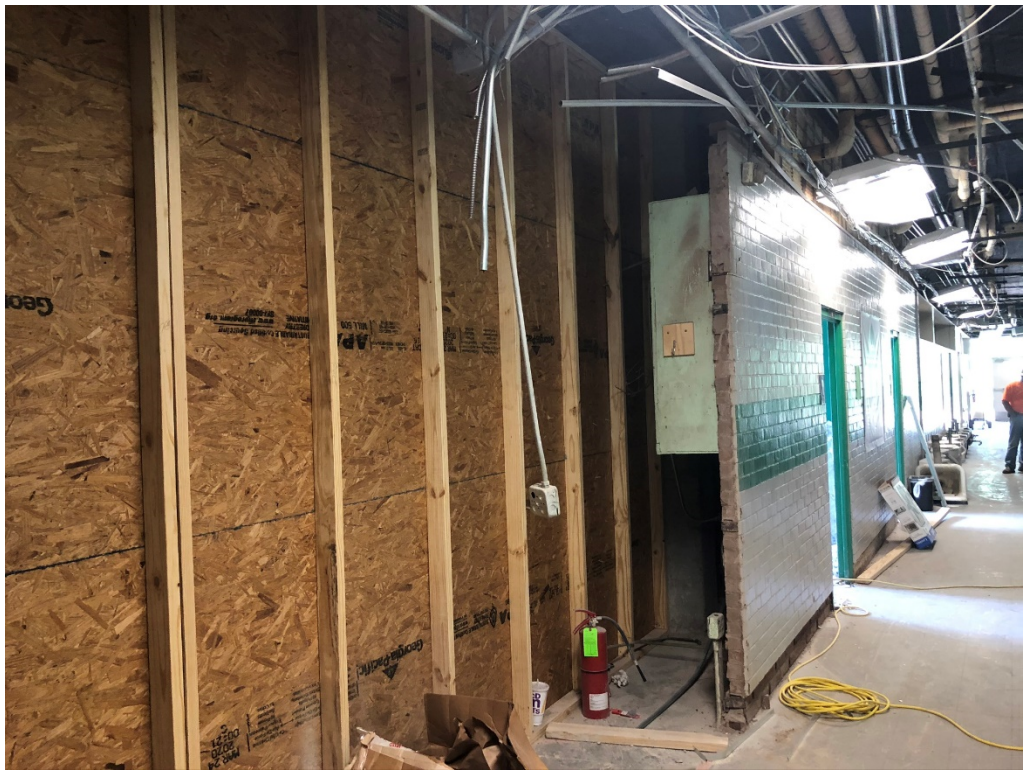
Figure 8 – Temp Wall @ West Hall
