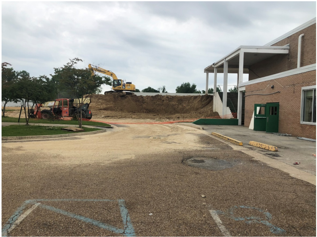
Figure 1 – Continued Dirt Work
