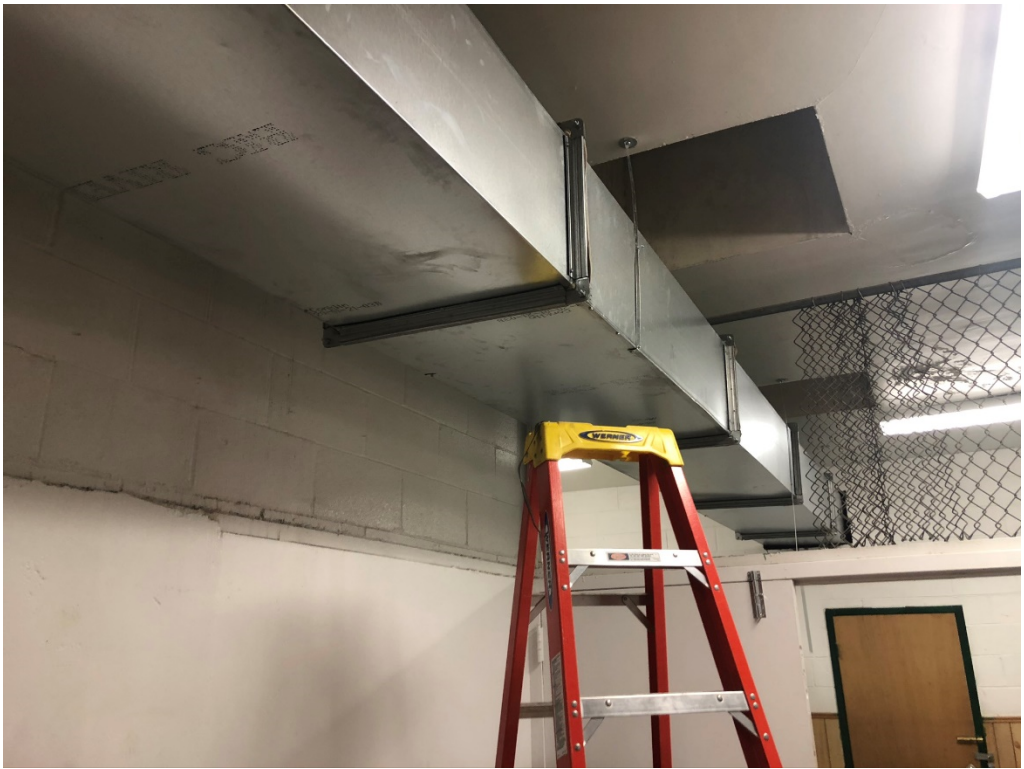
Figure 3 – Duct runs installed
