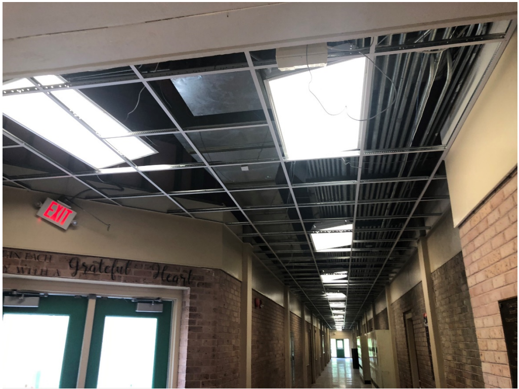
Figure 5 – Ceiling Grid Installed at lower floor Hall
