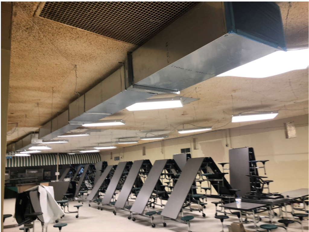
Figure 4 – Duct runs installed
