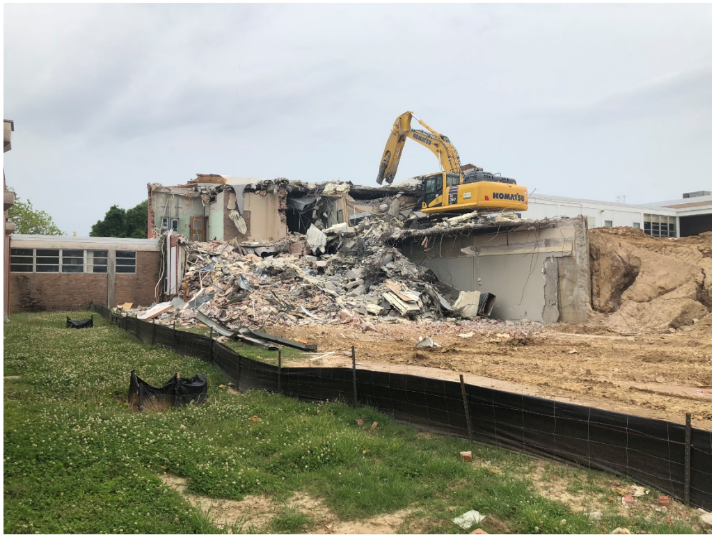
Figure 7 – Demo of Structure Ongoing
