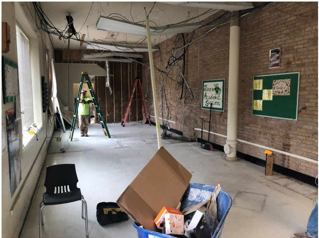
Figure 2 – Entry Office area Demo Ongoing
