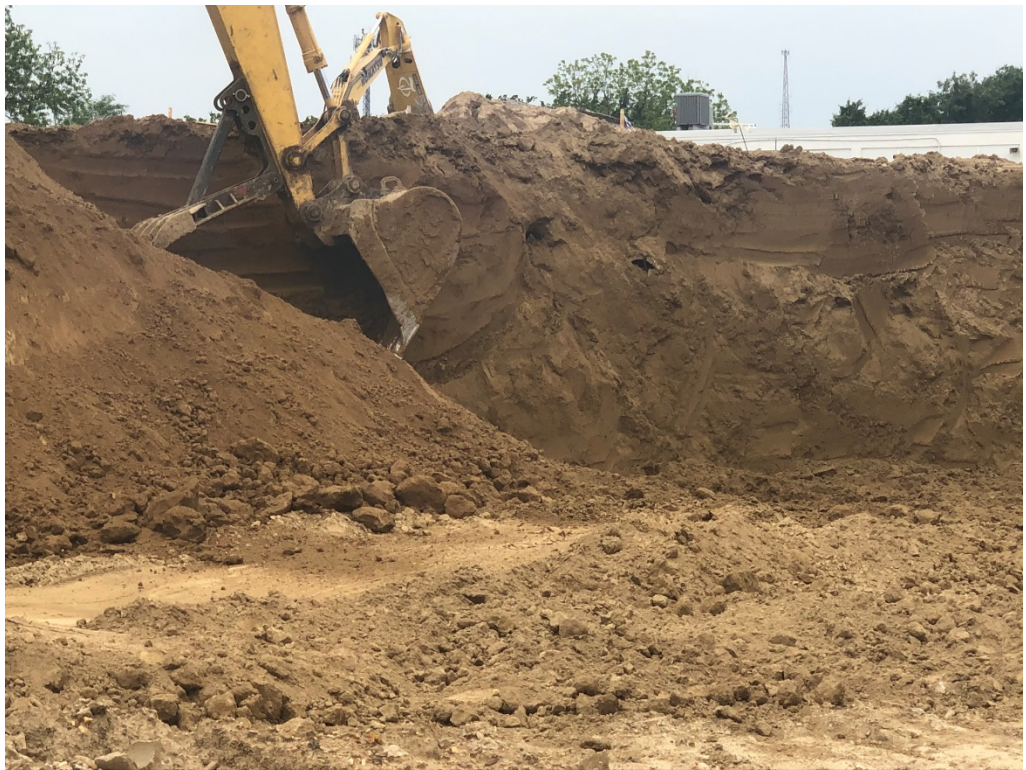
Figure 10 –Dirt Excavation for New Retaining Wall
