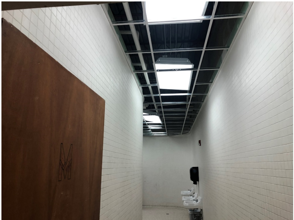
Figure 6 – Ceiling Grid at Lower Floor Bathrooms
