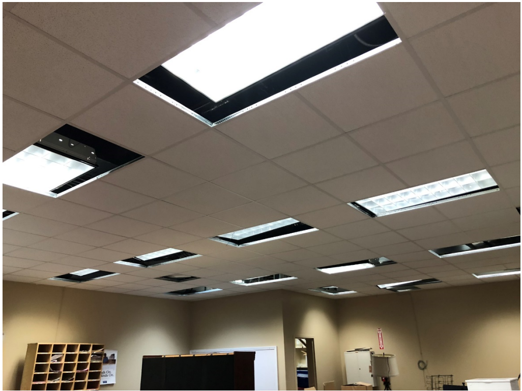
Figure 7 – Lower Level Ceiling Grid and New Tile Work
