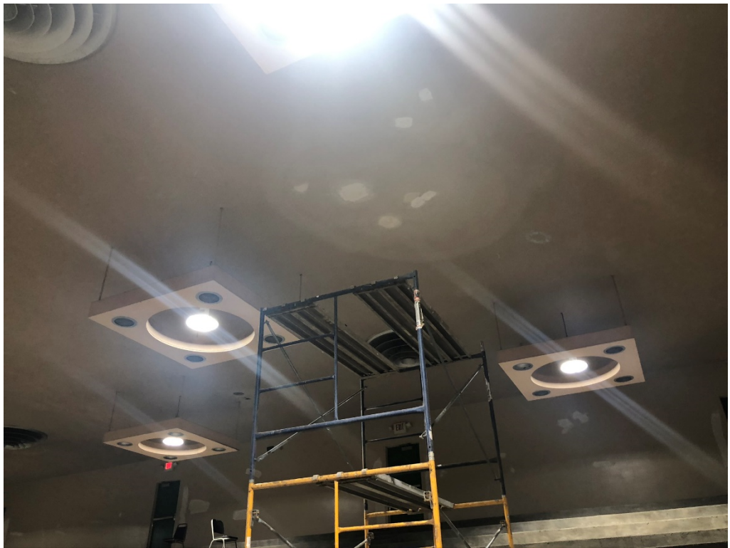
Figure 6 – Plaster patching @ Auditorium
