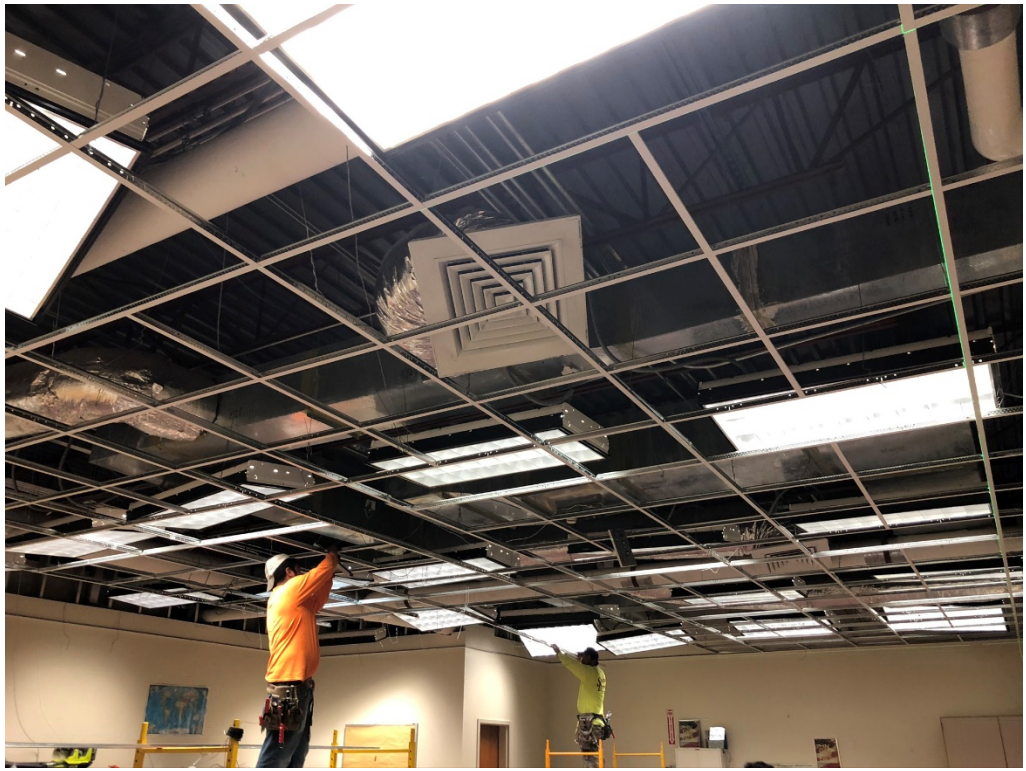
Figure 9 – Lower Level Ceiling Grid and New Tile Work
