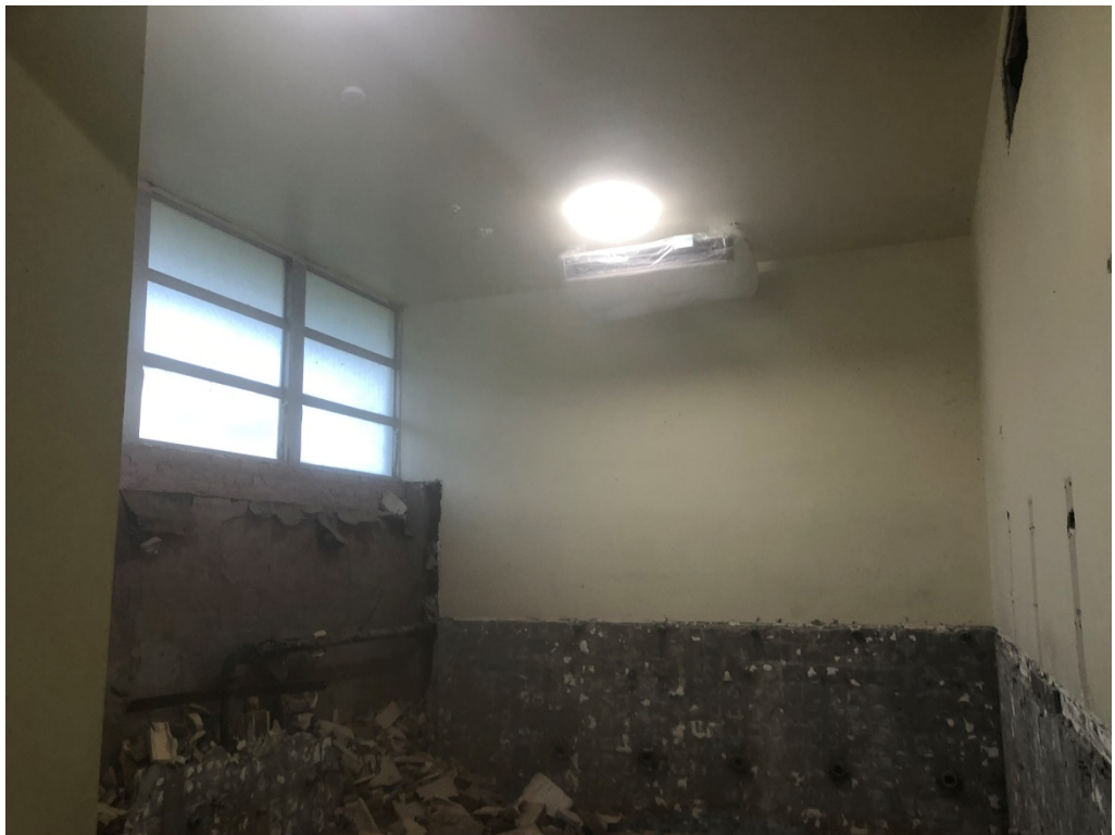
Figure 2 – Windows at Bath Area
