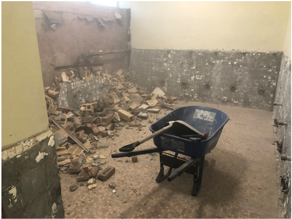
Figure 1 – Bathroom Demo of Chase Wall
