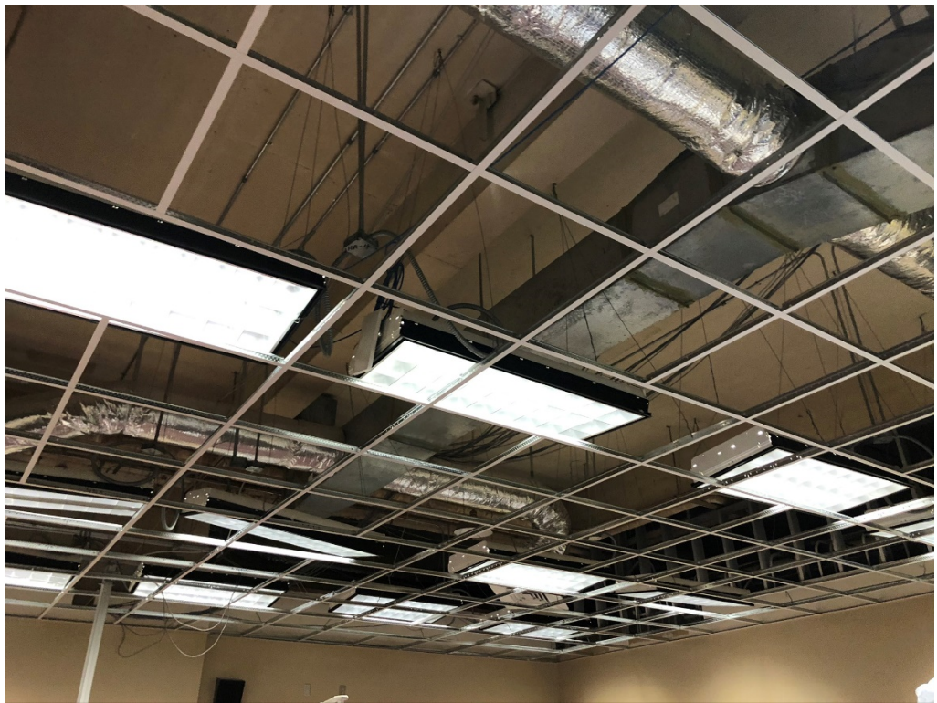
Figure 8 – Lower Level Ceiling Grid and New Tile Work
