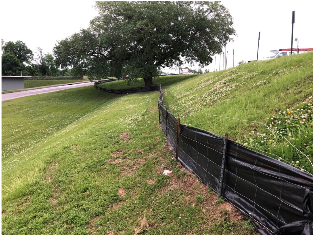
Figure 10 – North Hill Sediment Control In Place
