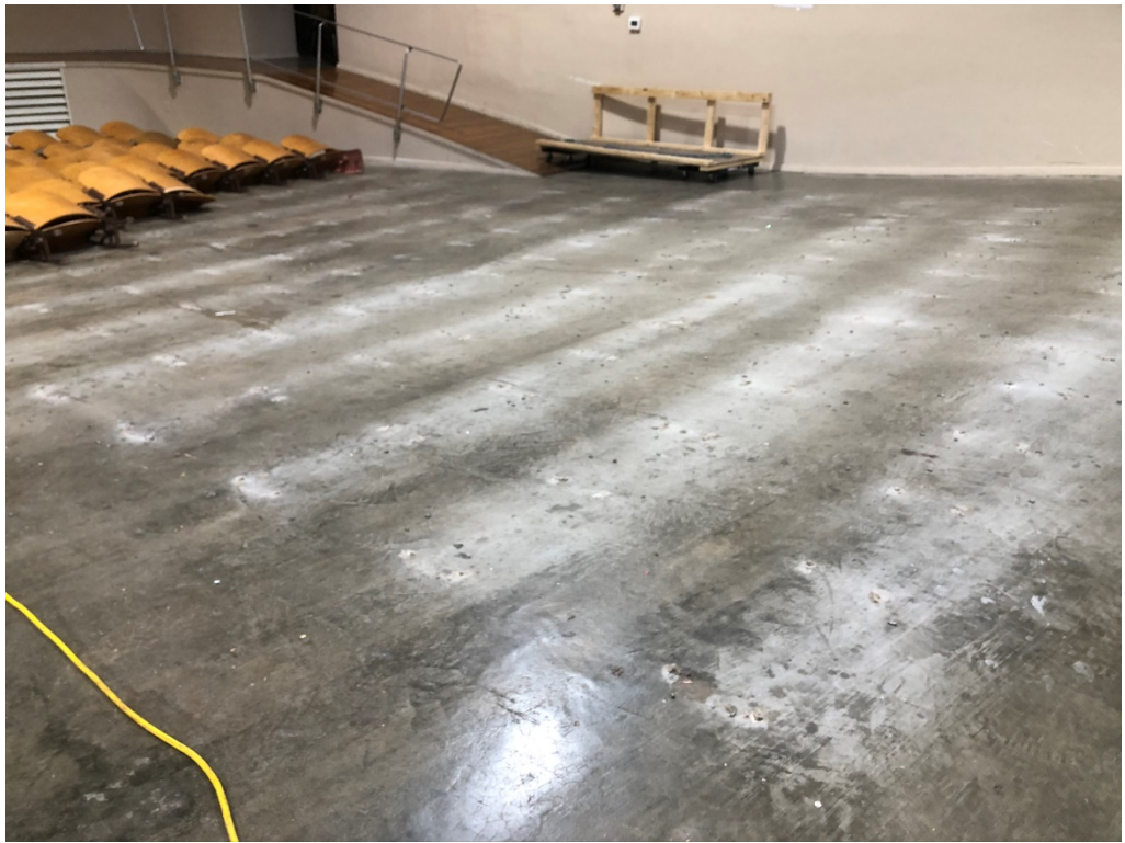
Figure 5 – Seats Removed from auditorium and metal studs ground to floor
