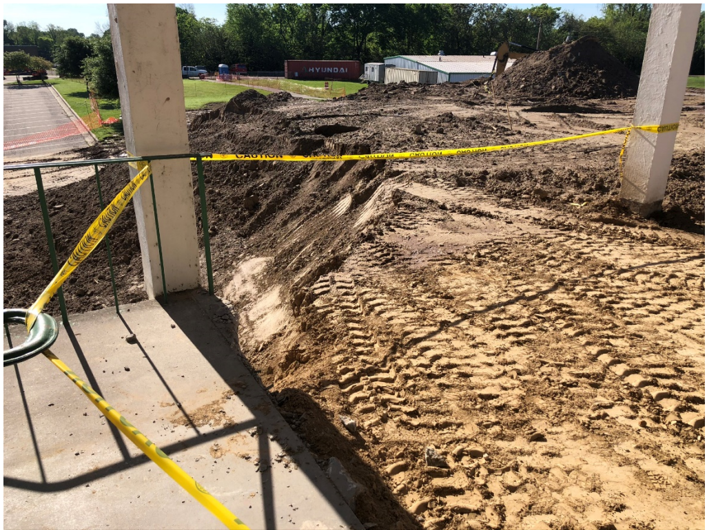
Figure 2 – Retaining Wall Removed
