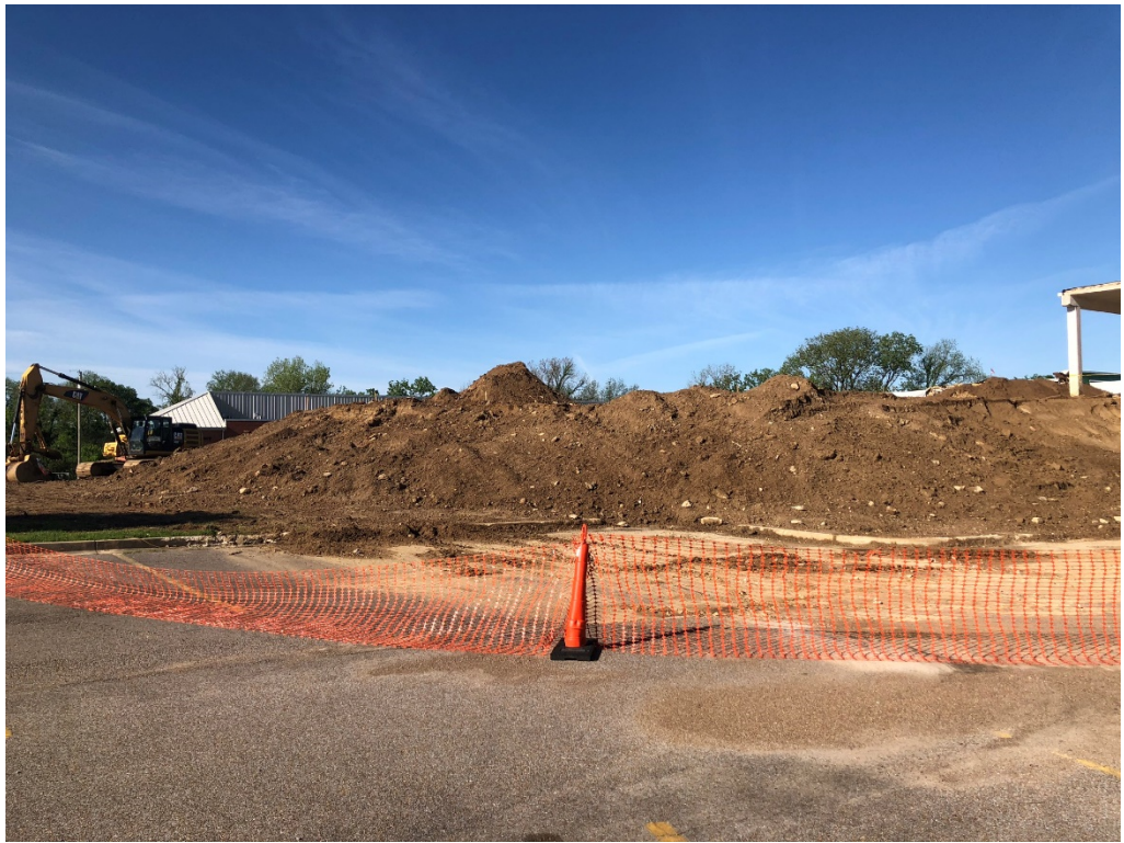
Figure 1 – Retaining Wall Removed
