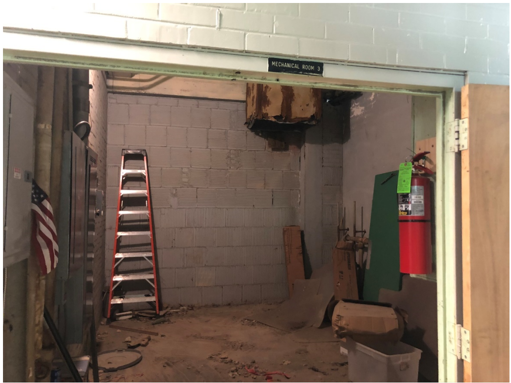
Figure 7 – Mechanical Room Demo
