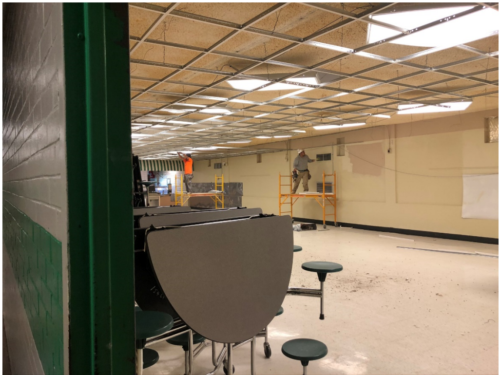
Figure 12 – Ceiling Grid Demo at Cafeteria
