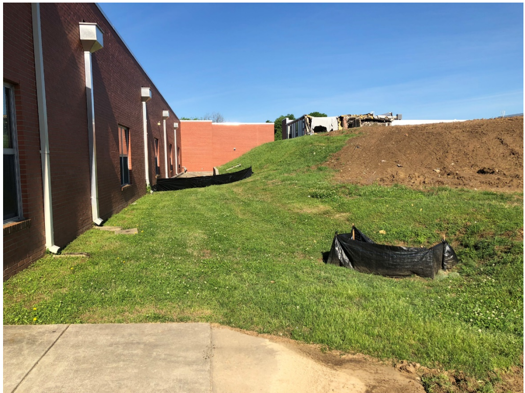
Figure 8 – Silt Fencing Installed
