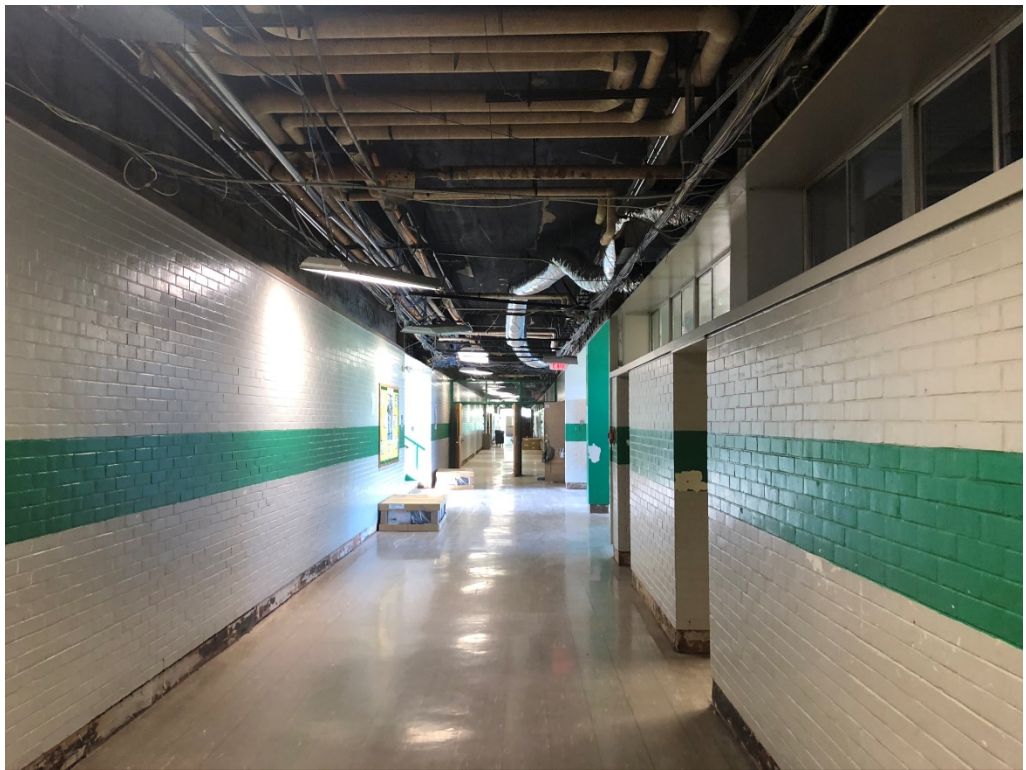
Figure 6 – Ducting Demo at Hallways
