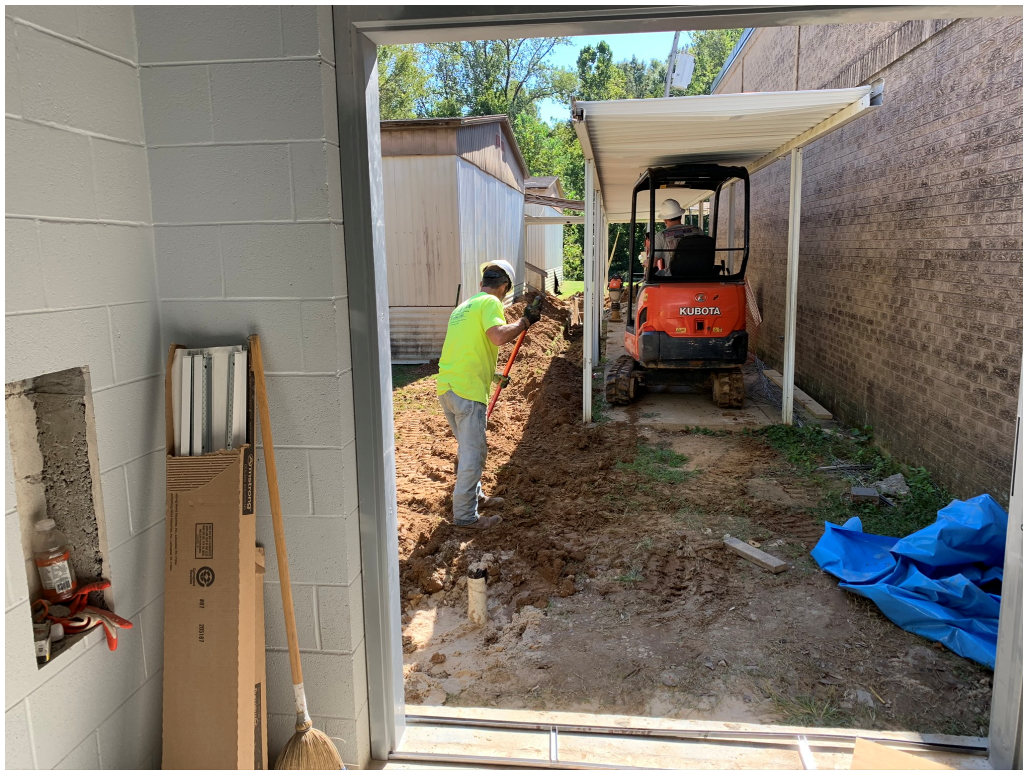
Figure 10 – Sewer Line Install
