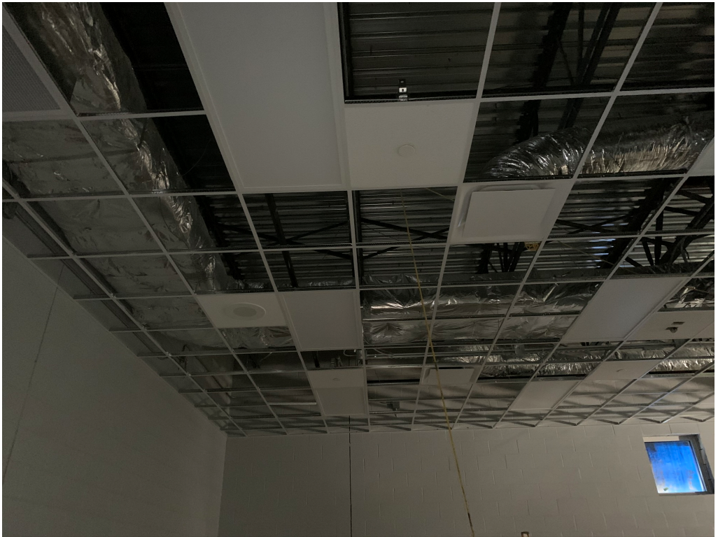
Figure 6 – Ceiling Grid Work
