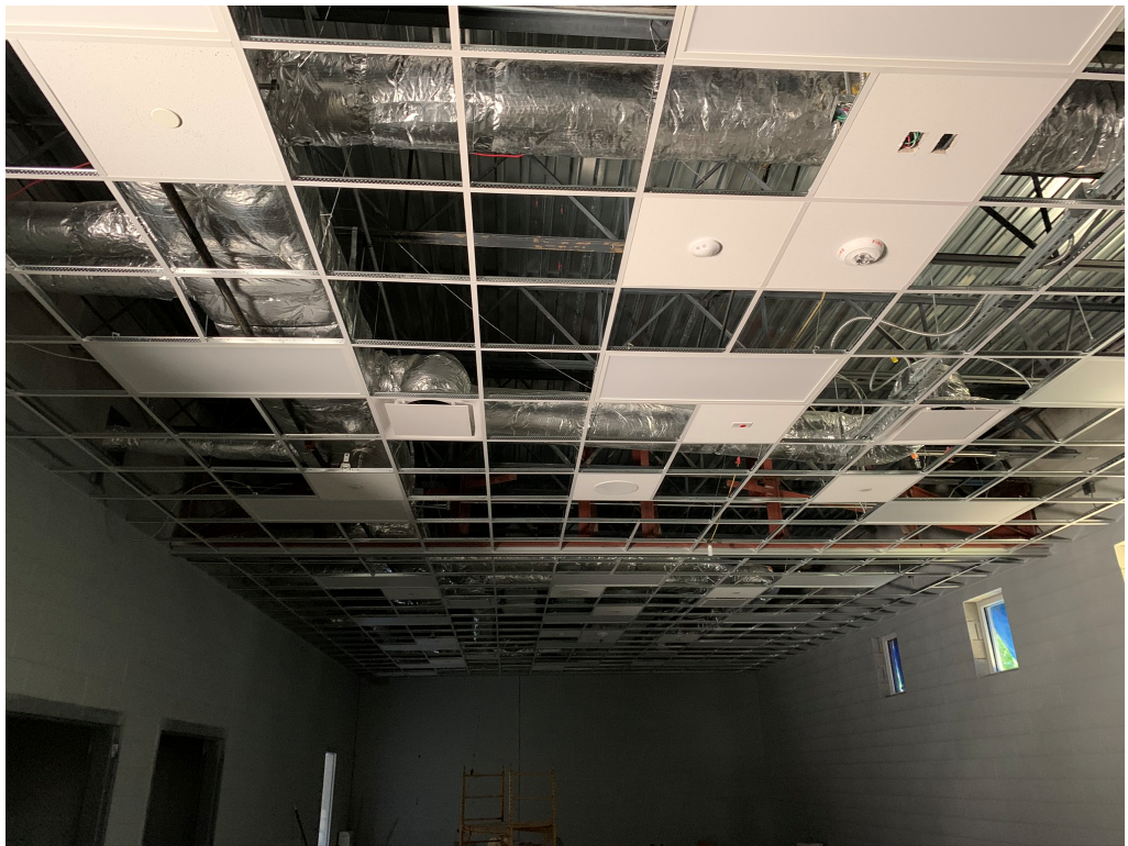
Figure 8 – Ceiling Grid Work
