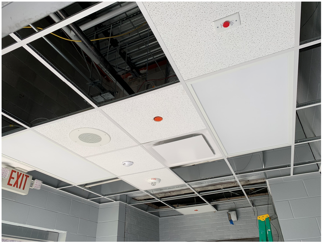
Figure 9 – Ceiling Grid Work
