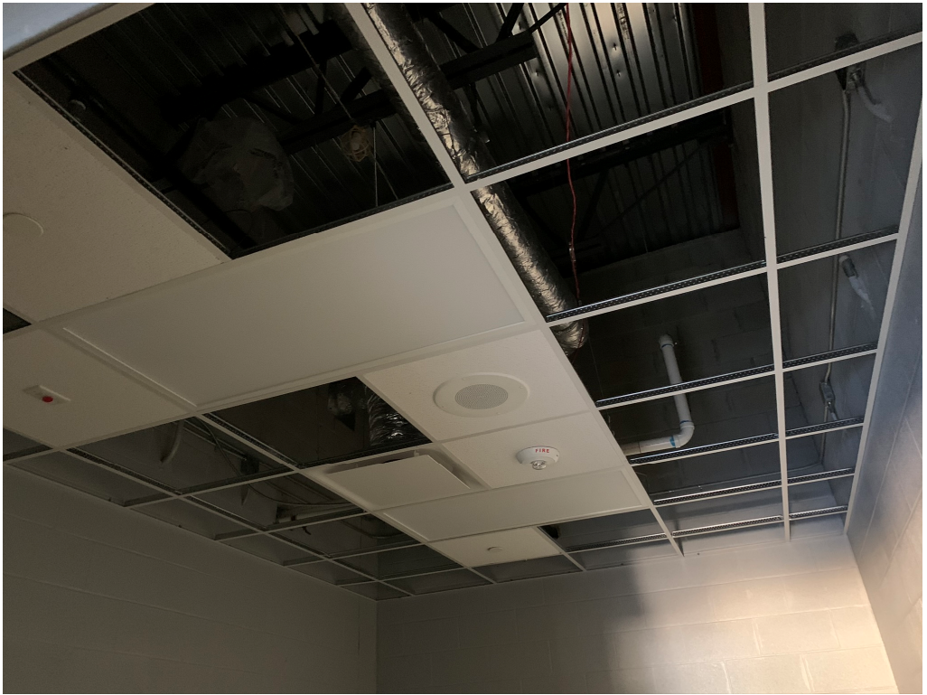
Figure 5 – Ceiling Grid Work
