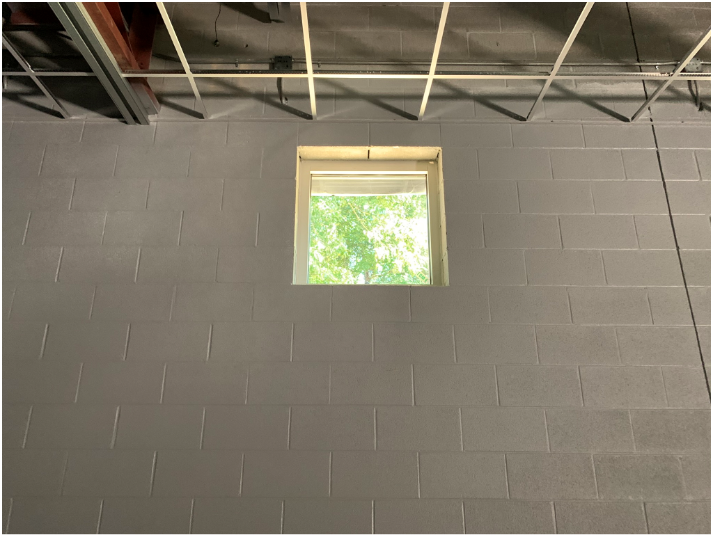
Figure 11 – Windows Installed at CMU Wall
