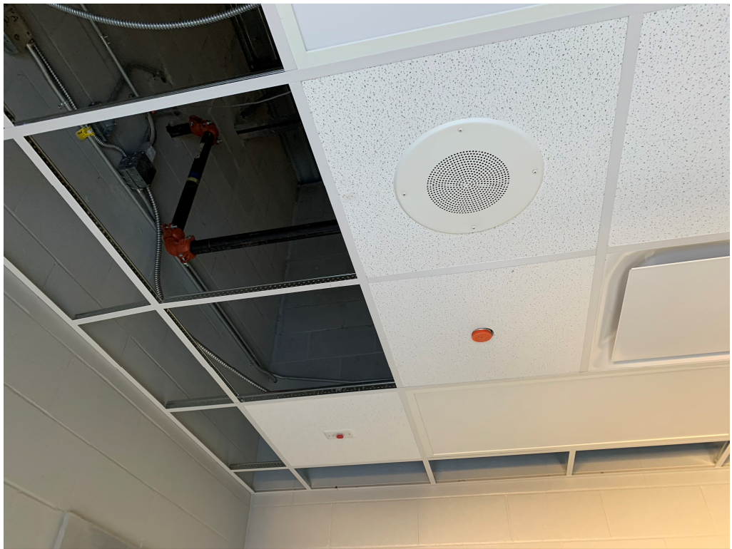
Figure 4 – Ceiling Grid Work
