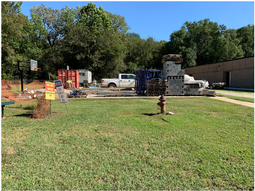
Figure 1 – Lay Down Area
