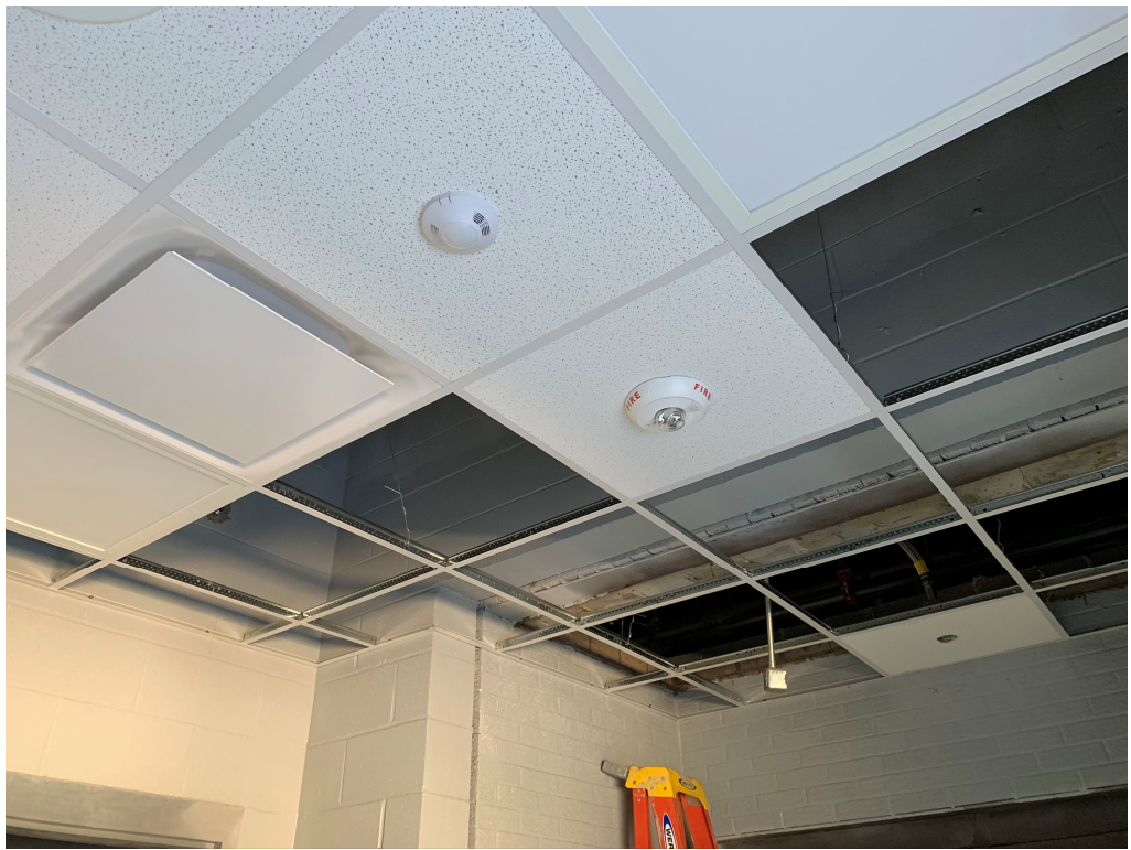
Figure 3 – Ceiling Grid Work
