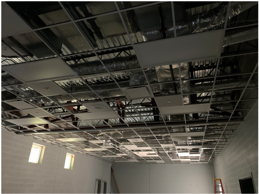
Figure 7 – Ceiling Grid Work
