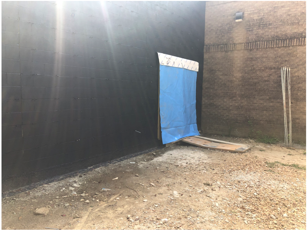
Figure 1 – Coverings Installed at Openings
