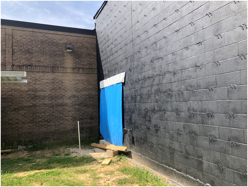
Figure 3 – Coverings Installed at Openings
