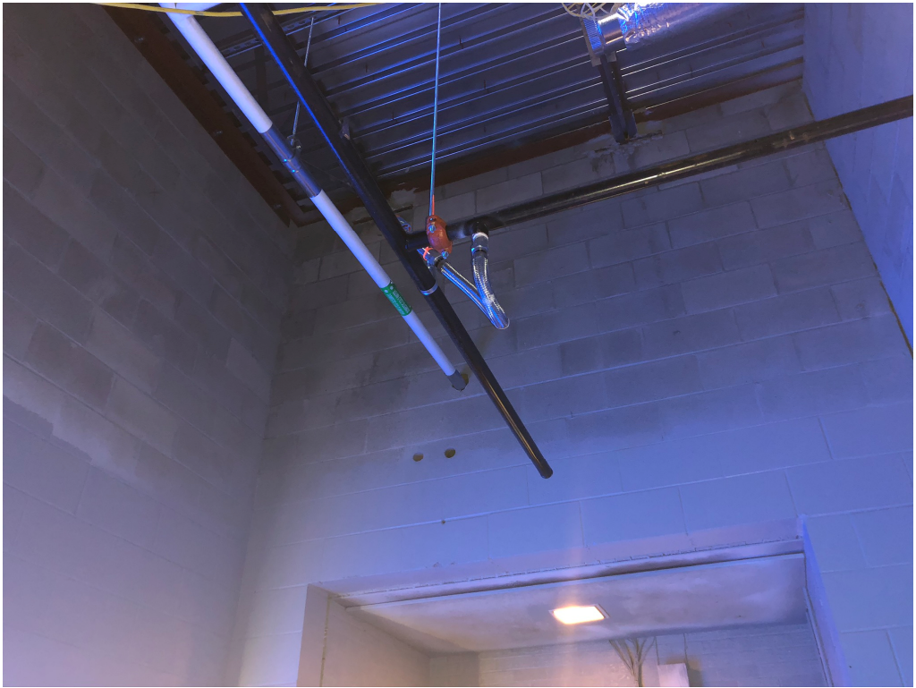
Figure 5 – Sprinkler Pipes Installed
