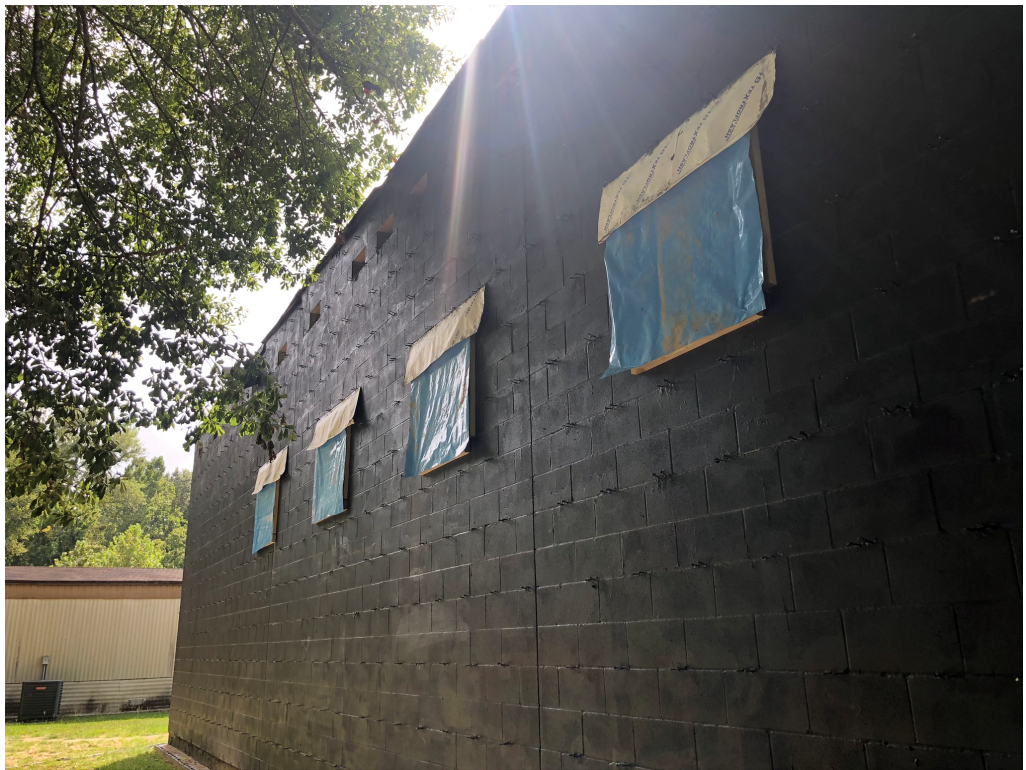
Figure 2 – Coverings Installed at Openings
