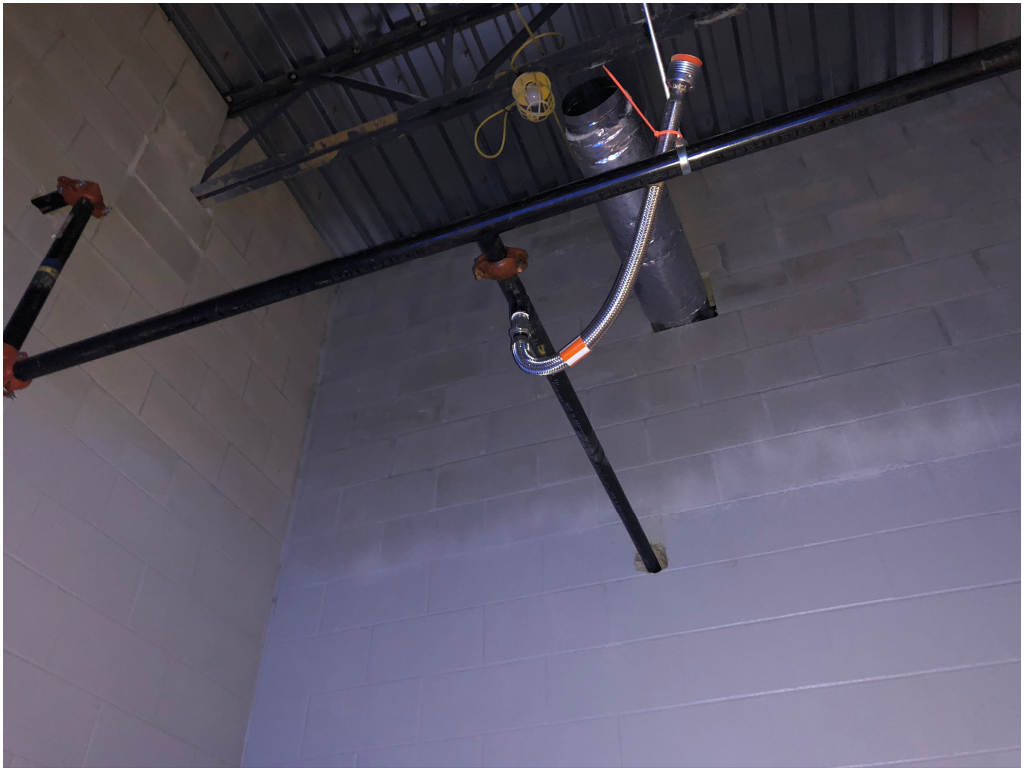
Figure 4 – Sprinkler Pipes Installed
