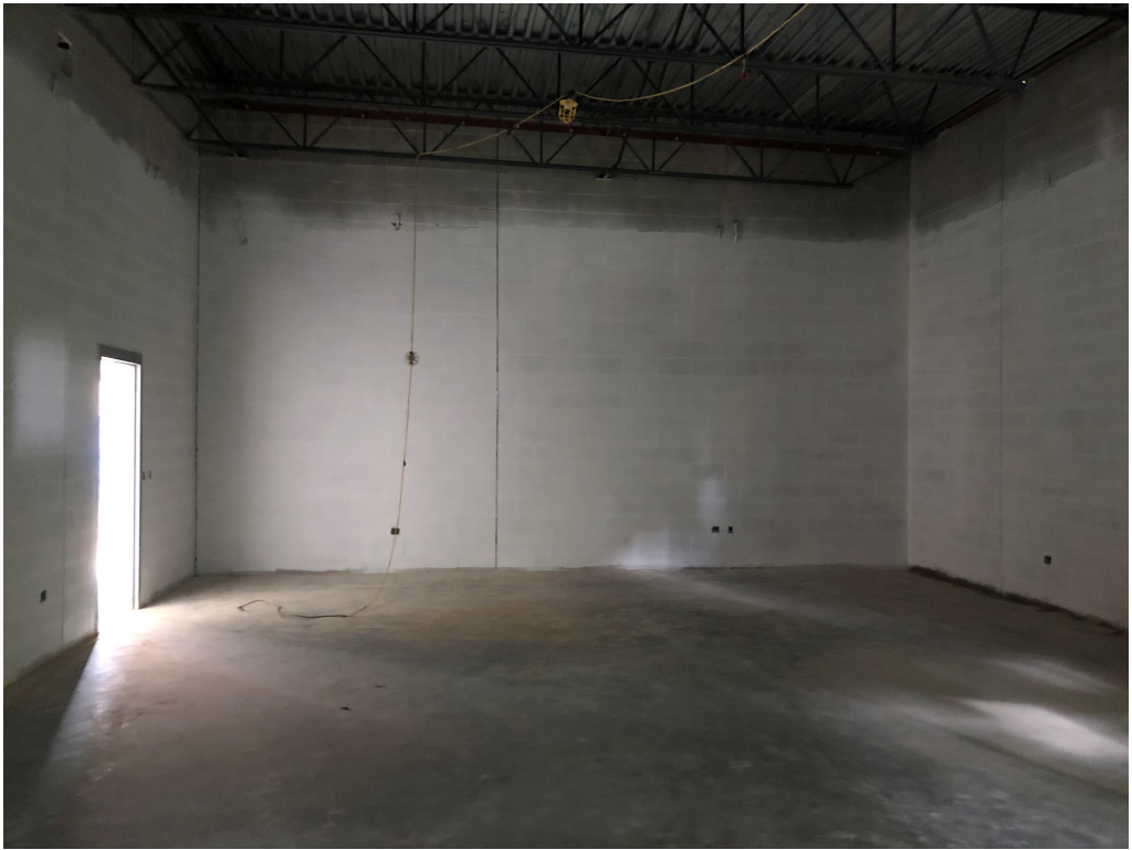
Figure 7 – Prime Coat at Addition
