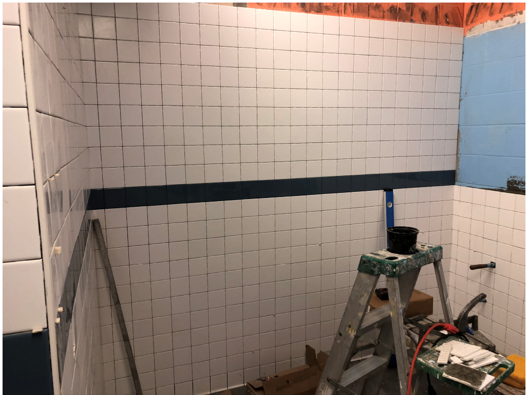
Figure 4 – Tile Reinstallation
