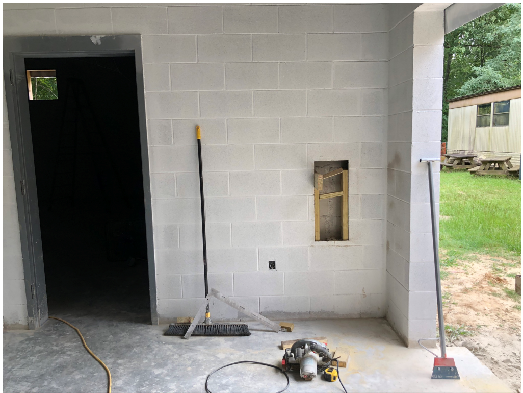
Figure 6 – Prime Coat at Addition
