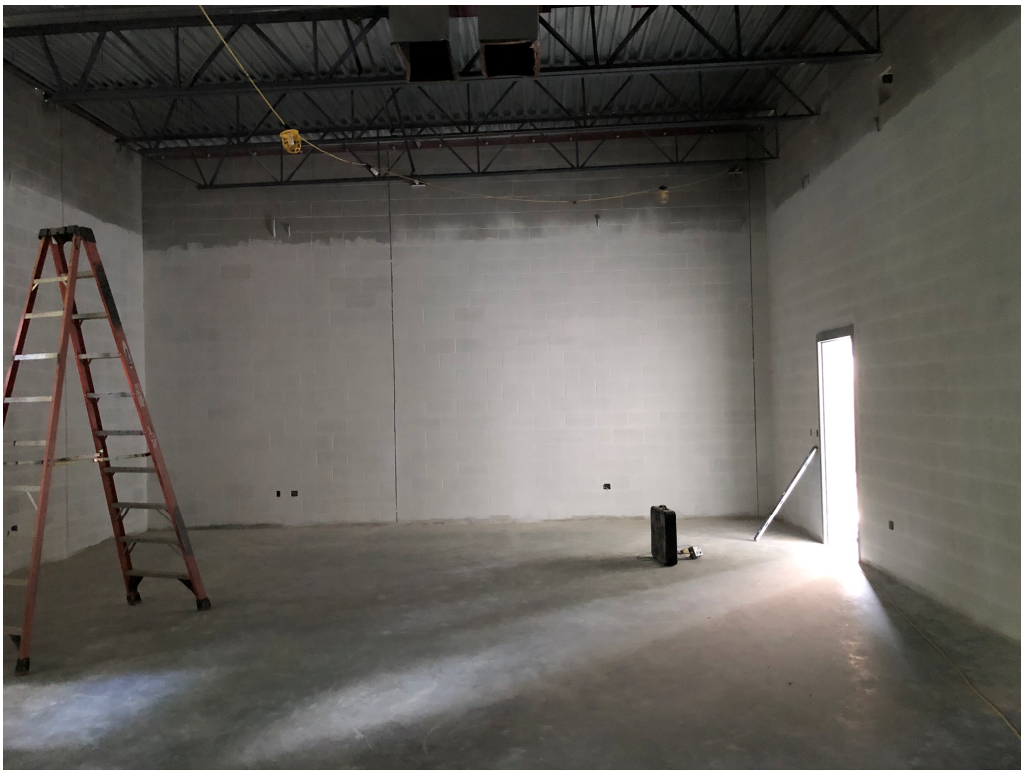
Figure 8 – Prime Coat at Addition
