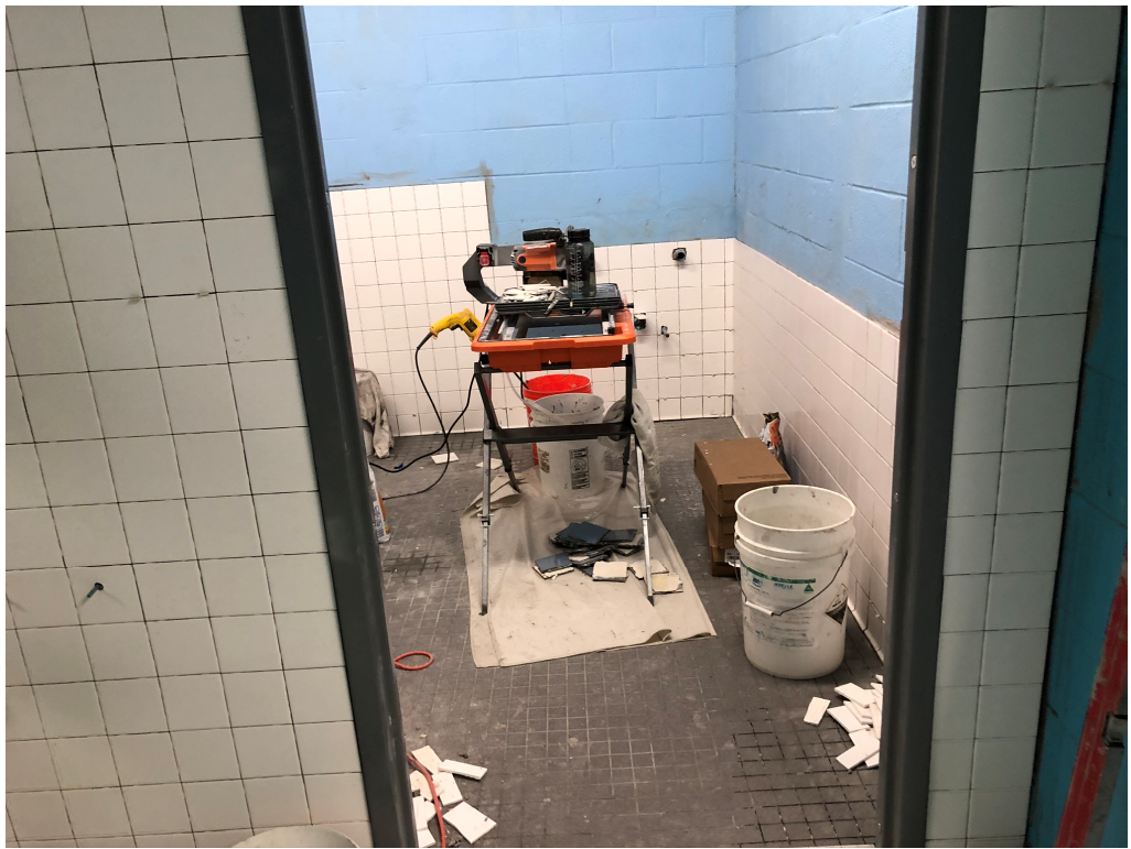
Figure 3 – Tile Reinstallation
