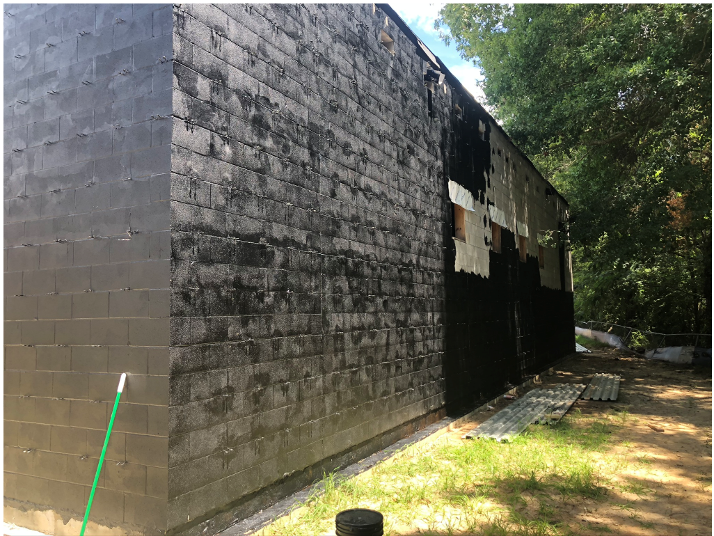
Figure 6 – Damp-proofing at CMU
