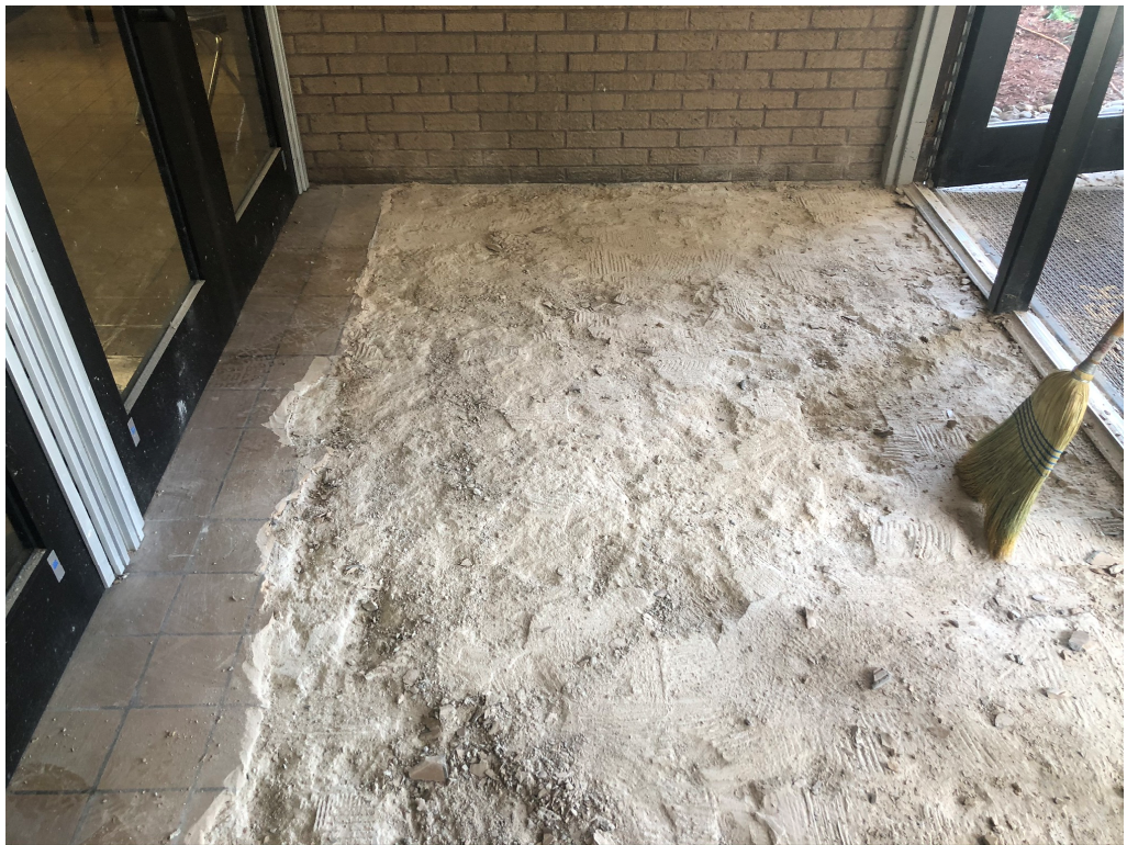
Figure 2 – Demoed Floor Tile
