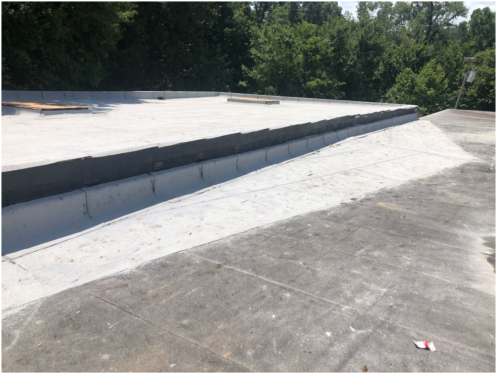
Figure 7 – Roofing at Cricket and New Roof
