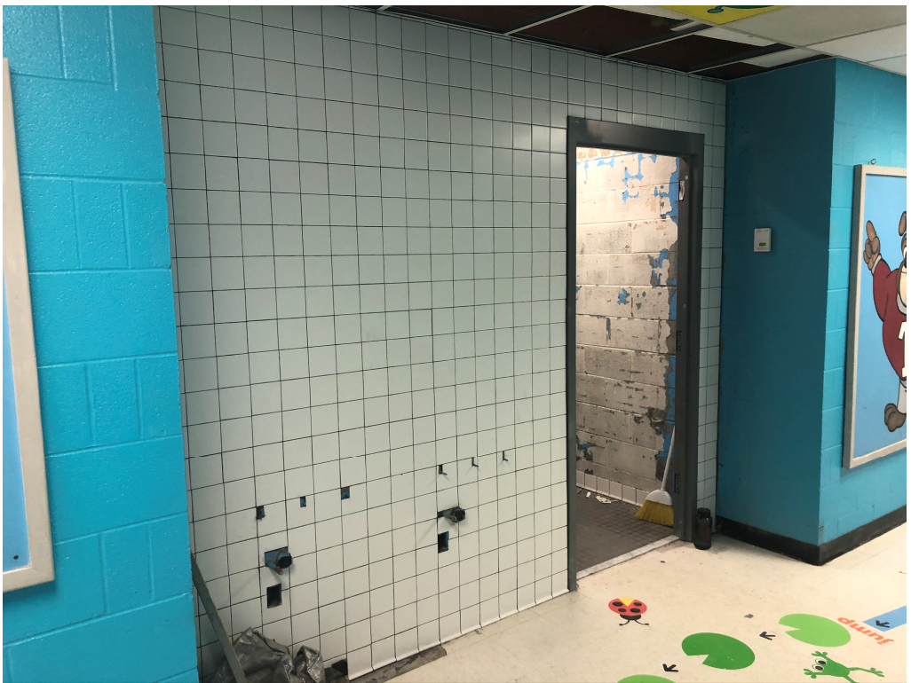
Figure 4 – Tile Installed at Wall
