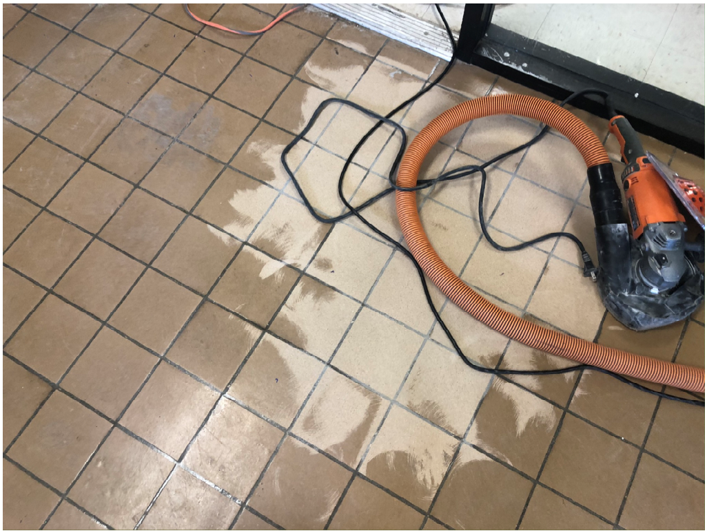
Figure 3 – Tile Grinding for Prep
