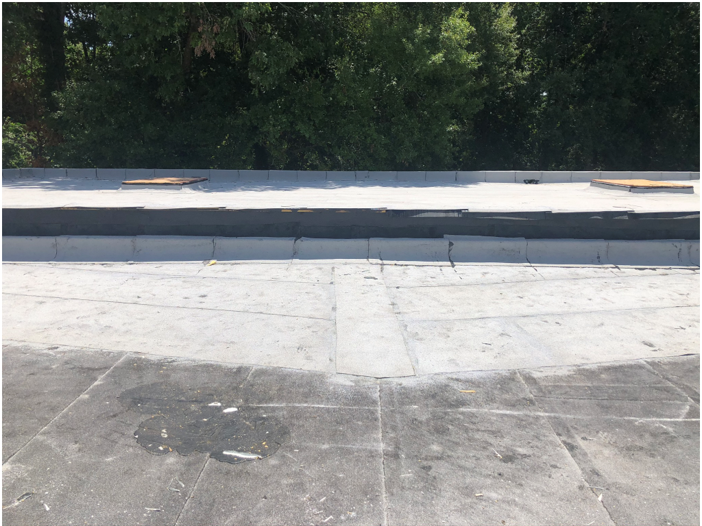
Figure 8 – Roofing at Cricket and New Roof
