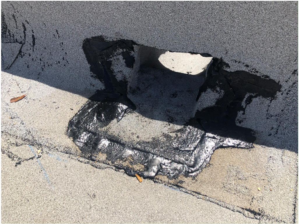
Figure 11 – Roof Drainage Outlet
