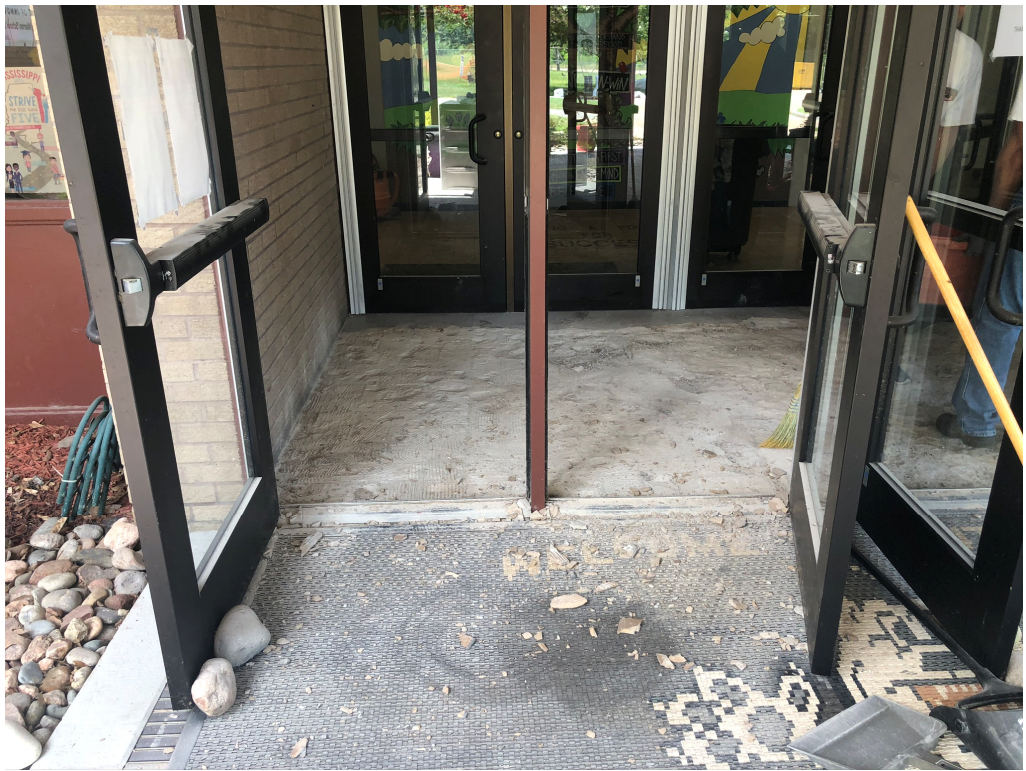
Figure 1 – Demoed Floor Tile
