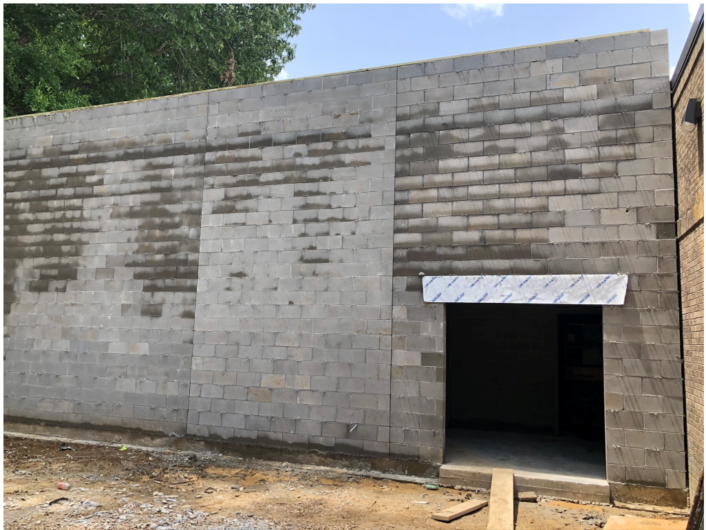
Figure 8 – Exterior Wall Closed in and Treated Parapet Board Installed
