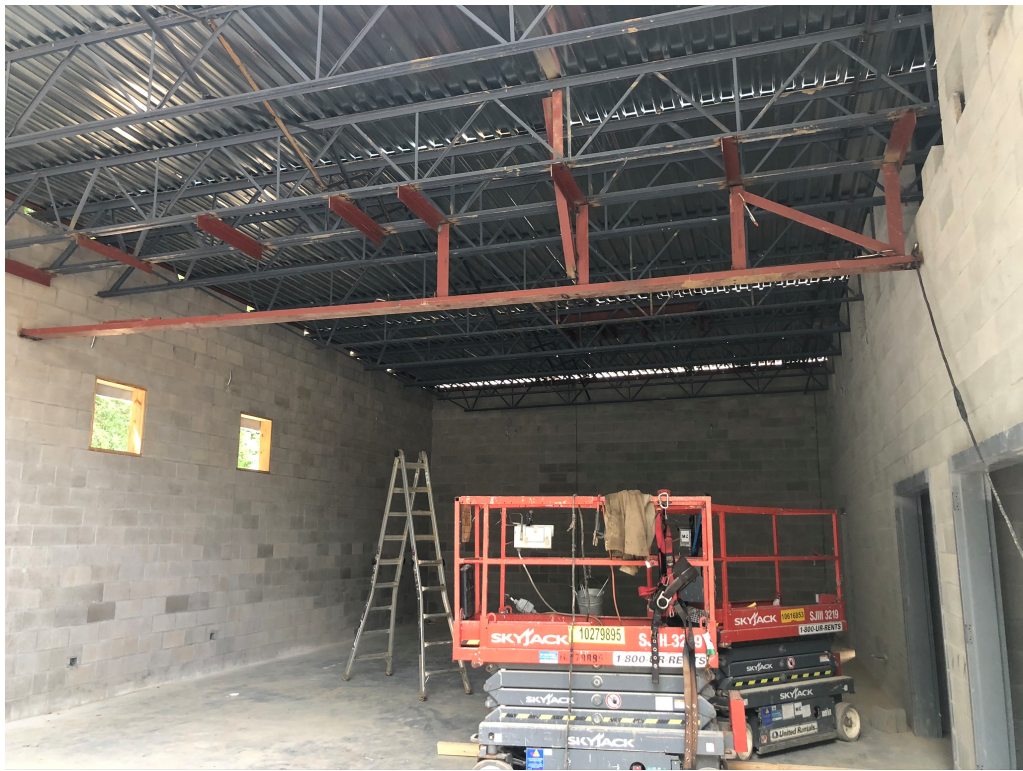
Figure 5 – Structural Steel Installation
