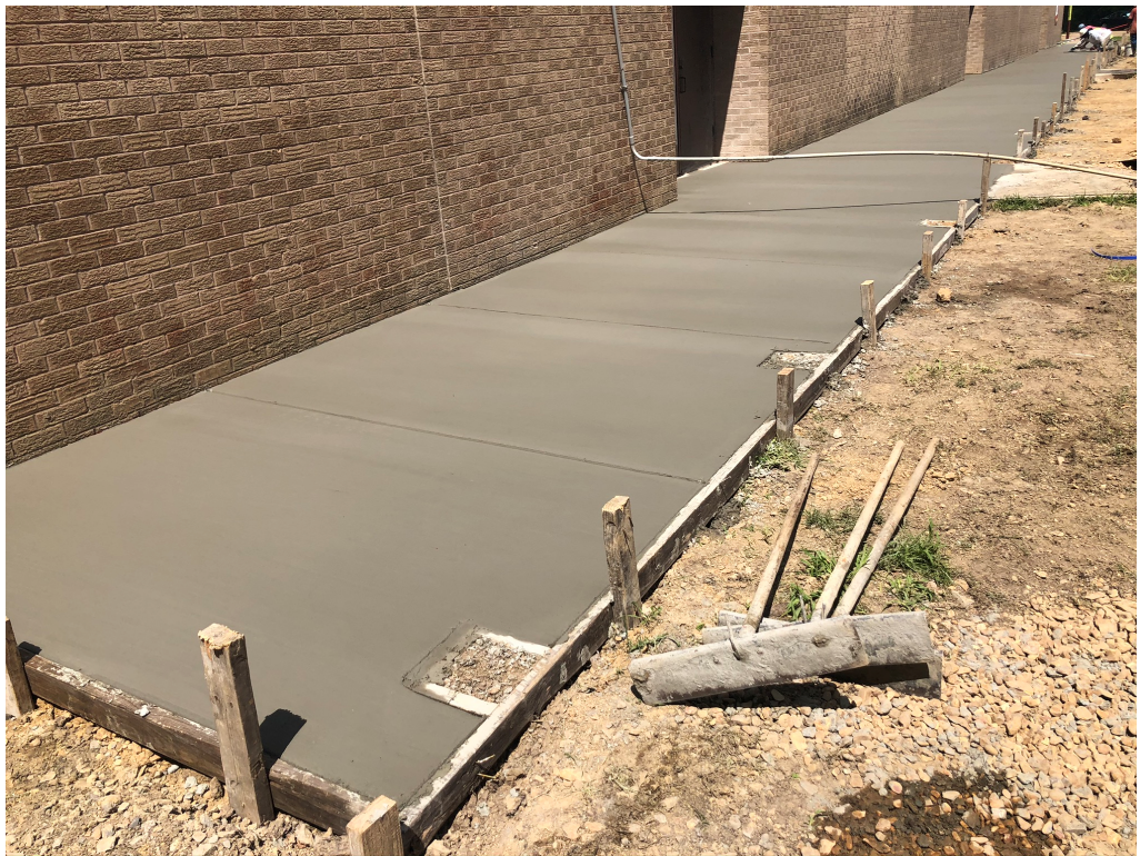
Figure 2 – Sidewalk in Curing Stage
