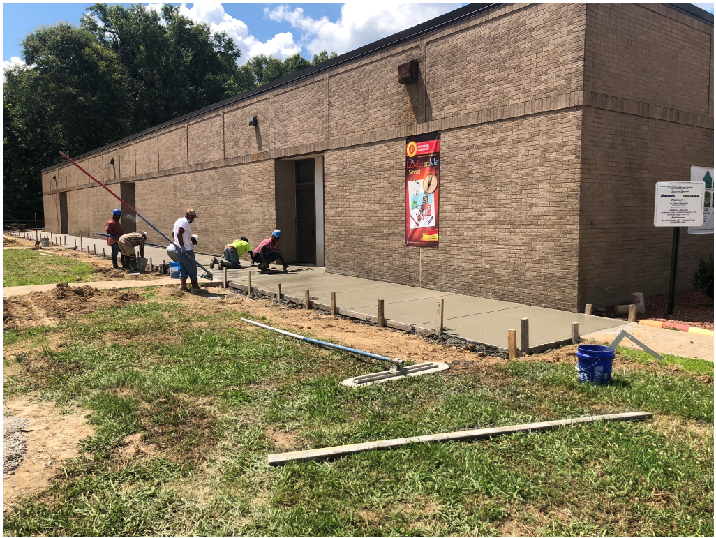
Figure 1 – Concrete Finishers at Work
