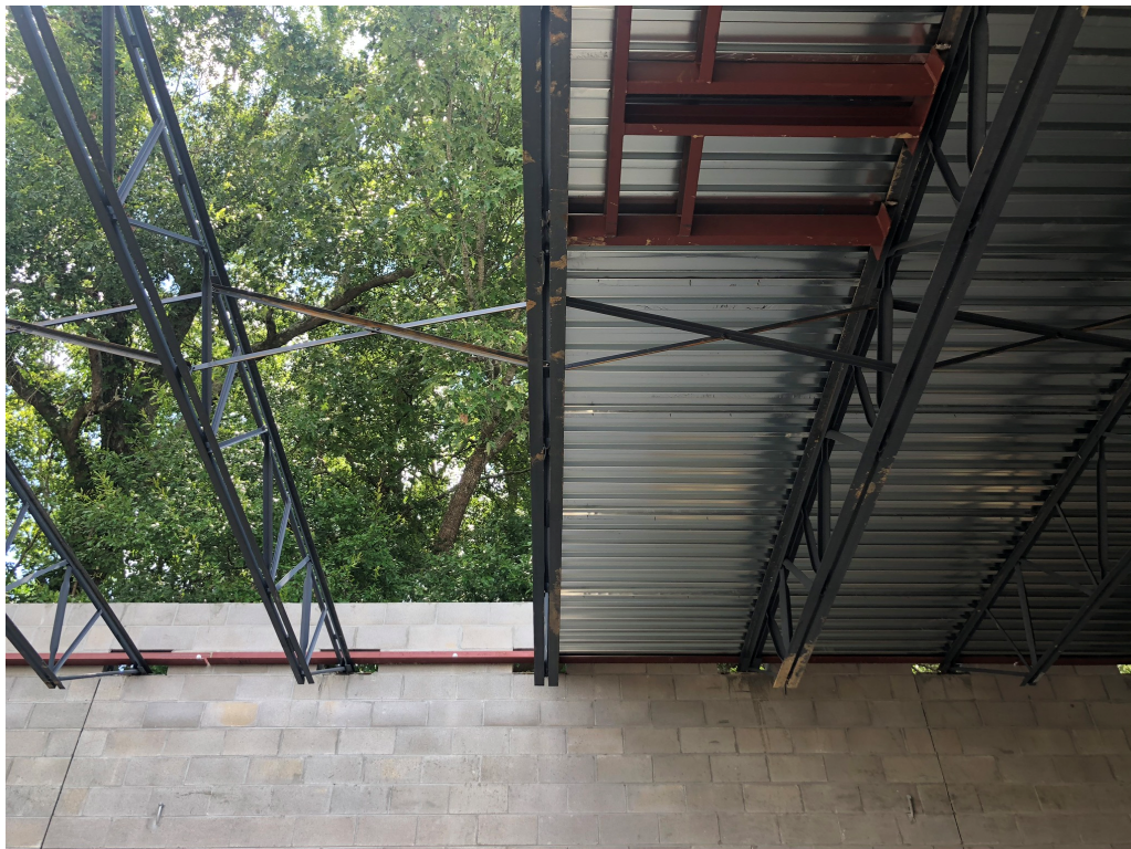
Figure 6 – Deck Installation is Ongoing
