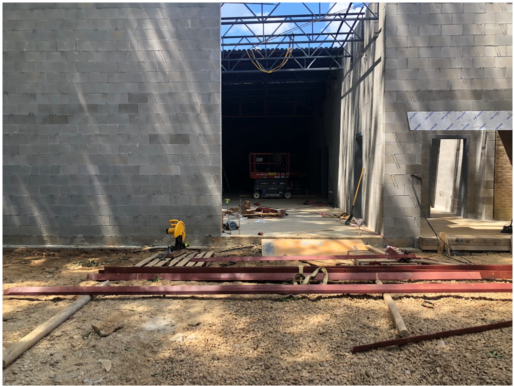
Figure 3 – Structural Steel Fabrication
