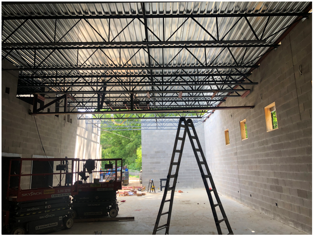
Figure 7 – Ongoing Work From Band Room
