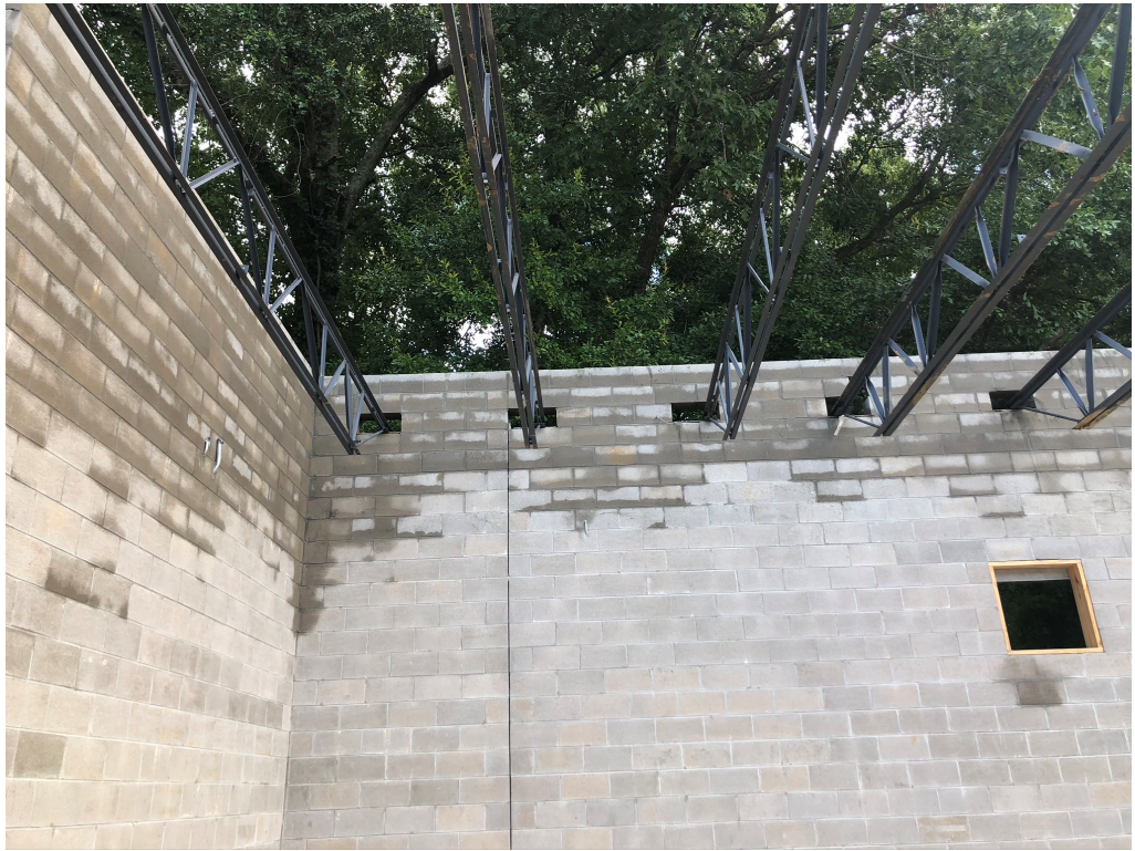
Figure 3 – Truss Installation
