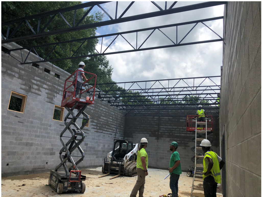
Figure 4 – Truss Installation
