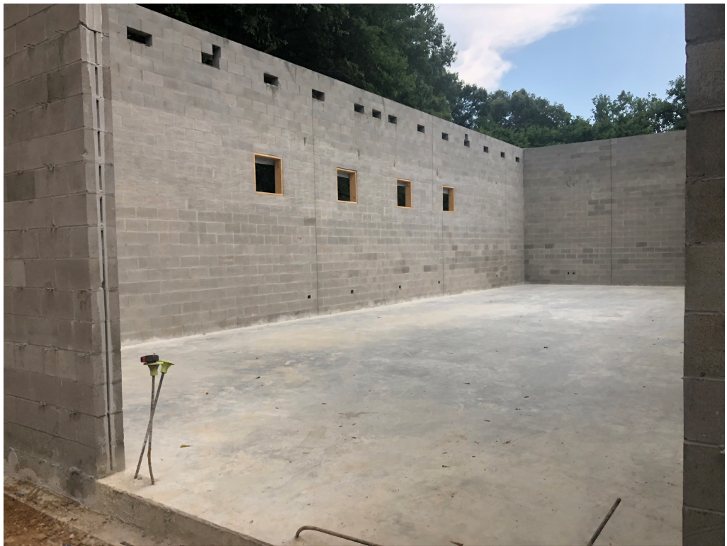
Figure 2 – CMU Block Rubbed and Free of Debris
