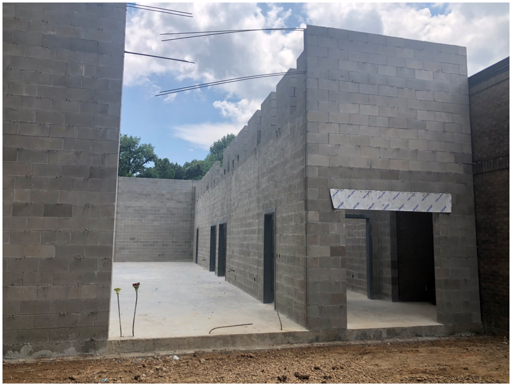
Figure 1 – Interior Block work
