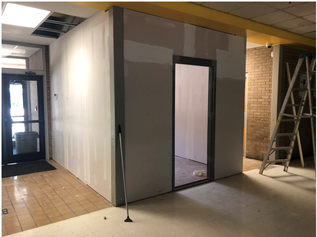
Figure 12 – Mud Work @ Room 114.1
