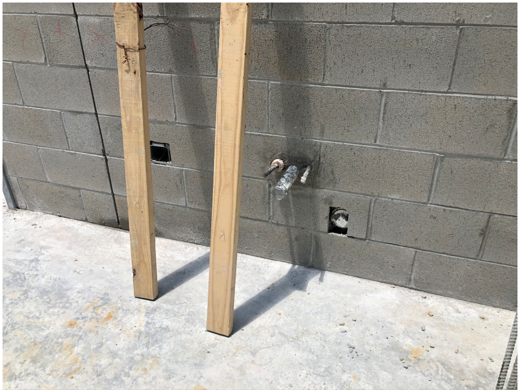
Figure 6 – Rough In Plumbing
