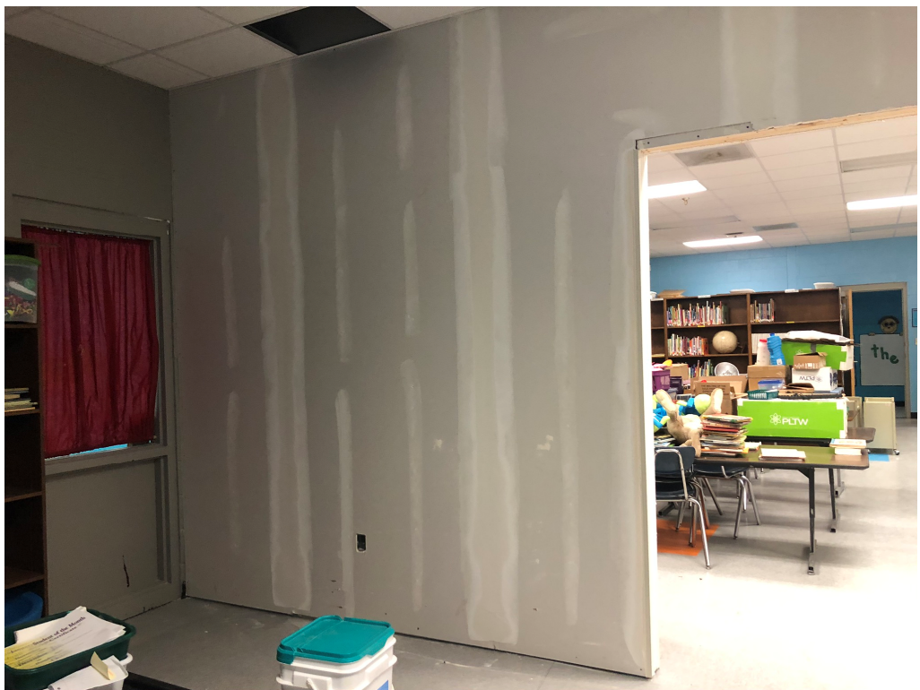
Figure 10 – Mud Work @ Room 170
