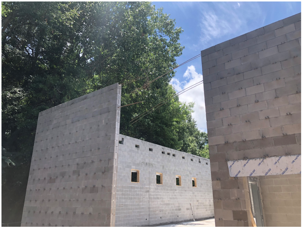
Figure 1 – CMU Block Work
