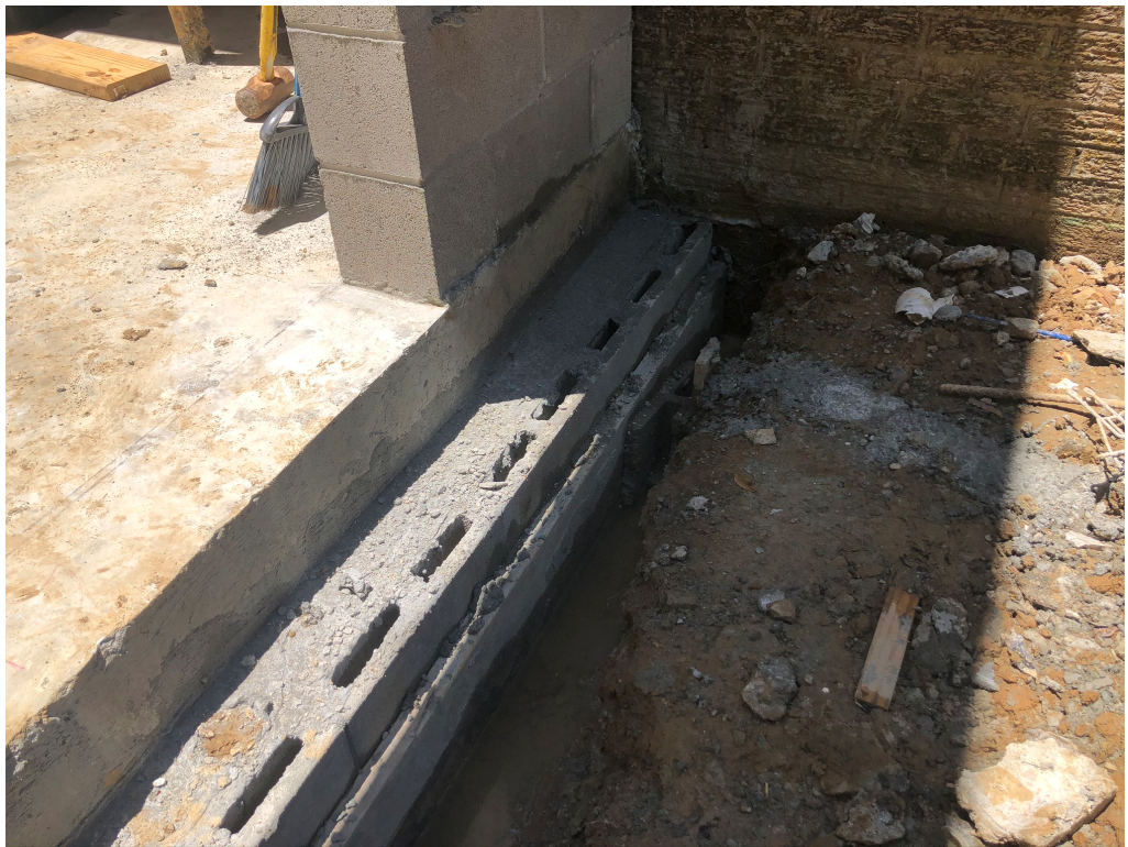
Figure 2 – Brick Ledge for Brick
