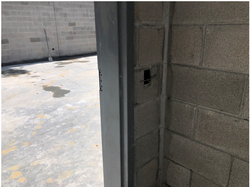
Figure 4 – Electrical Roughed in at CMU
