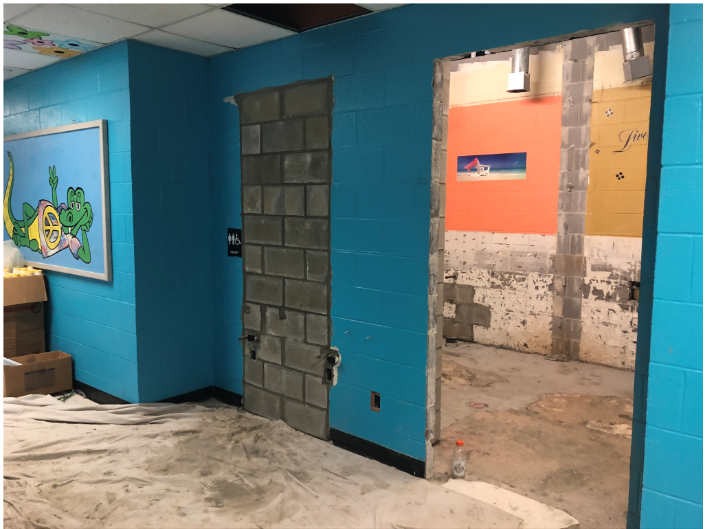
Figure 8 – CMU Blocked in at New ADA Restroom
