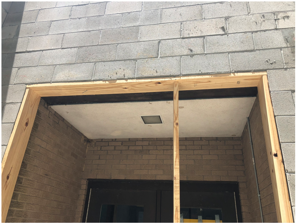
Figure 3 – Temp Support to be removed
