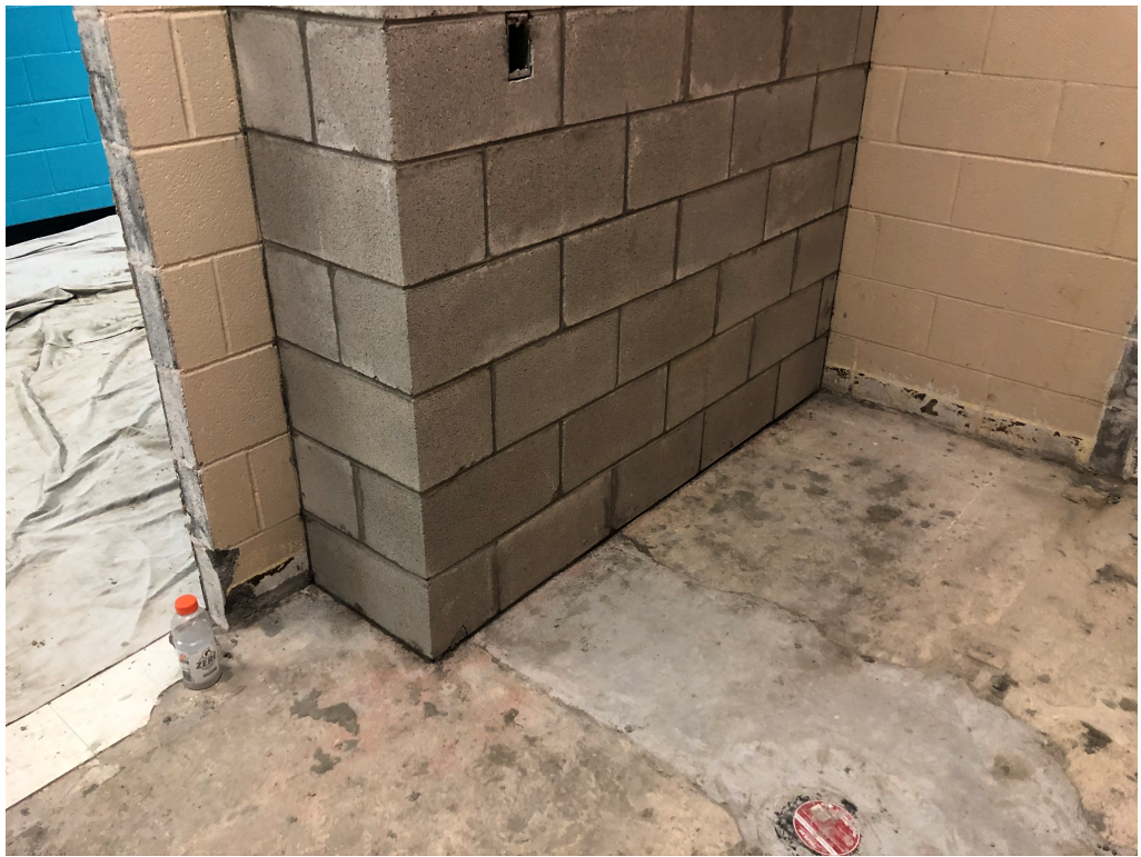
Figure 9 – CMU Blocked in at New ADA Restroom
