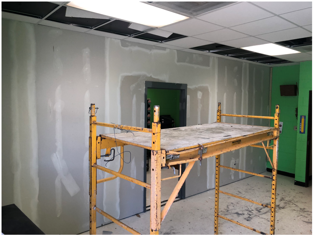
Figure 7 – Mud Work at Room 153
