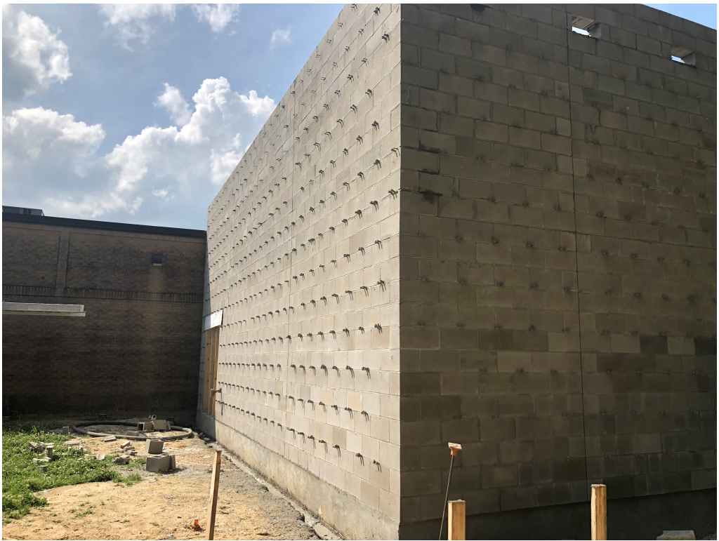
Figure 3 – Southwest Masonry Wall
