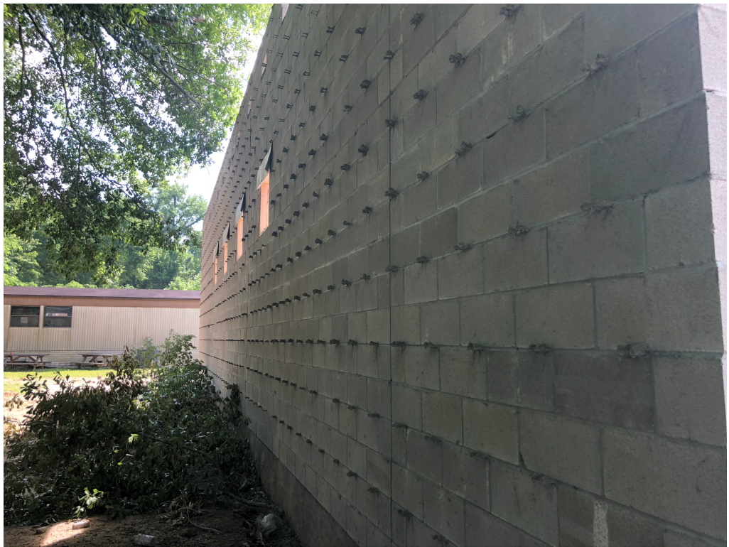
Figure 2 – Rear Masonry Wall
