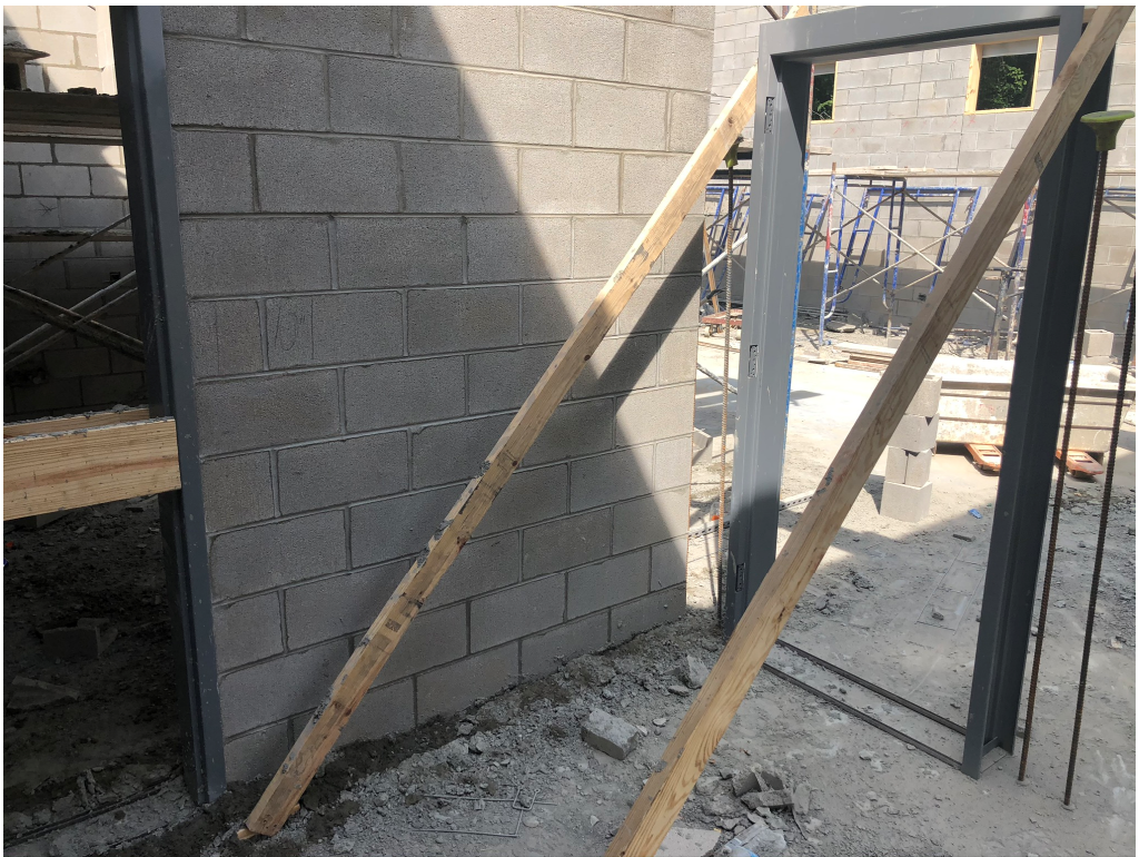
Figure 4 – Temporary Support to HM Door Frame
