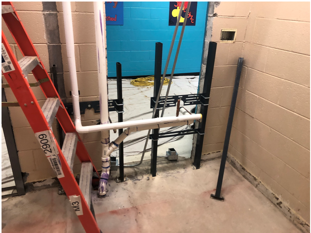
Figure 6 – Rough In Plumbing
