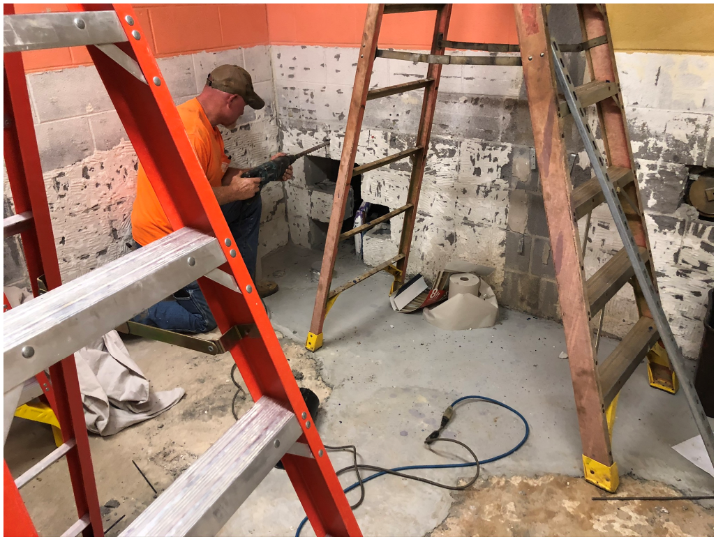
Figure 12 – Plumbing Structure Install
