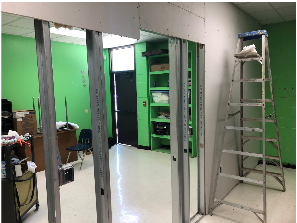
Figure 10 – New Wall at Room 153
