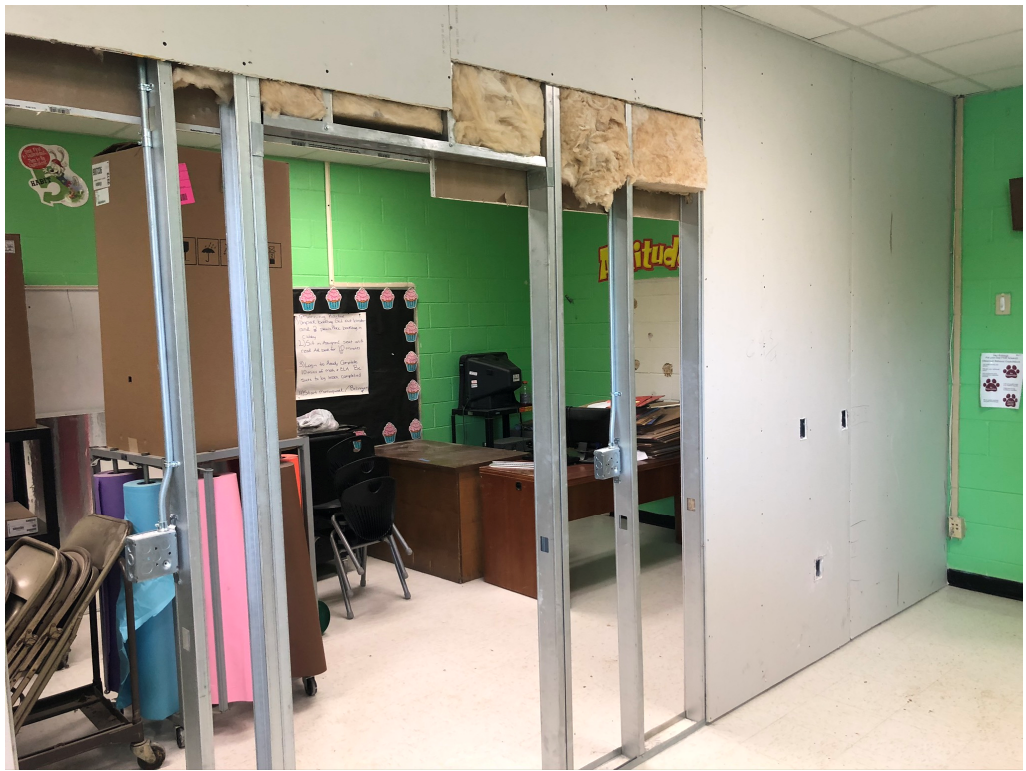
Figure 9 – New Wall at Room 153
