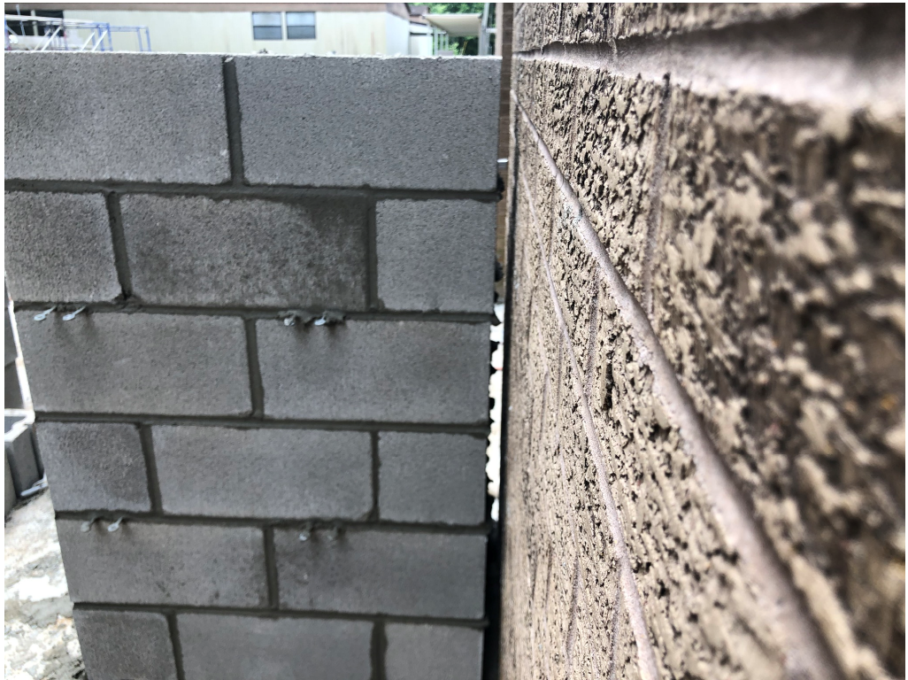
Figure 2 – Gap for Expansion Joint
