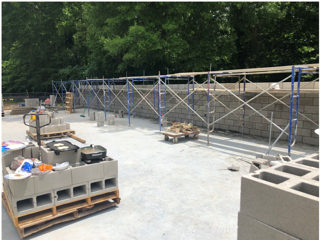
Figure 8 – CMU Work Ongoing
