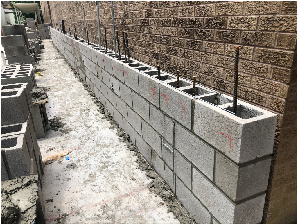
Figure 3 – New Bearing Wall Construction Ongoing
