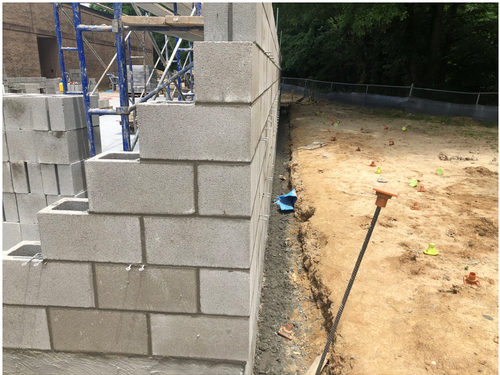
Figure 4 – Rear Wall at Addition
