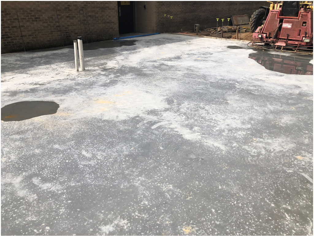
Figure 3 – Slab is Dry
