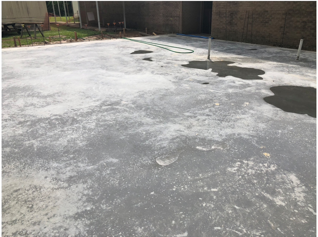
Figure 2 – Slab is Dry
