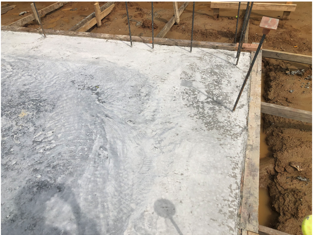
Figure 4 – Reinforcing set at Perimeter
