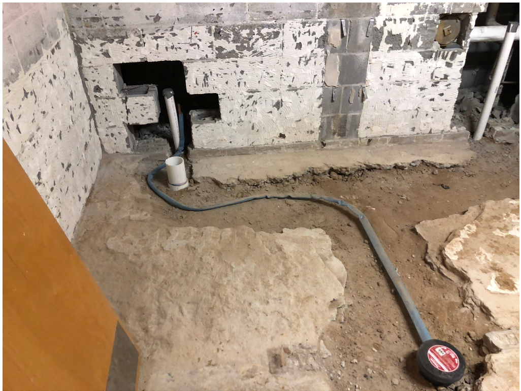
Figure 6 – Interior Supply Line Installed
