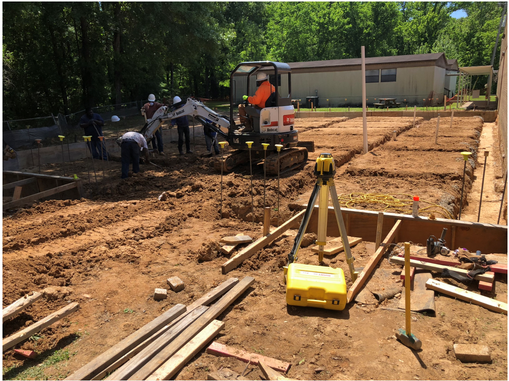
Figure 1 – Footing Trenching in Progress
