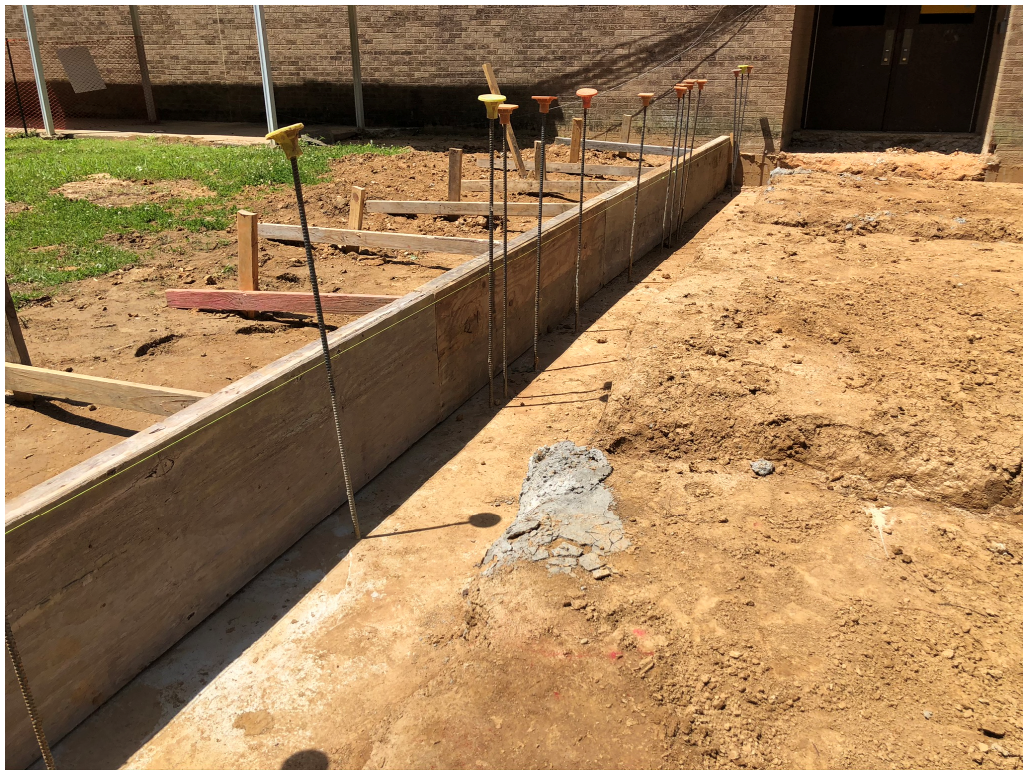
Figure 5 – Perimeter Footing Poured
