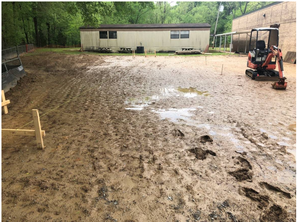
Figure 2 – Batter Boards set and Pad to grade
