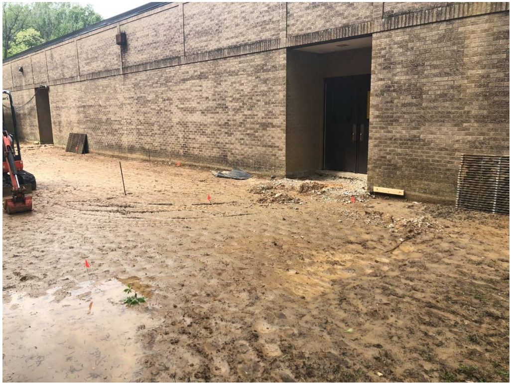
Figure 3 – Apron concrete Removed at entry
