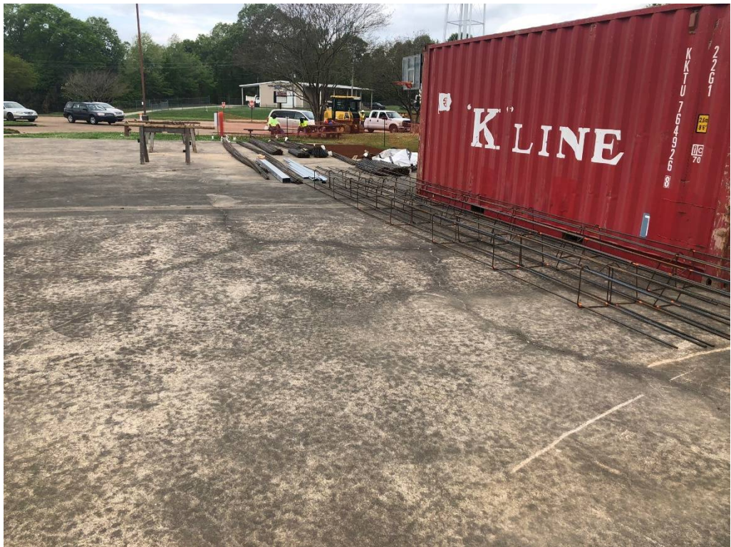
Figure 4 – Rebar Work Begun
