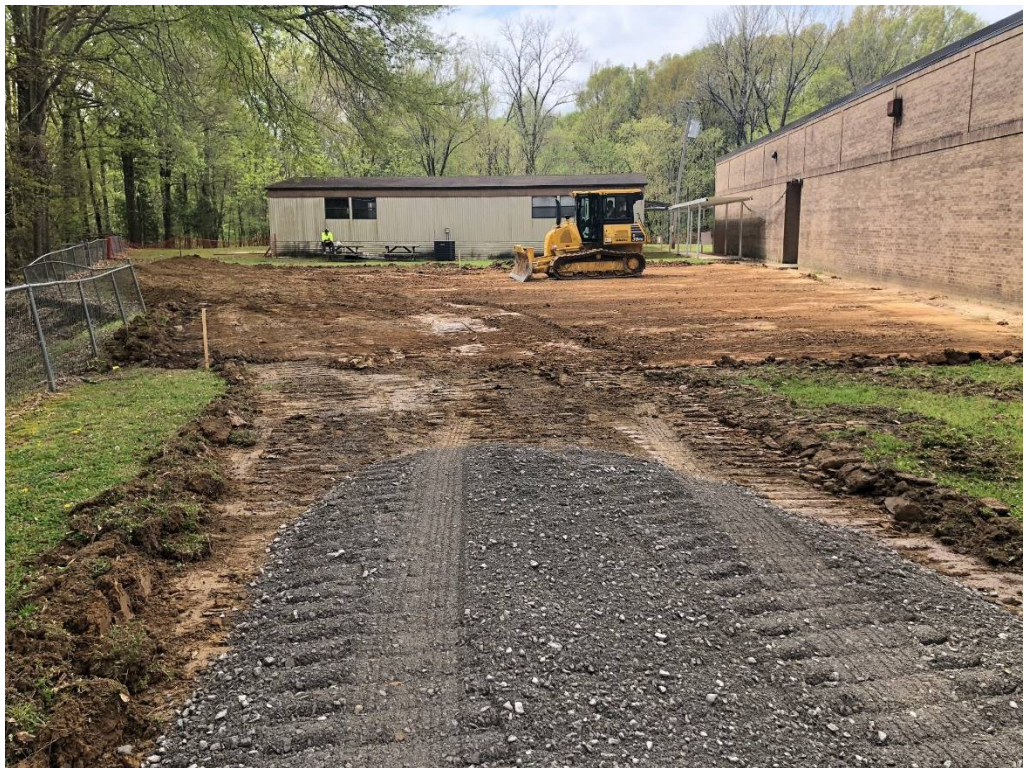
Figure 2 – Pad Prep for Addition
