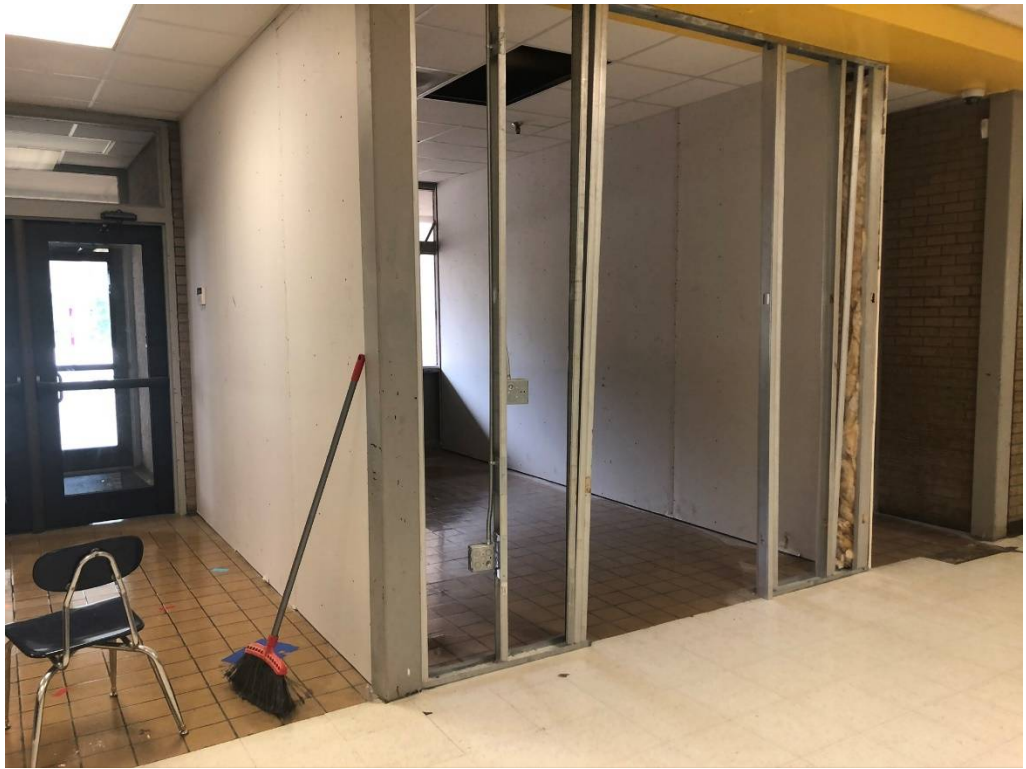
Figure 5 – Storage Room @ Cafeteria Progress
