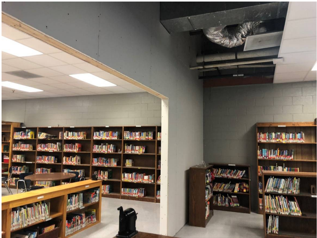
Figure 4 – Steam Lab Dividing Wall Progress
