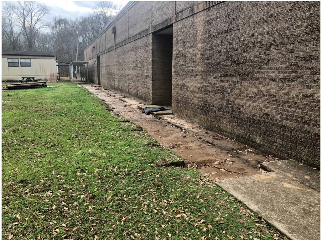
Figure 11 – Prep at East Side for Addition
