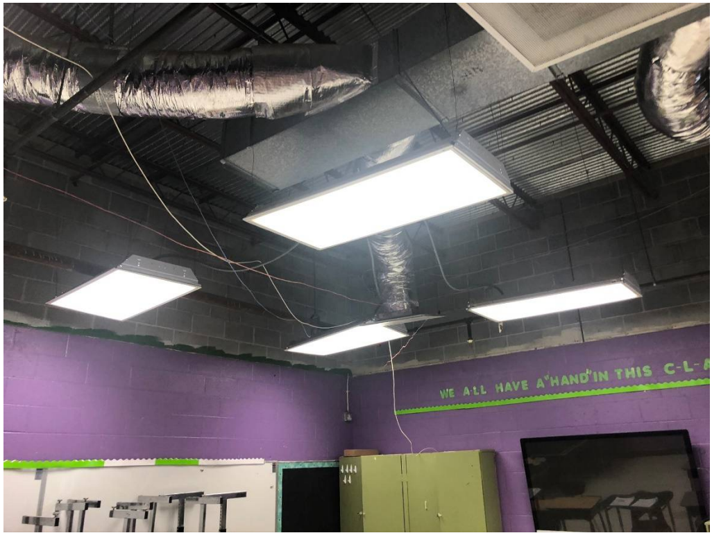
Figure 9 – RM 195 Ceiling Demo
