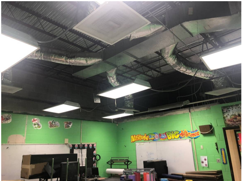
Figure 8 – RM 153 Ceiling Demo
