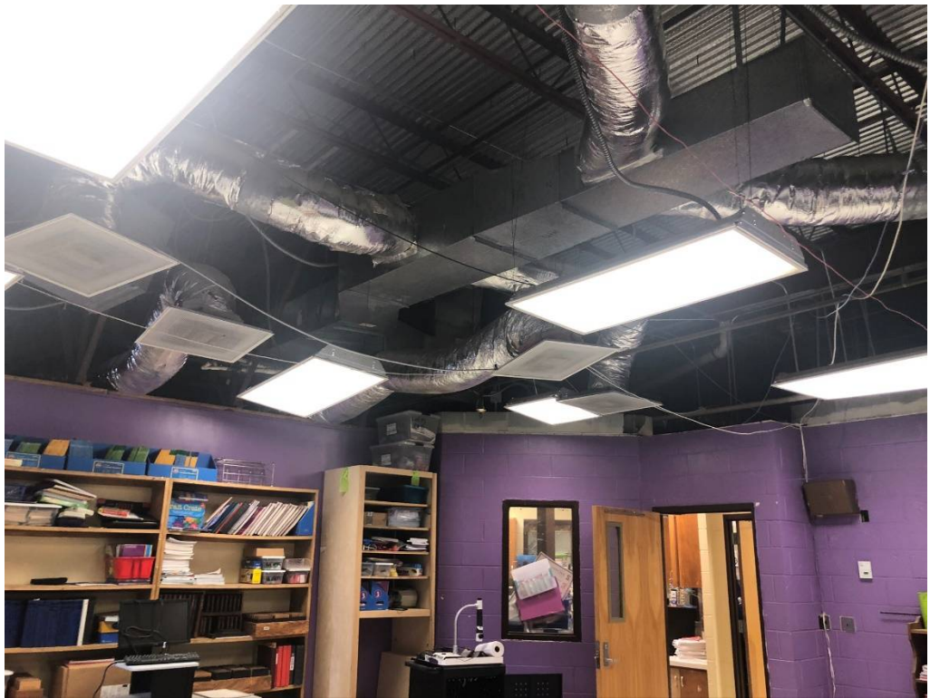
Figure 10 – RM 195 Ceiling Demo
