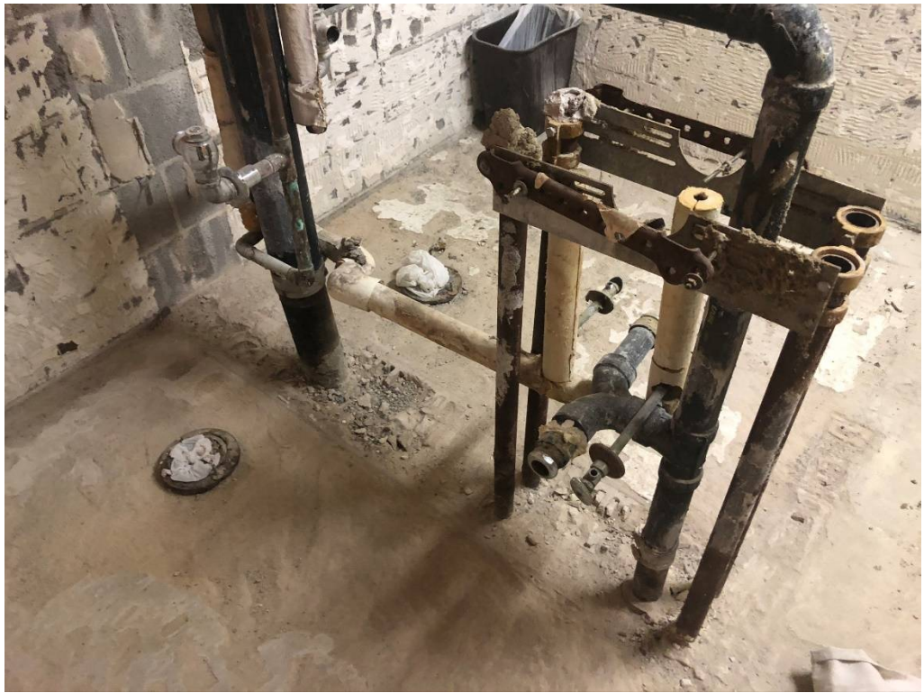
Figure 5 – Existing Plumbing @ Restroom
