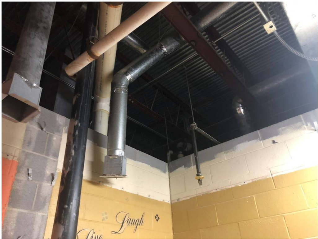
Figure 4 – Restroom Above Ceiling
