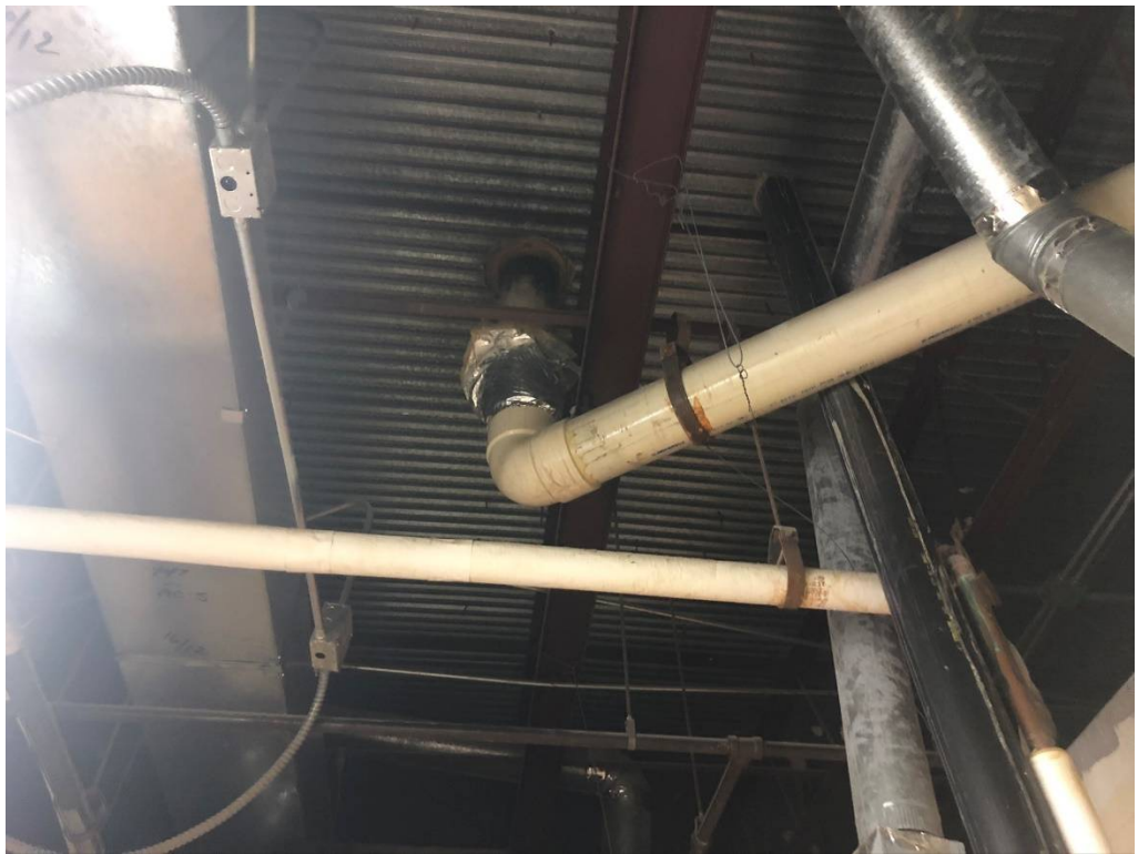
Figure 6 – Roof Drain Above Restroom
