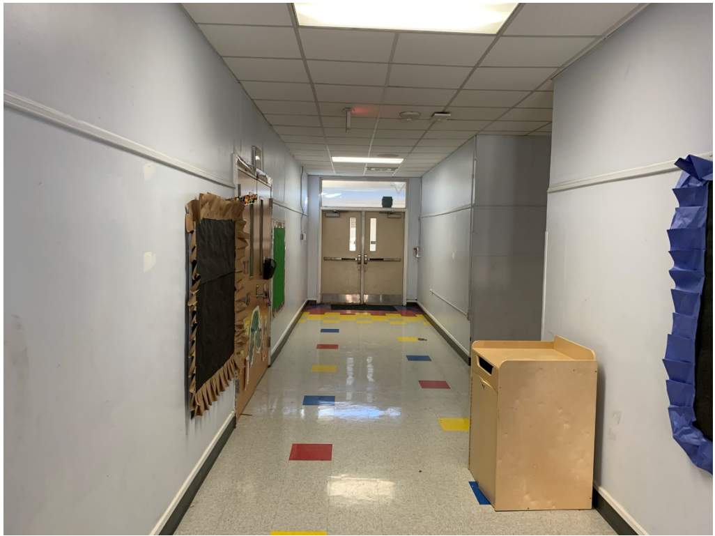
Figure 1 – Paint Prep at Halls
