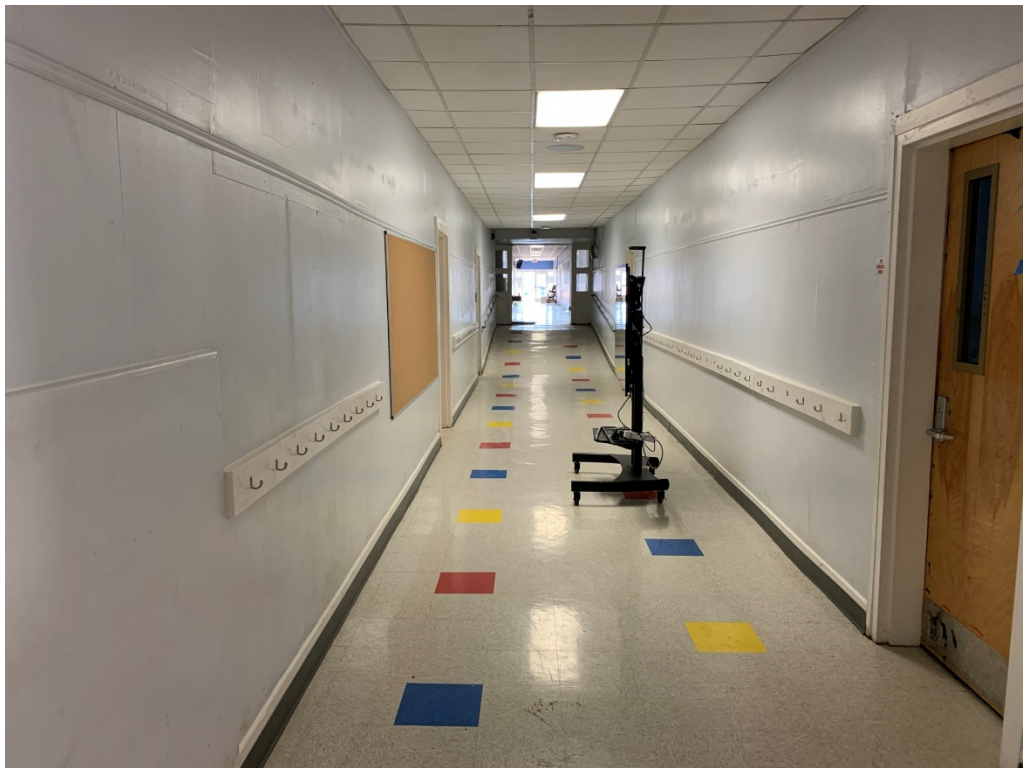
Figure 2 – Paint Prep at Halls
