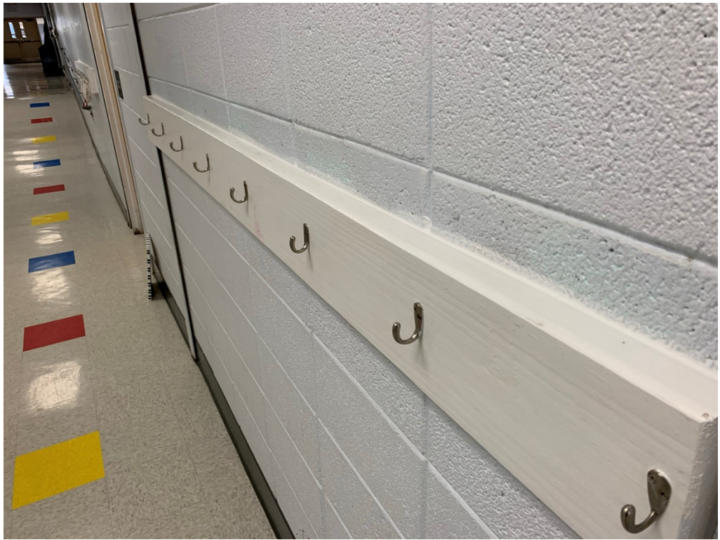
Figure 3 – Paint Prep at Halls
