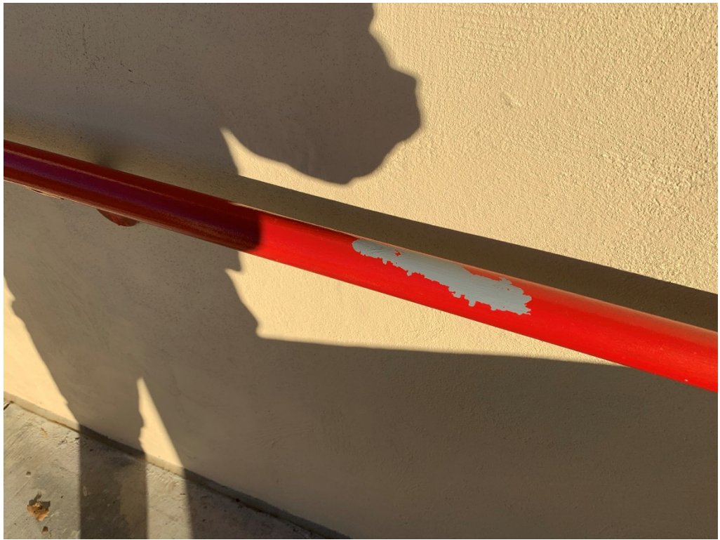
Figure 7 – Handrail paint is Ongoing
