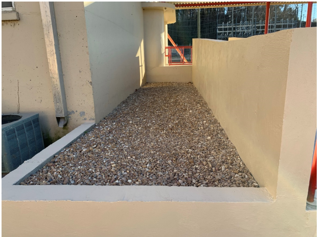
Figure 8 – Rock Installed at Planter
