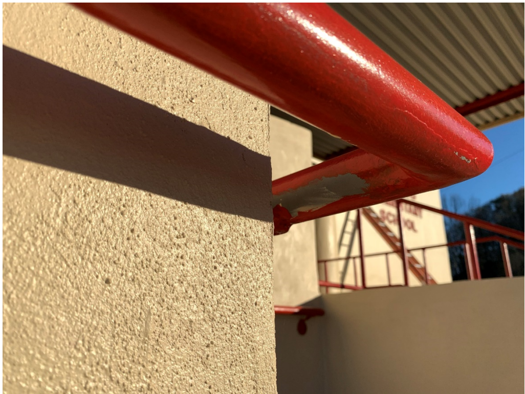
Figure 6 – Handrail paint is Ongoing
