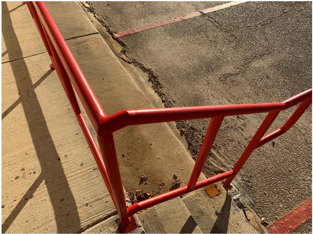
Figure 5 – Handrail paint is Ongoing
