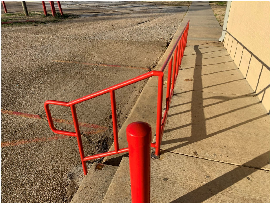
Figure 4 – Handrail paint is Ongoing
