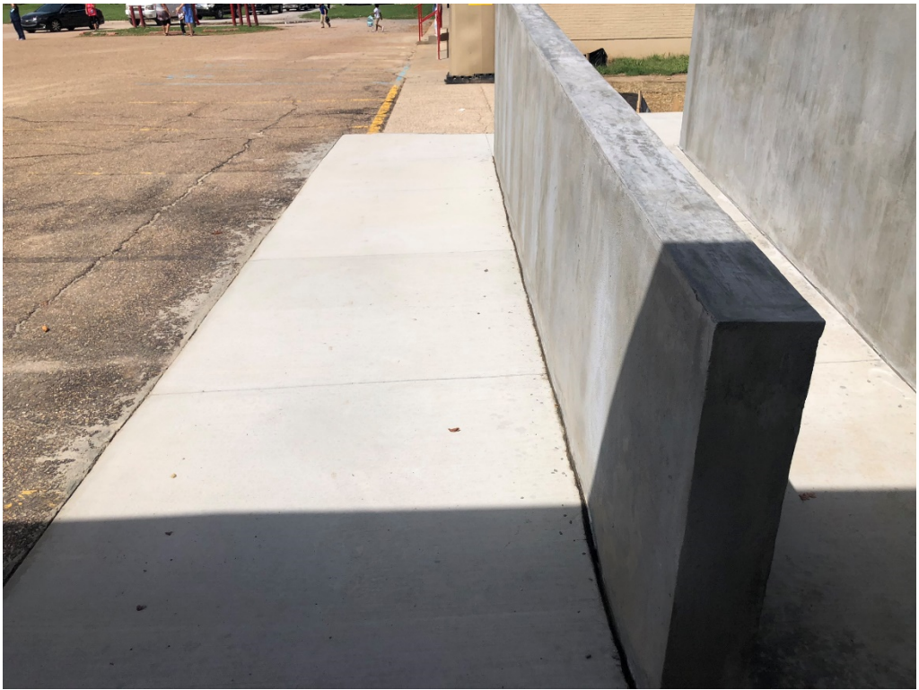
Figure 5 – Front Entry Sidewalks Poured
