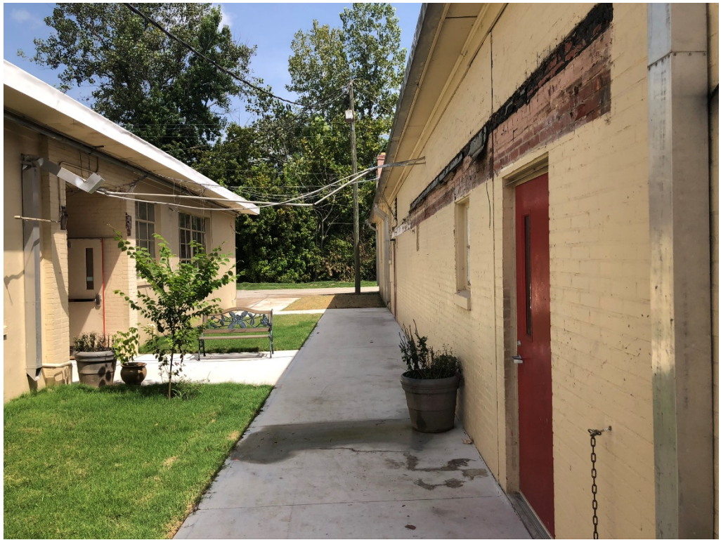
Figure 1 – Demo of Canopy still requires removal of asphalt & asphalt flashing
