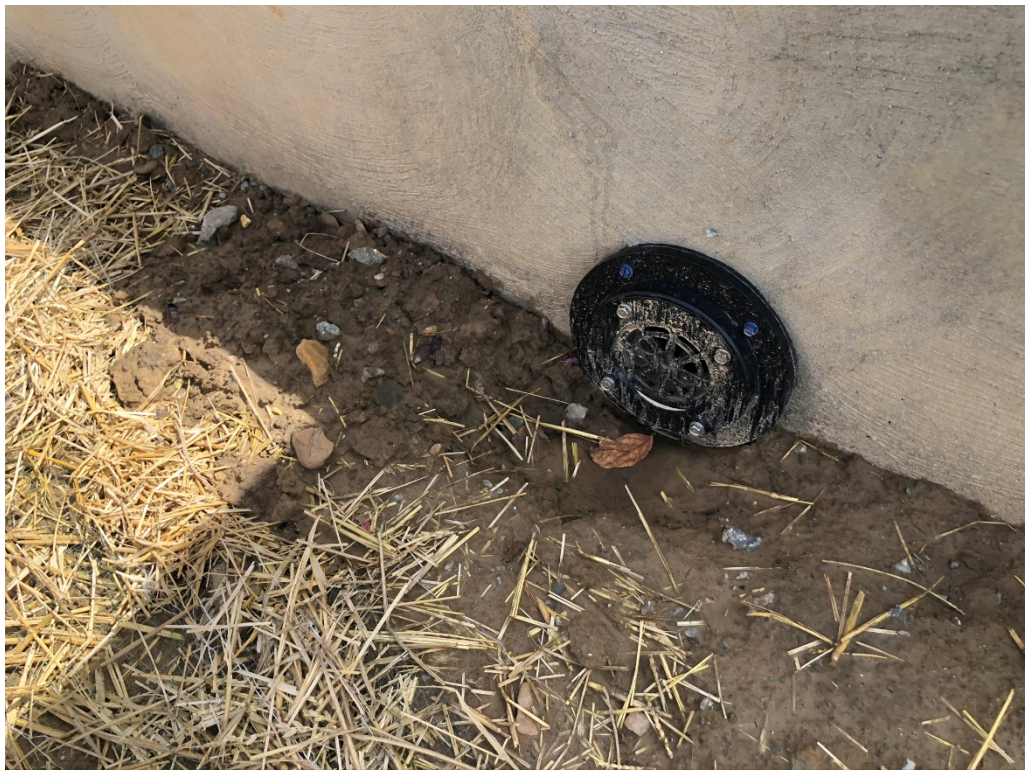
Figure 8 – Drainage Outlets at Planter
