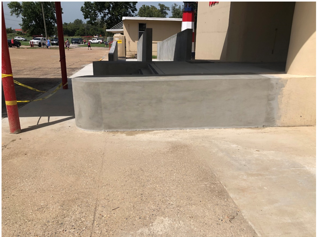
Figure 2 – Concrete Work at Entry
