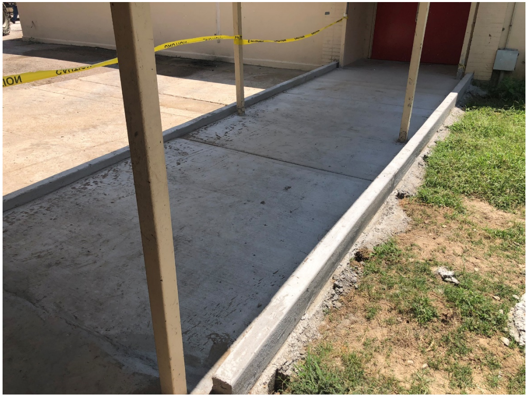
Figure 13 – Concrete Sidewalks Installed
