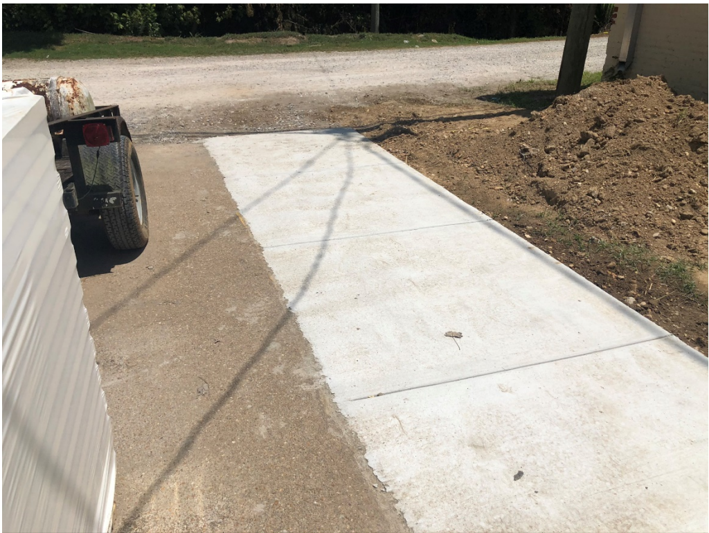
Figure 18 – Concrete Sidewalks Installed
