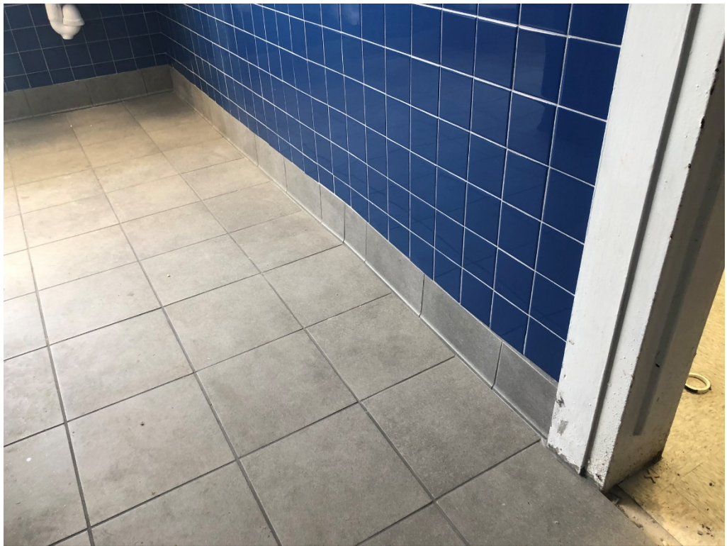
Figure 2 – Tile Installed at Bathrooms
