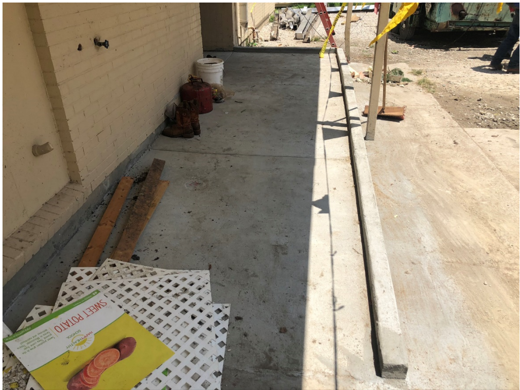
Figure 14 – Concrete Sidewalks Installed
