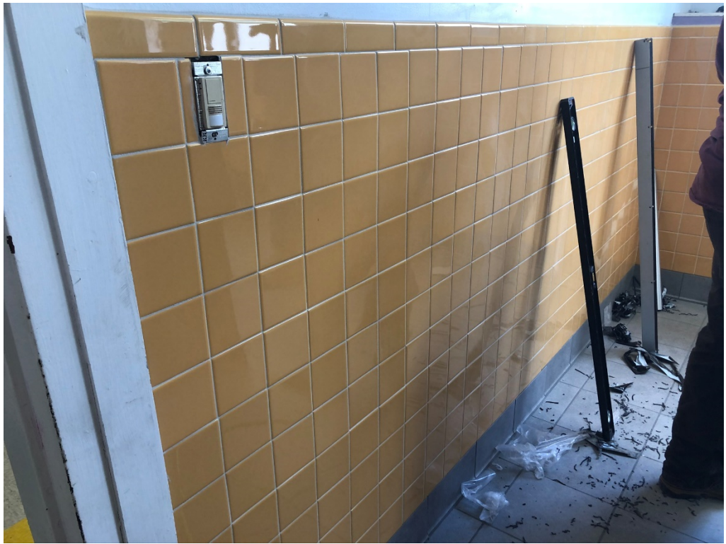
Figure 9 – Tile Installed at Bathrooms
