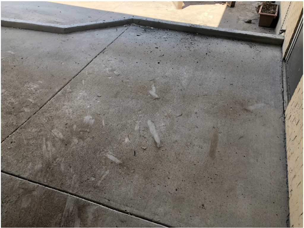
Figure 15 – Concrete Sidewalks Installed
