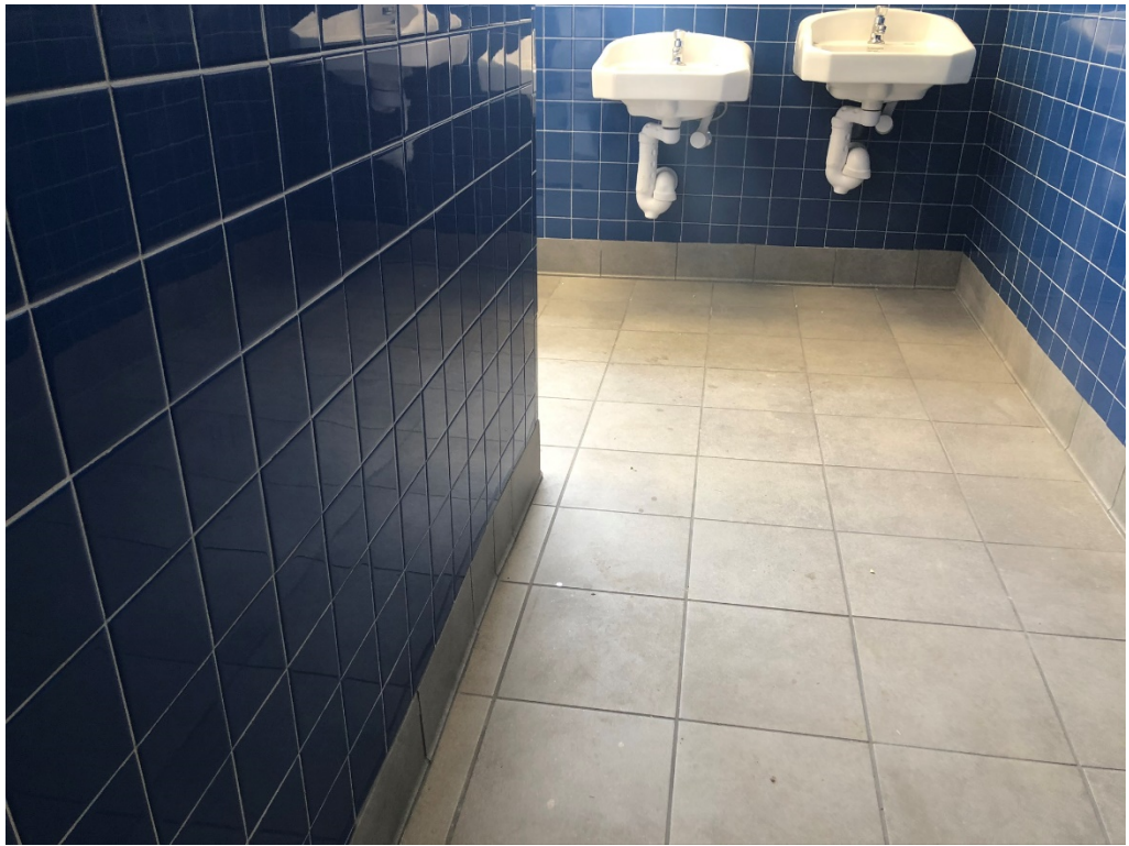
Figure 3 – Tile Installed at Bathrooms
