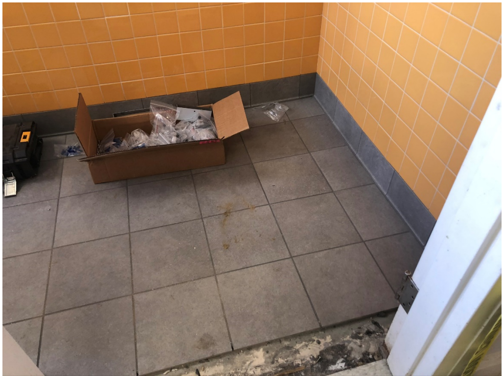
Figure 8 – Tile Installed at Bathrooms
