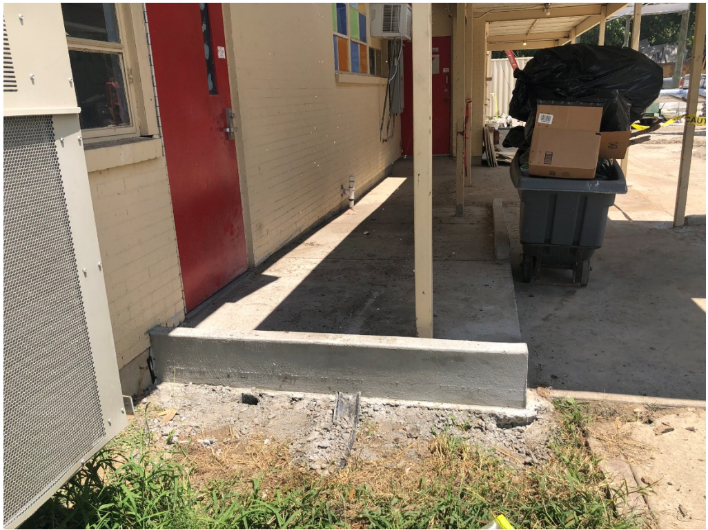
Figure 11 – Concrete Sidewalks Installed
