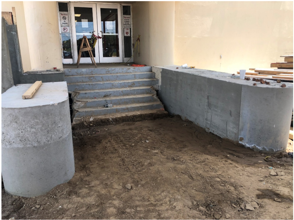
Figure 1 – Entry Concrete Work
