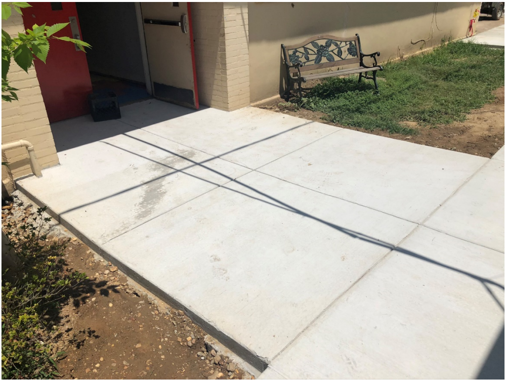
Figure 21 – Concrete Sidewalks Installed
