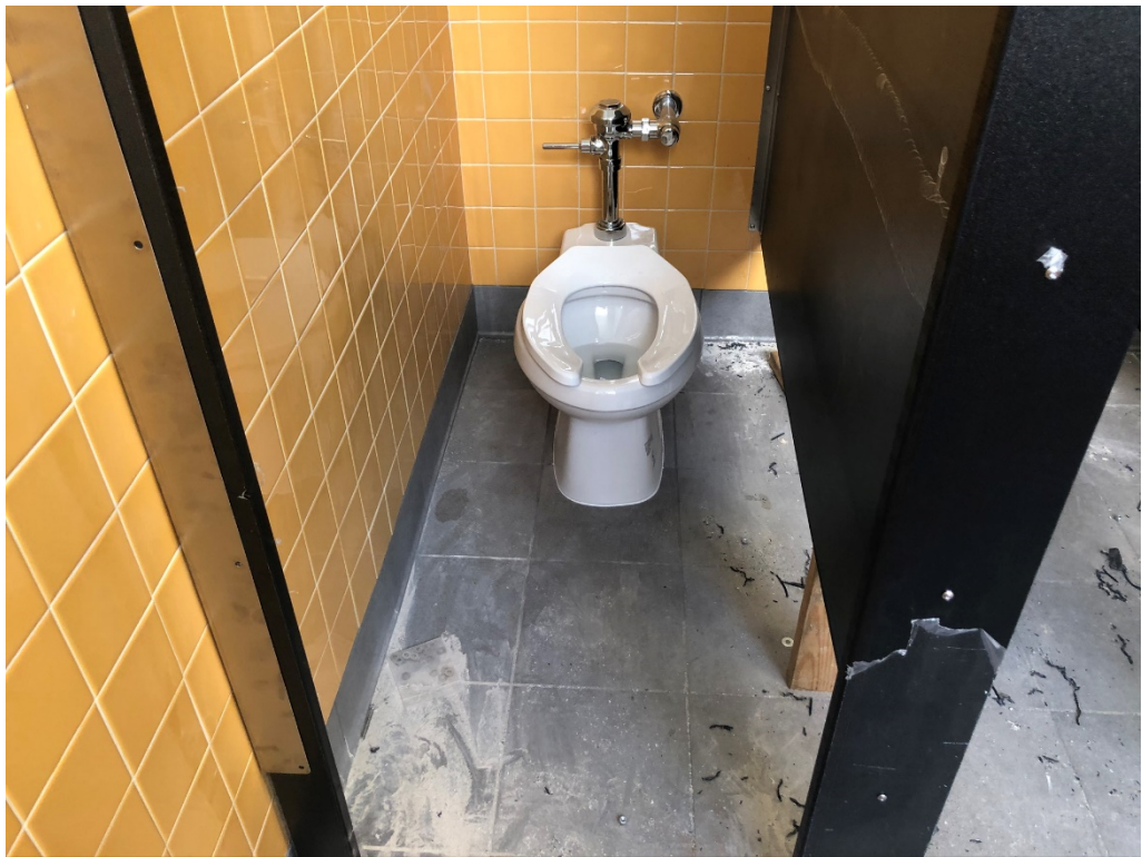
Figure 10 – Partitions and Fixtures Installed
