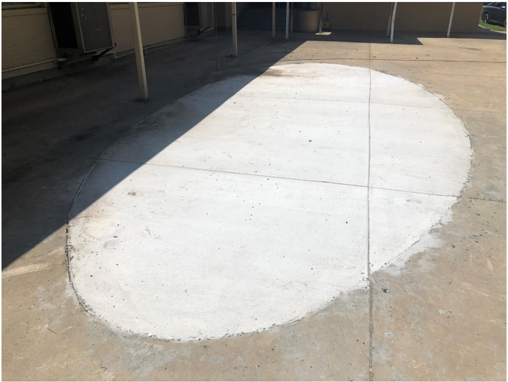
Figure 17 – Concrete Sidewalks Installed
