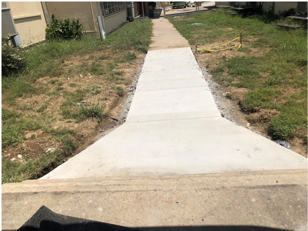
Figure 12 – Concrete Sidewalks Installed
