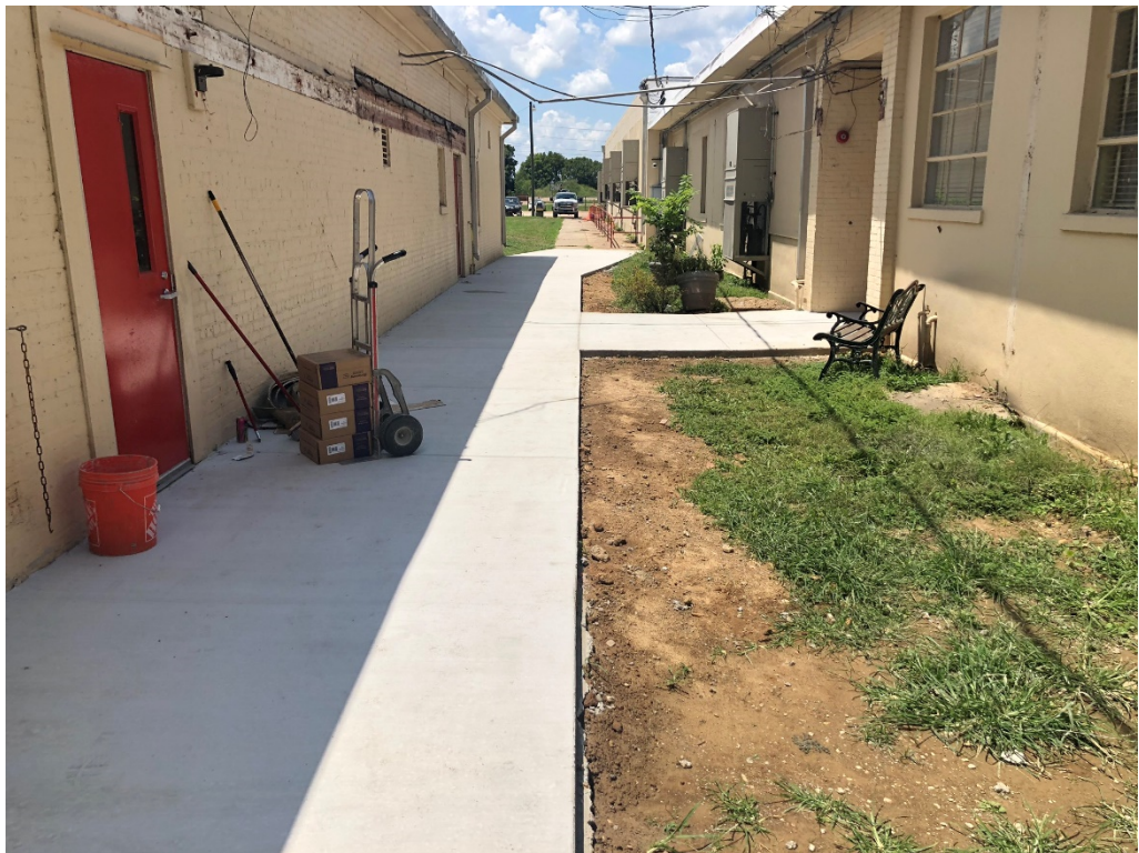
Figure 20 – Concrete Sidewalks Installed
