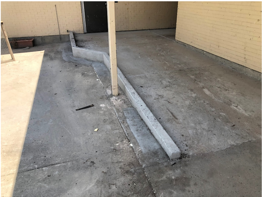
Figure 16 – Concrete Sidewalks Installed
