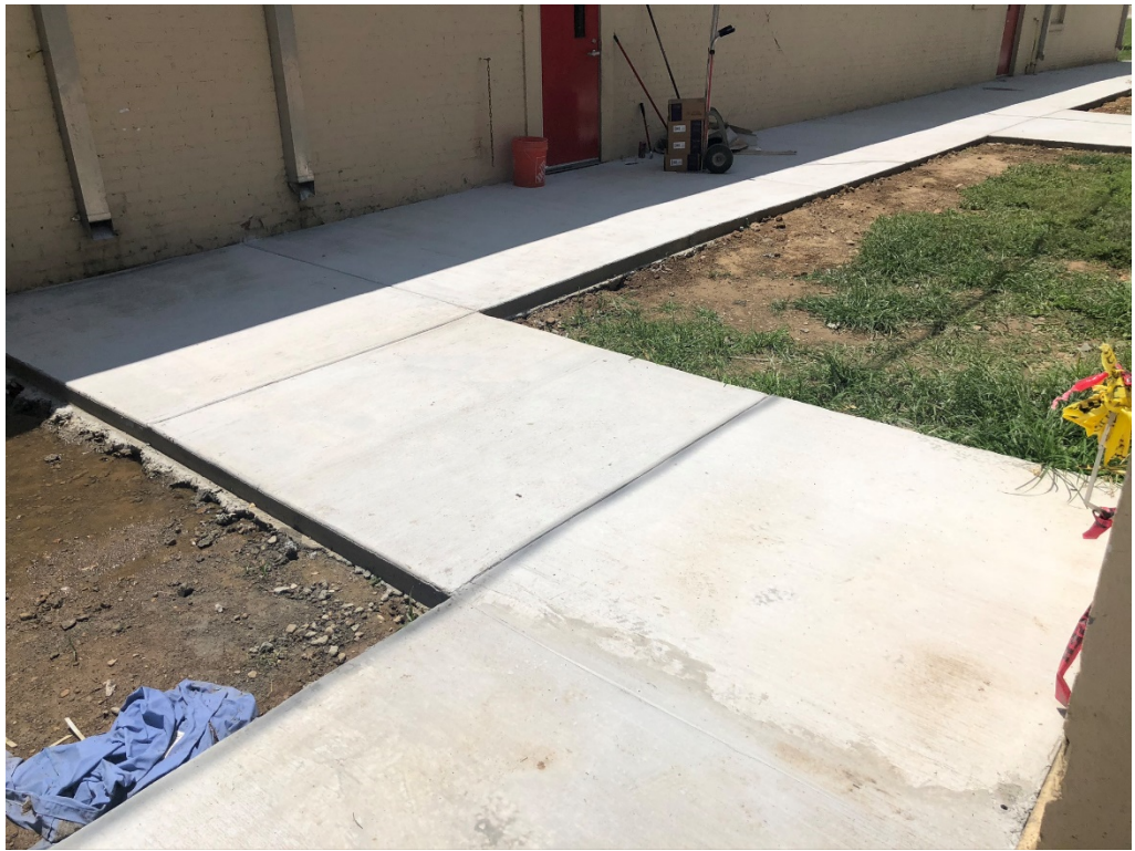
Figure 19 – Concrete Sidewalks Installed
