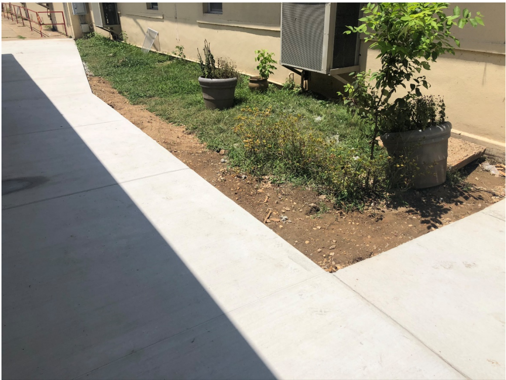
Figure 22 – Concrete Sidewalks Installed
