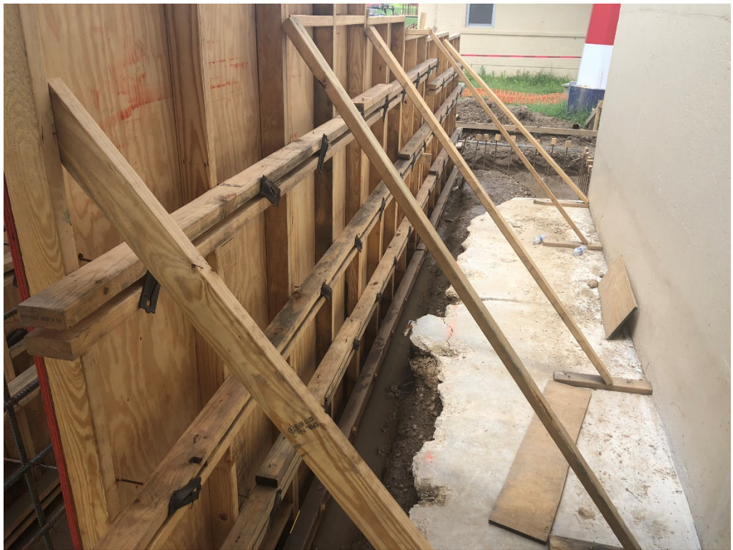
Figure 2 – Formwork Structure
