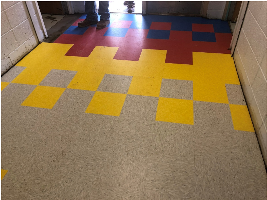
Figure 6 – VCT Flooring Installed
