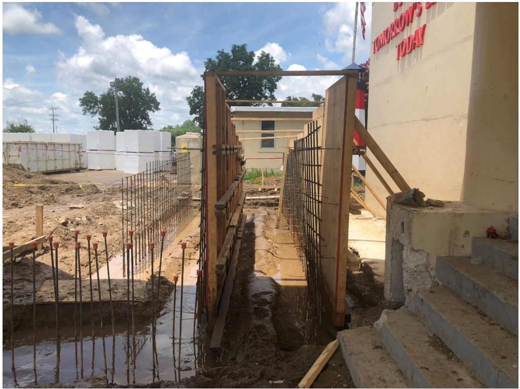
Figure 1 – Formwork Begun @ Ramp
