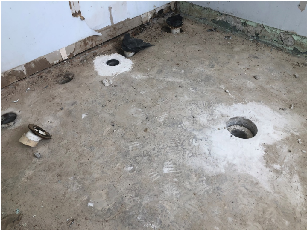
Figure 4 – Core drilling at Bathroom for new Drains
