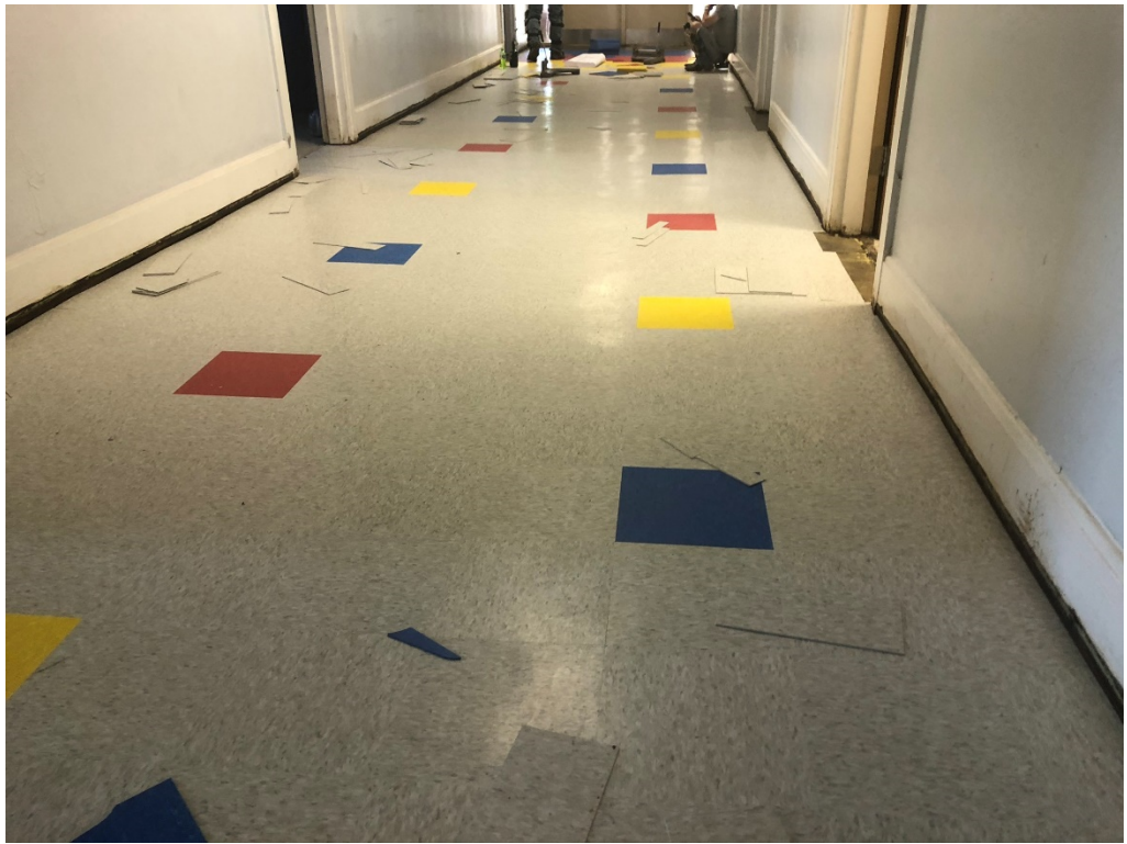
Figure 5 – VCT Flooring Installed
