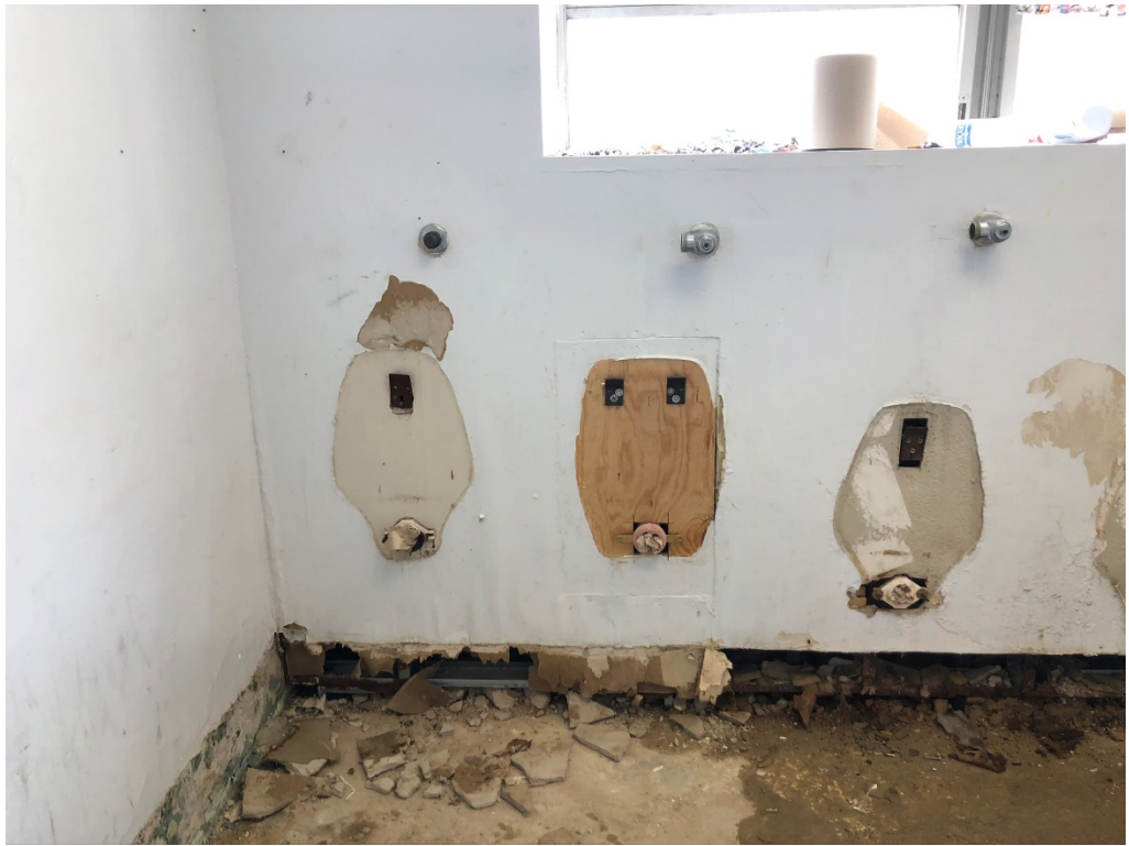
Figure 5 – Bare Plywood should be Sealed with Waterproofing Before Tile Work Begins
