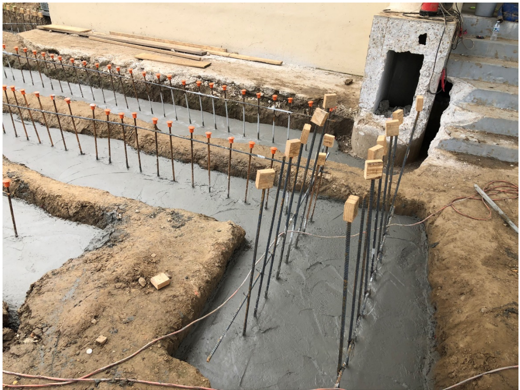
Figure 2 – Footing Concrete Installed
