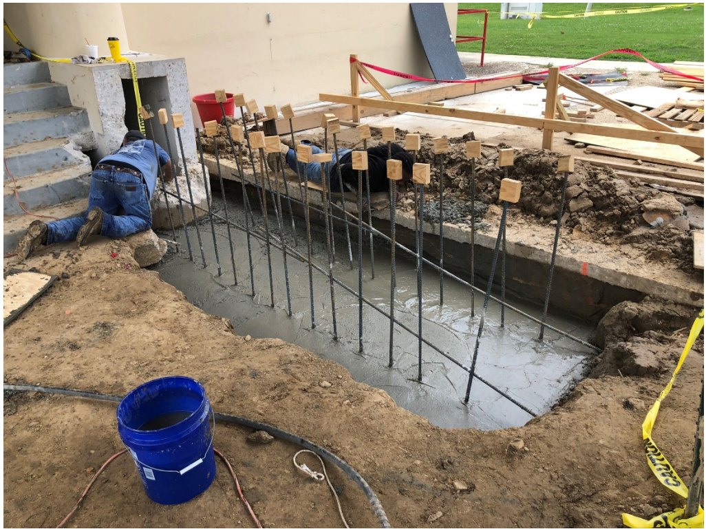
Figure 3 – Footing Concrete Installed
