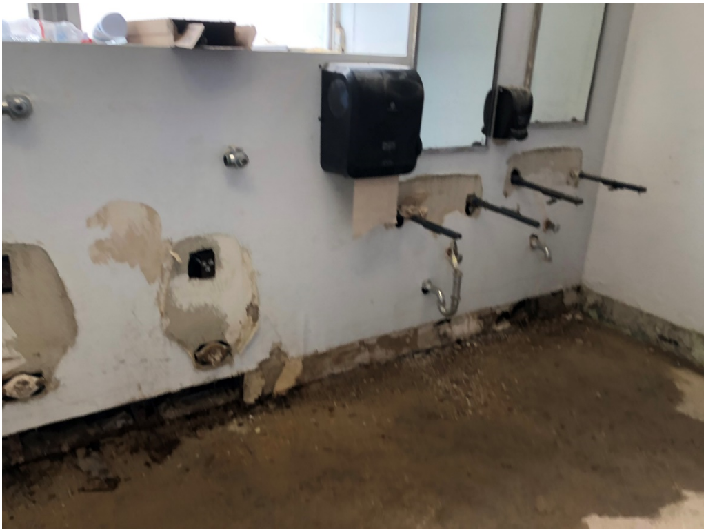
Figure 7 – E-128 Fixtures Removed
