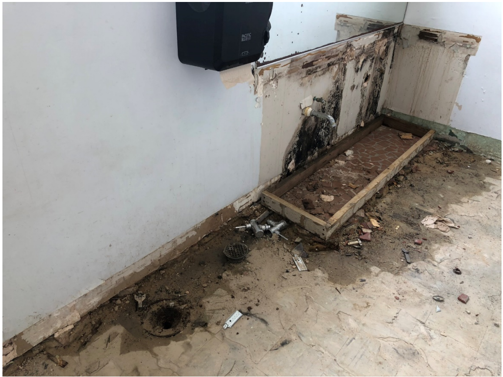
Figure 9 – E-109 Lavatory Demoed
