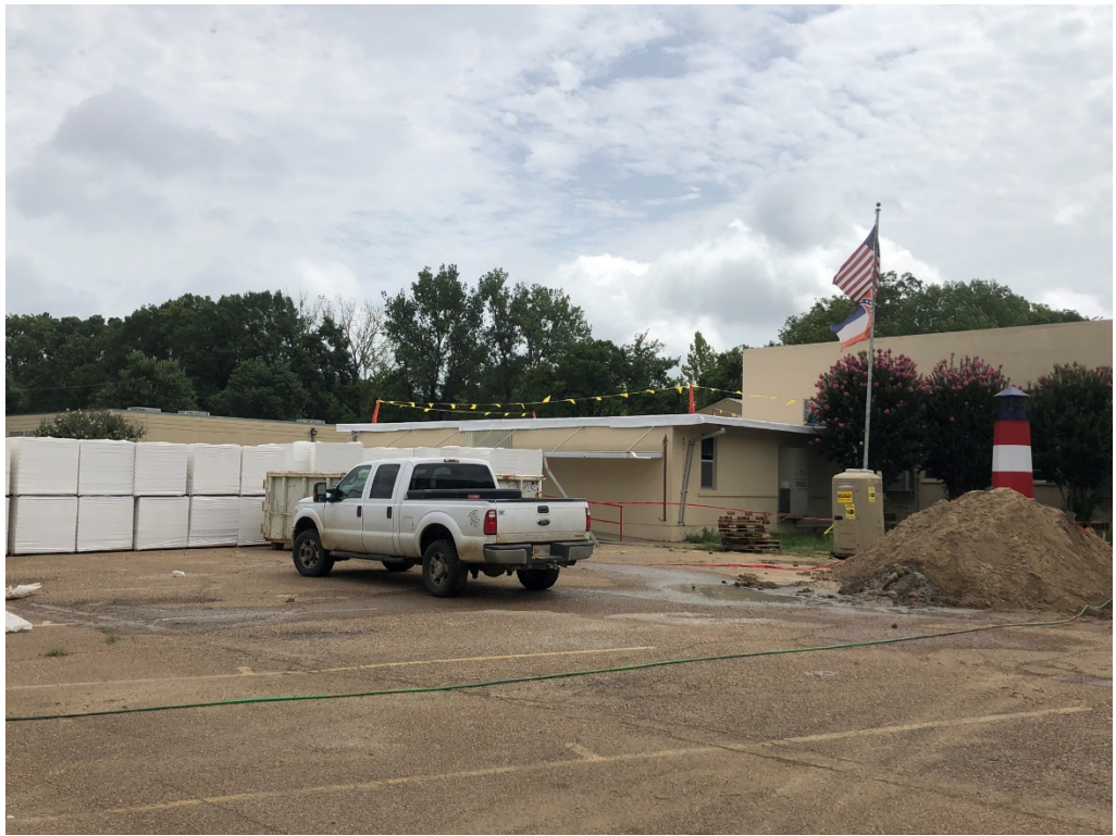
Figure 1 – Roofing Work is Ongoing
