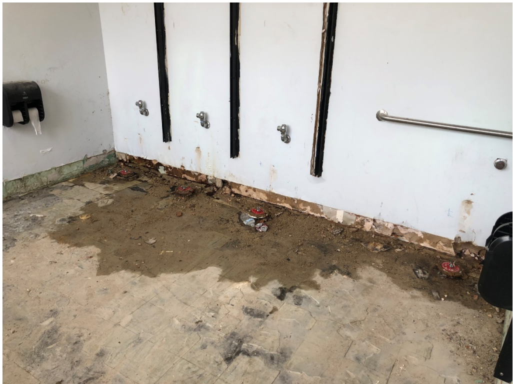
Figure 10 – E-109 Fixtures Removed
