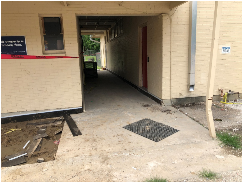
Figure 3 – Contraction Joints Installed
