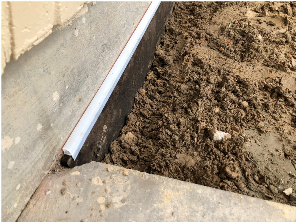
Figure 4 – Contraction Joints Installed
