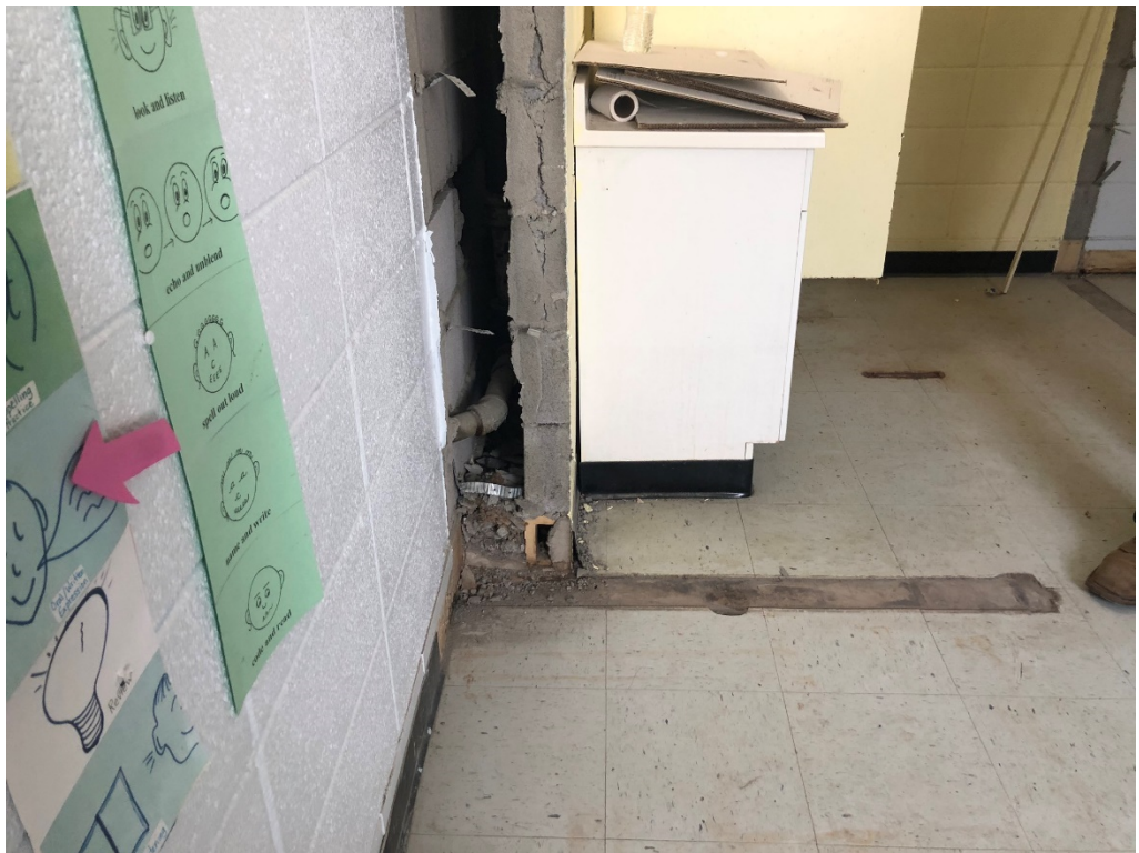
Figure 12 – Wall to Remain to Conceal Plumbing
