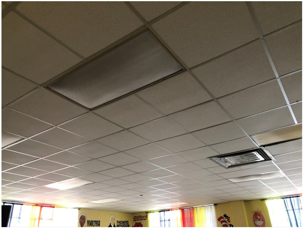
Figure 7 – Library Ceiling Work
