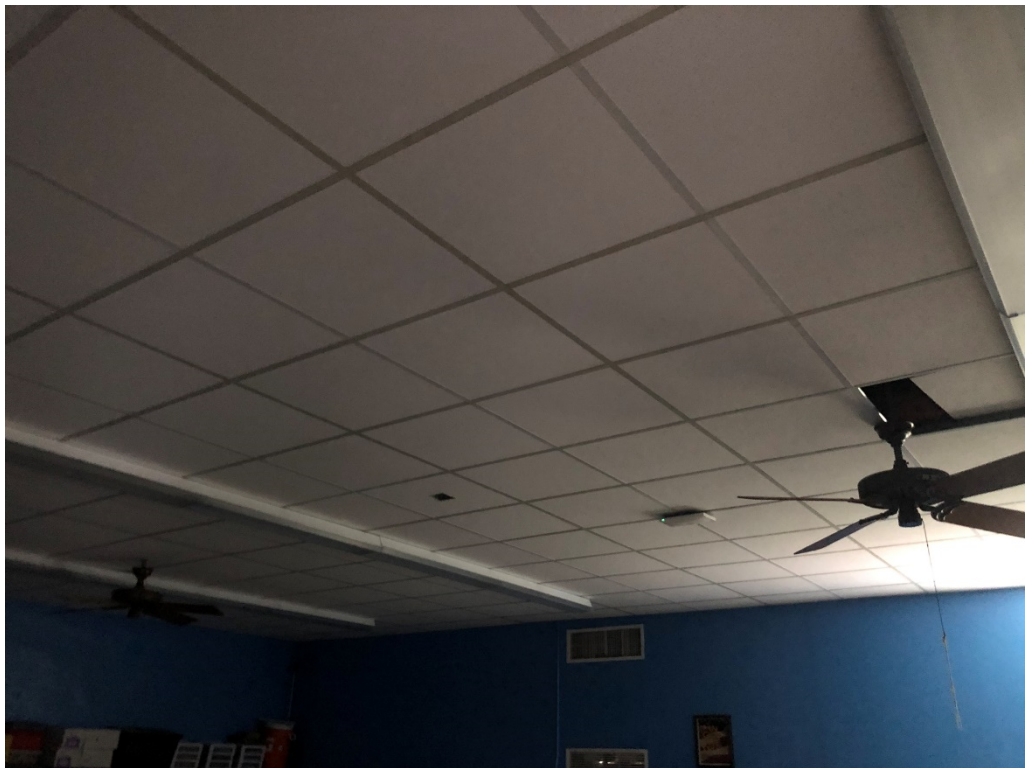
Figure 4 – New Ceiling Installation @ Classrooms is Ongoing
