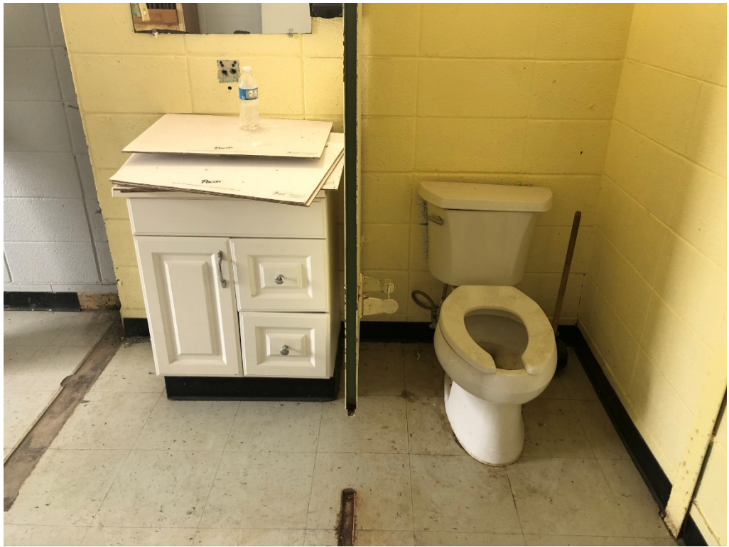
Figure 11 – Plumbing to be Removed
