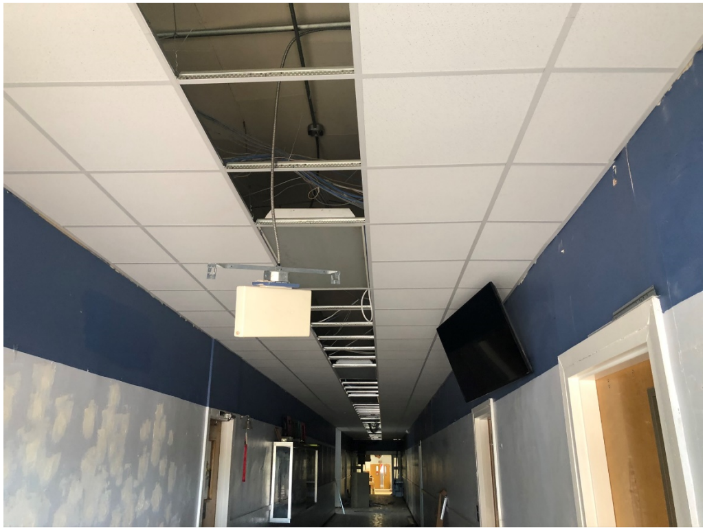
Figure 3 – New Ceiling Installation is Ongoing
