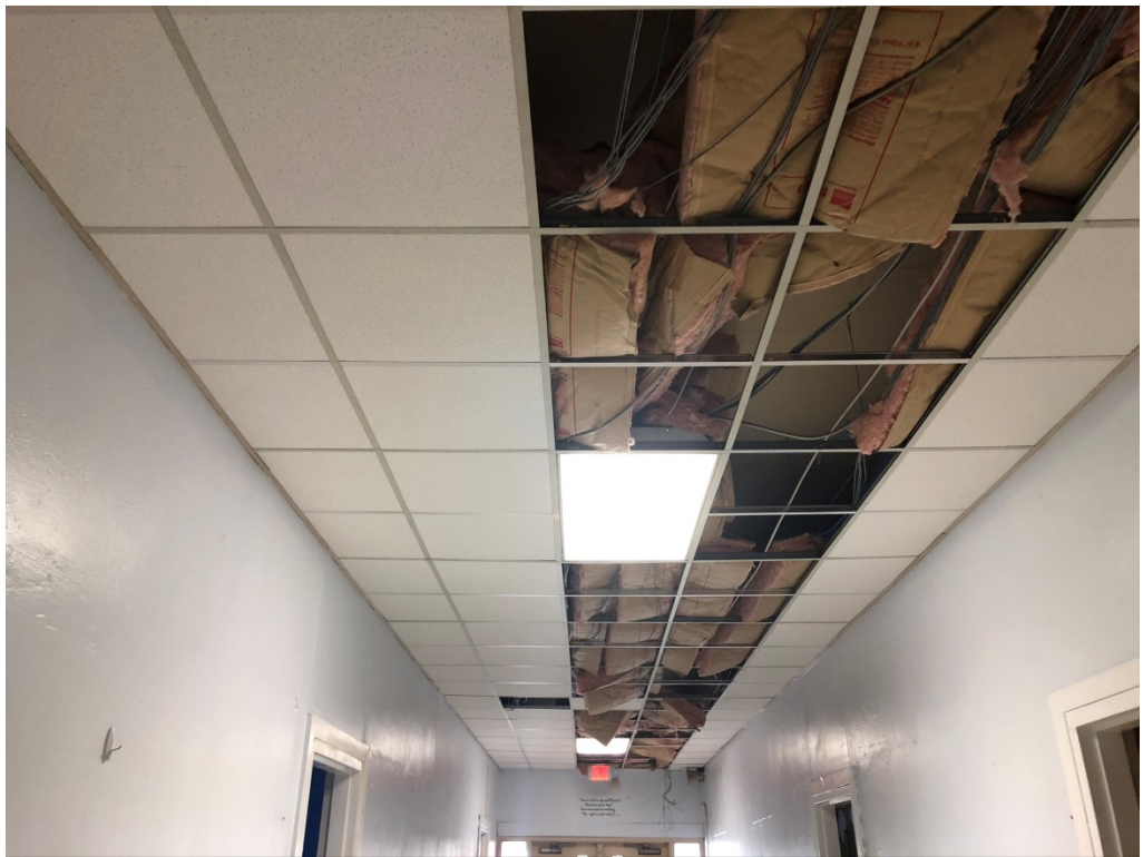
Figure 10 – Hall Ceiling Replacement
