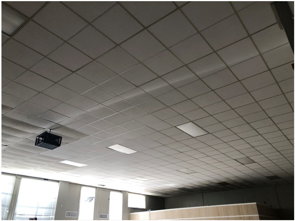
Figure 9 – Auditorium Ceiling Replacement is Ongoing
