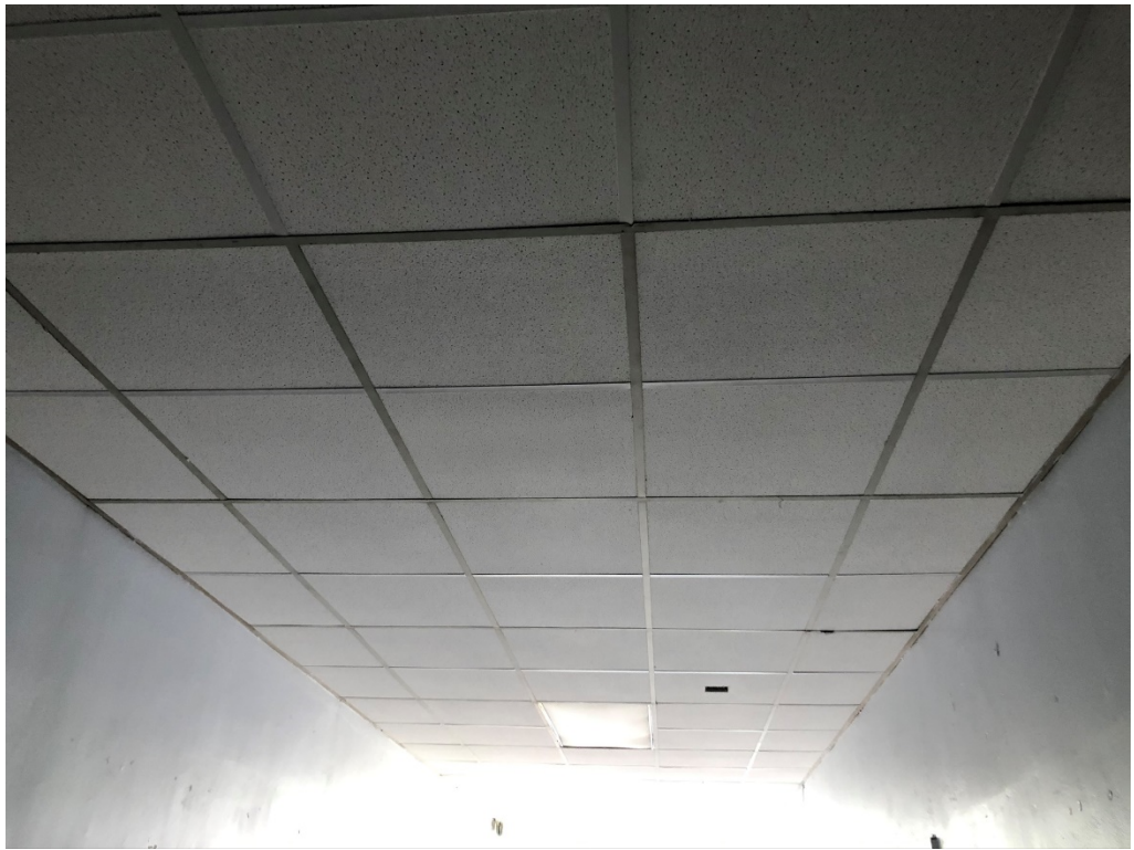
Figure 5 – Ceiling Tile Replacement
