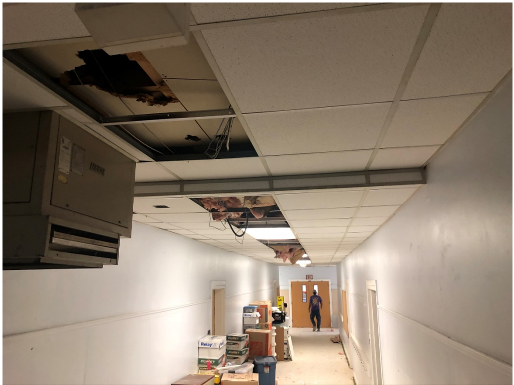
Figure 6 – Ceiling Tile Replacement
