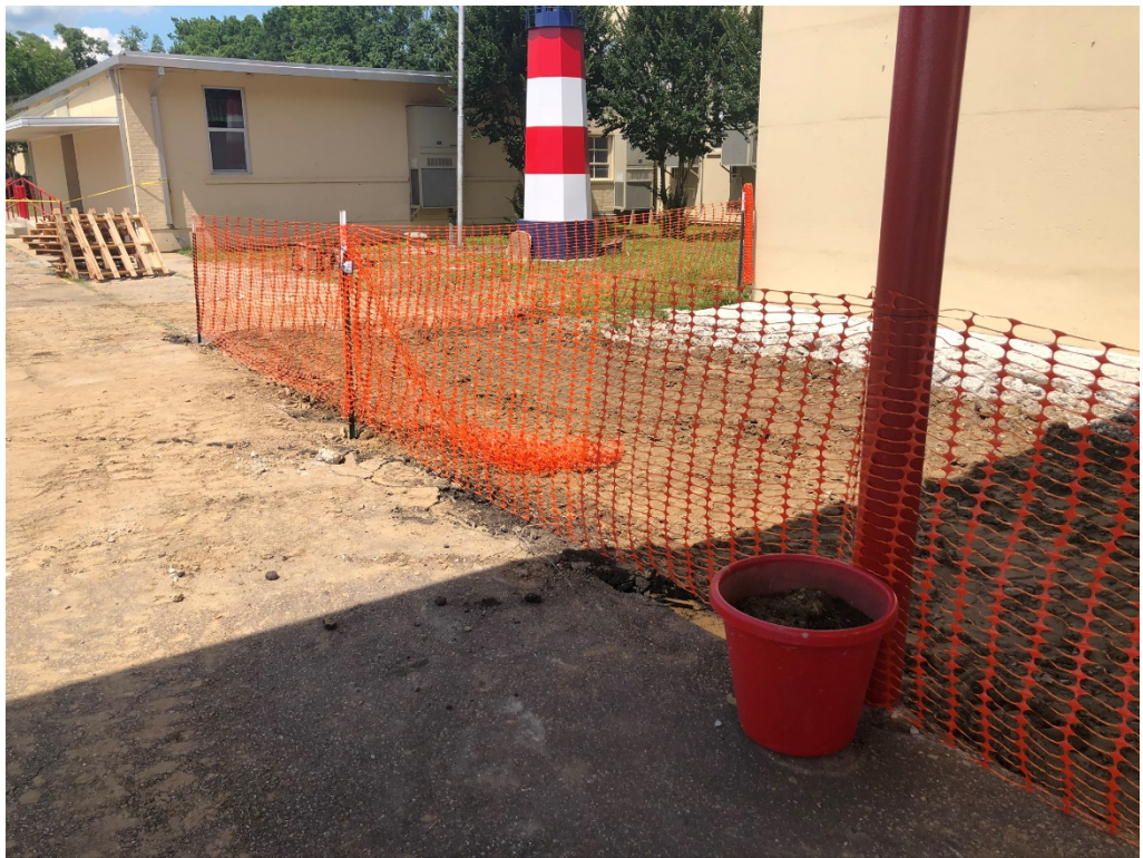
Figure 2 – Entry Demo Work
