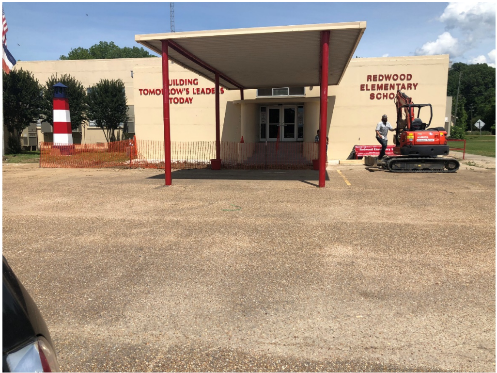
Figure 1 – Entry Demo Work
