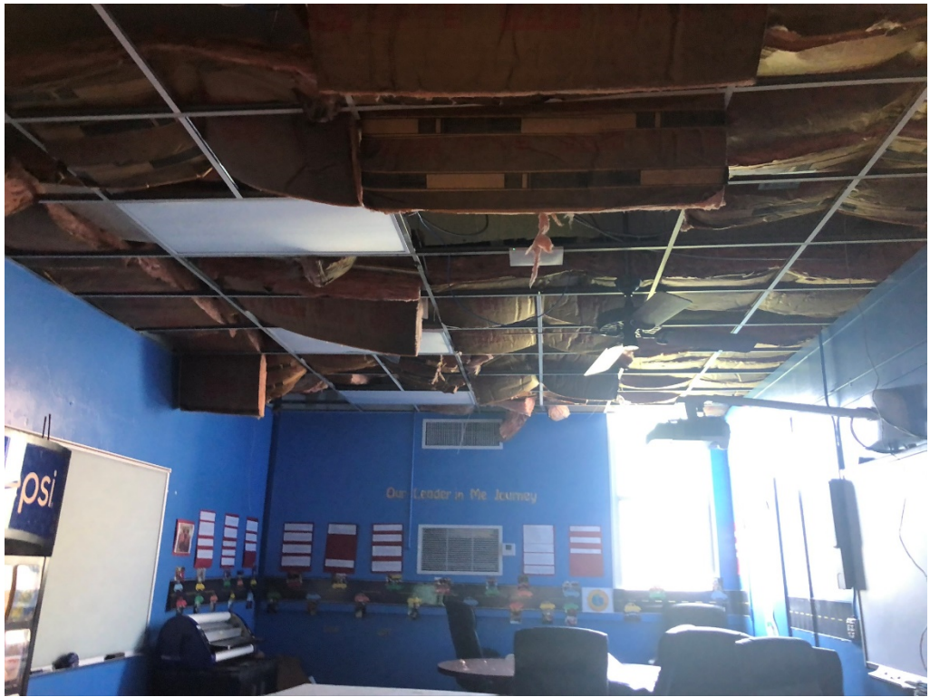
Figure 13 – Ceiling Demo Progress (Classrooms on North Section of Building)
