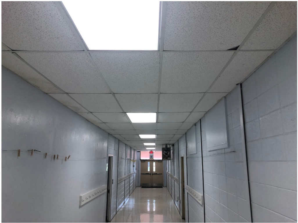
Figure 15 – North Section of Building
