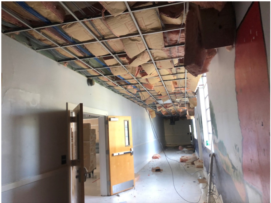
Figure 10 – Ceiling Demo Progress (Section A N/S Hall)
