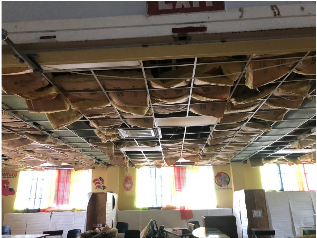
Figure 9 – Ceiling Demo Progress (Classrooms on South Section of Building)
