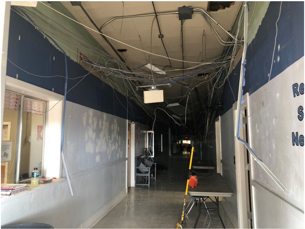
Figure 1 – Ceiling Demo Progress (Main Entry)
