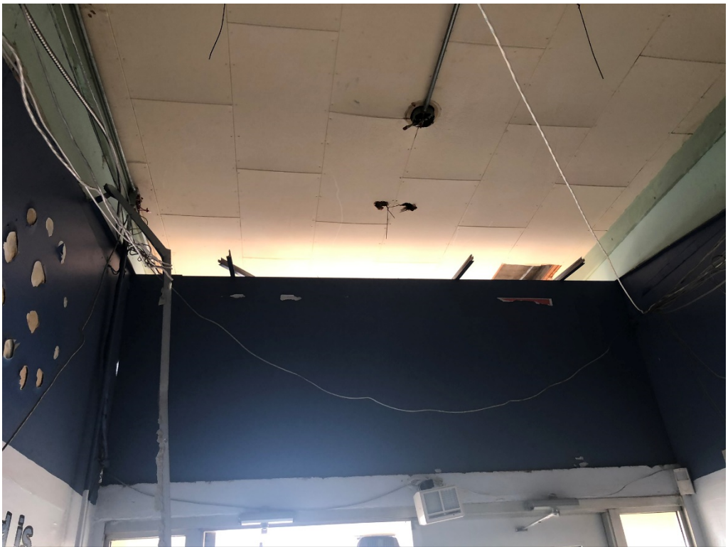
Figure 2 – Ceiling Demo Progress (Main Entry)
