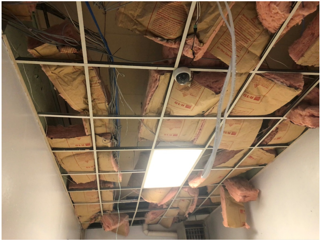
Figure 11 – Ceiling Demo Progress (Section A North Hall)
