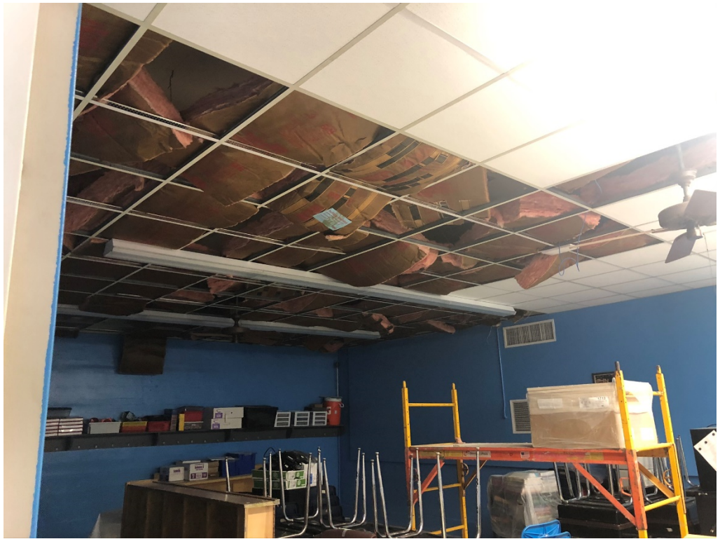
Figure 3 – Ceiling Demo Progress (Classrooms on South Section of Building)
