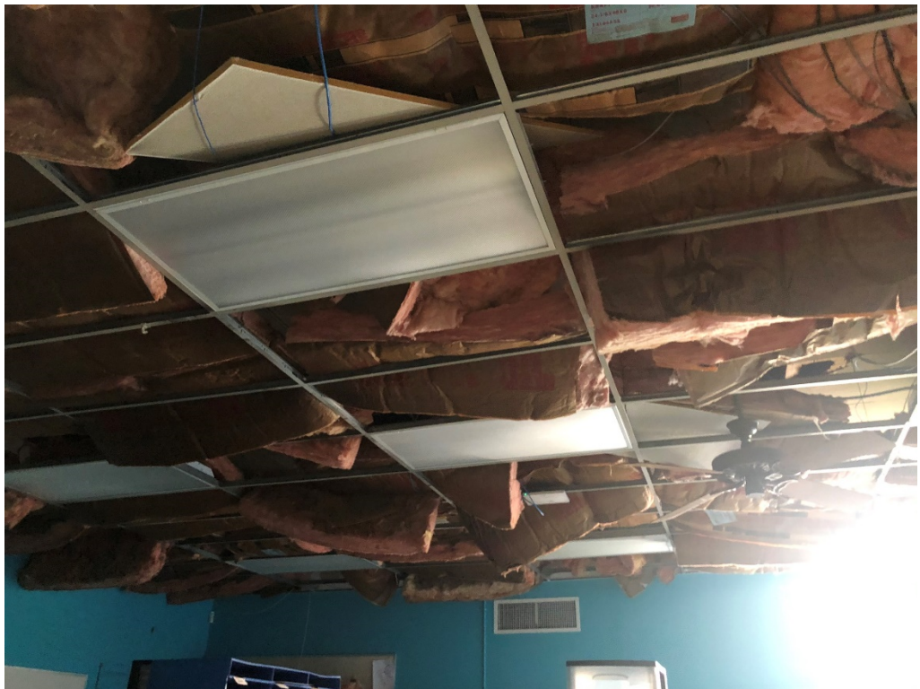
Figure 14 – Ceiling Demo Progress (Classrooms on North Section of Building)
