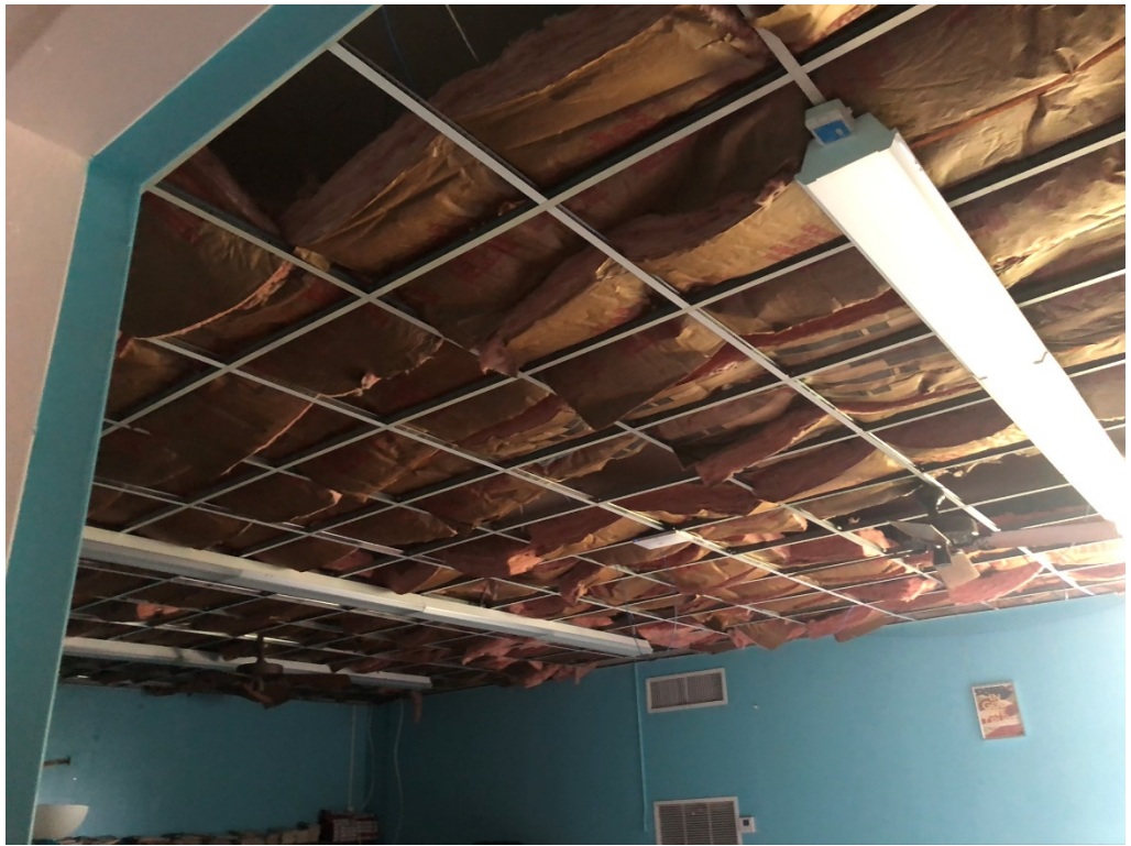
Figure 7 – Ceiling Demo Progress (Classrooms on South Section of Building)
