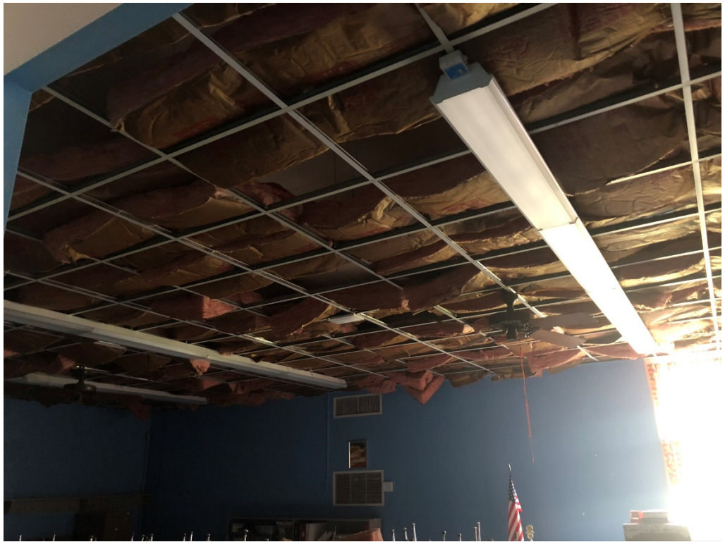
Figure 5 – Ceiling Demo Progress (Classrooms on South Section of Building)
