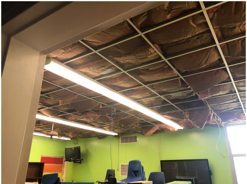
Figure 8 – Ceiling Demo Progress (Classrooms on South Section of Building)
