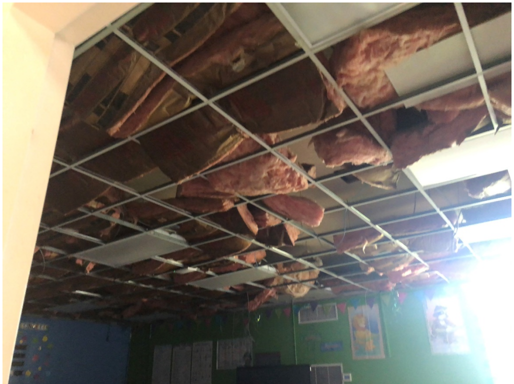
Figure 12 – Ceiling Demo Progress (Classrooms on North Section of Building)
