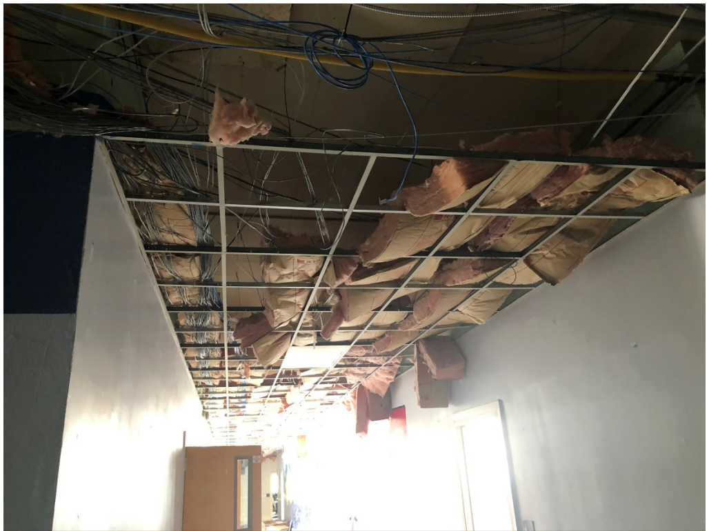
Figure 6 – Ceiling Demo Progress (Section A N/S Hall)
