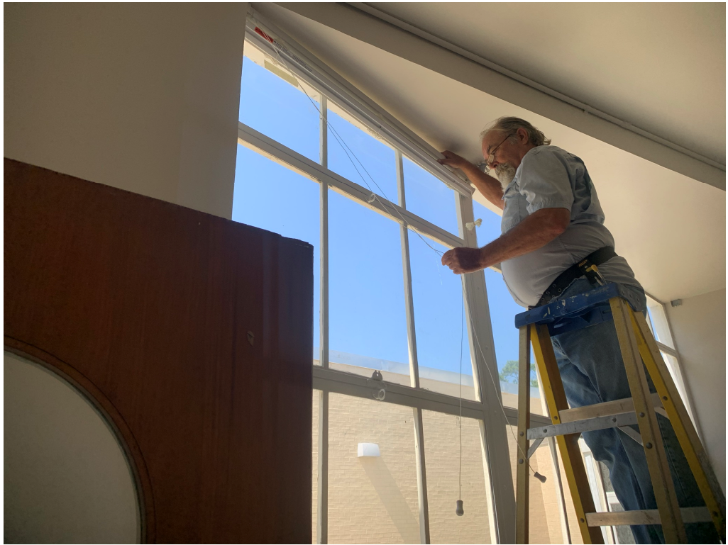
Figure 15 – Blind Installation is Ongoing
