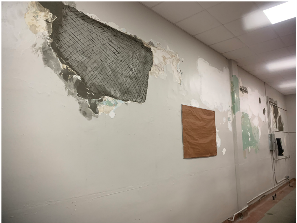
Figure 13 – Wall Patch and Repair in Cafeteria
