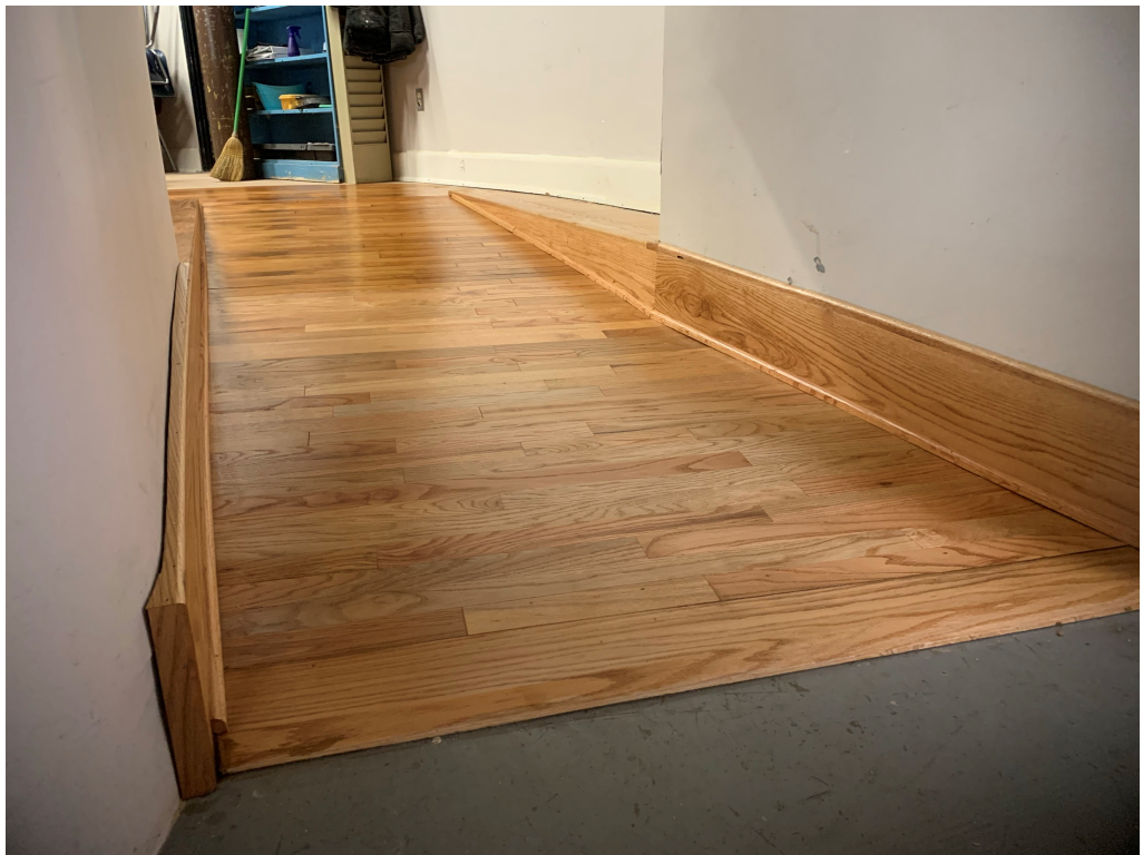
Figure 14 – New ADA ramps installed and Wood Finished
