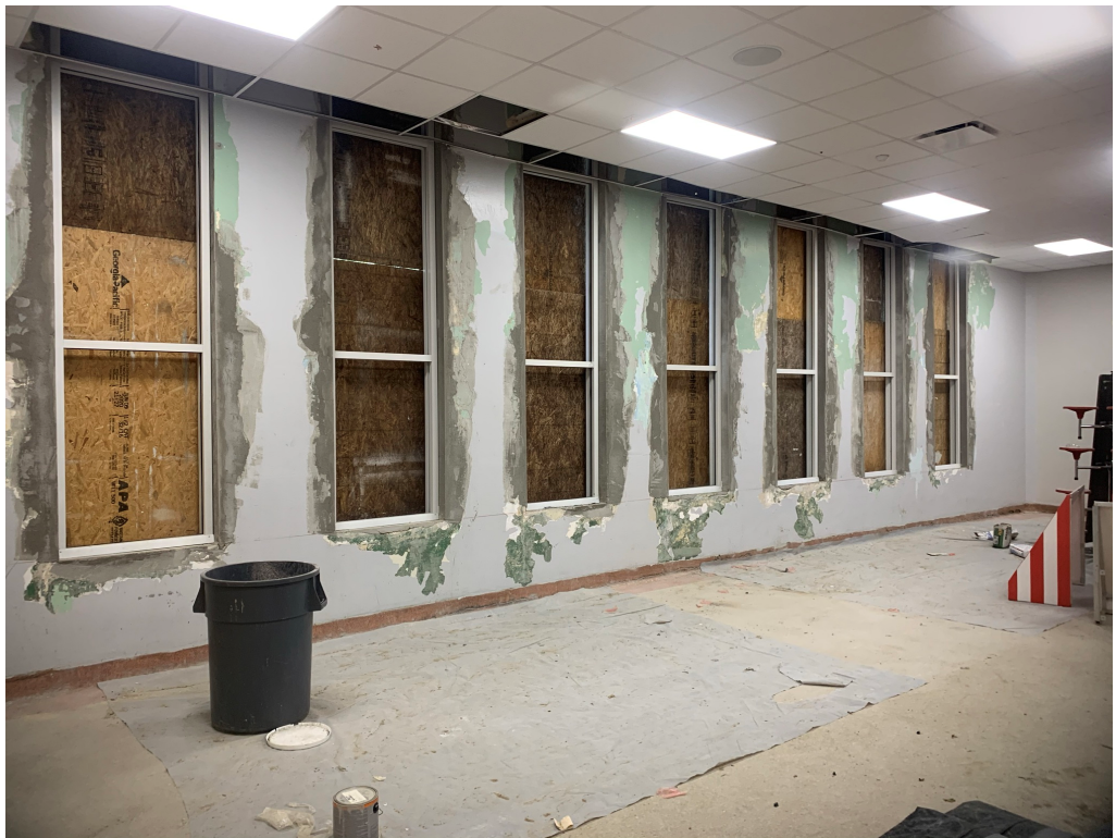
Figure 12 – Window Progress at Cafeteria Wall
