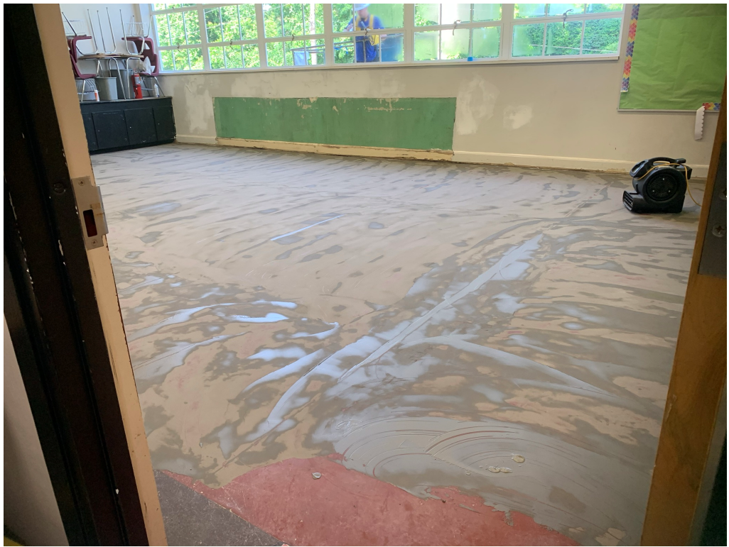
Figure 5 – Floor Prep at Laminate Floor @ 2 nd Floor
