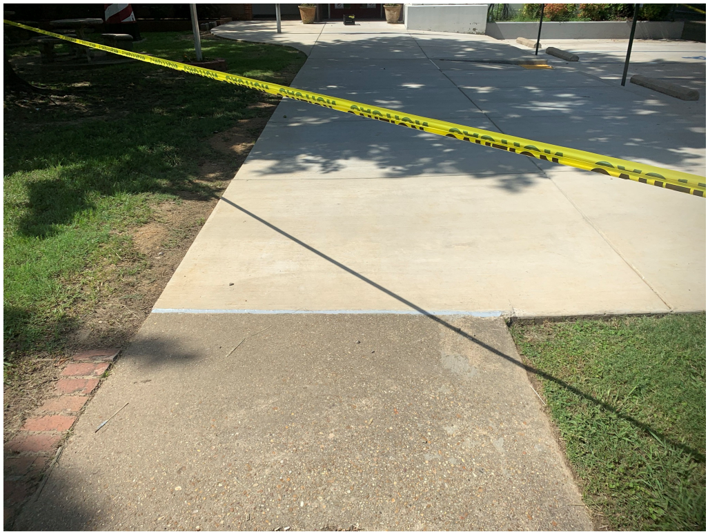
Figure 1 – Caulking at New Concrete
