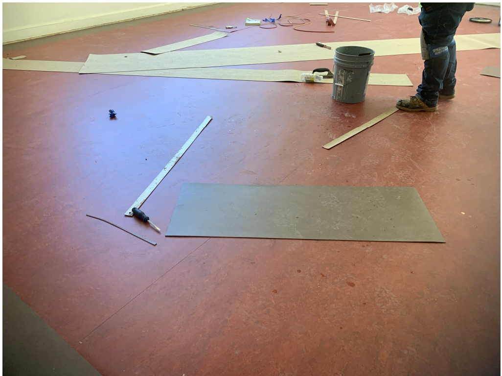
Figure 6 – Linoleum Floor Installation is Ongoing
