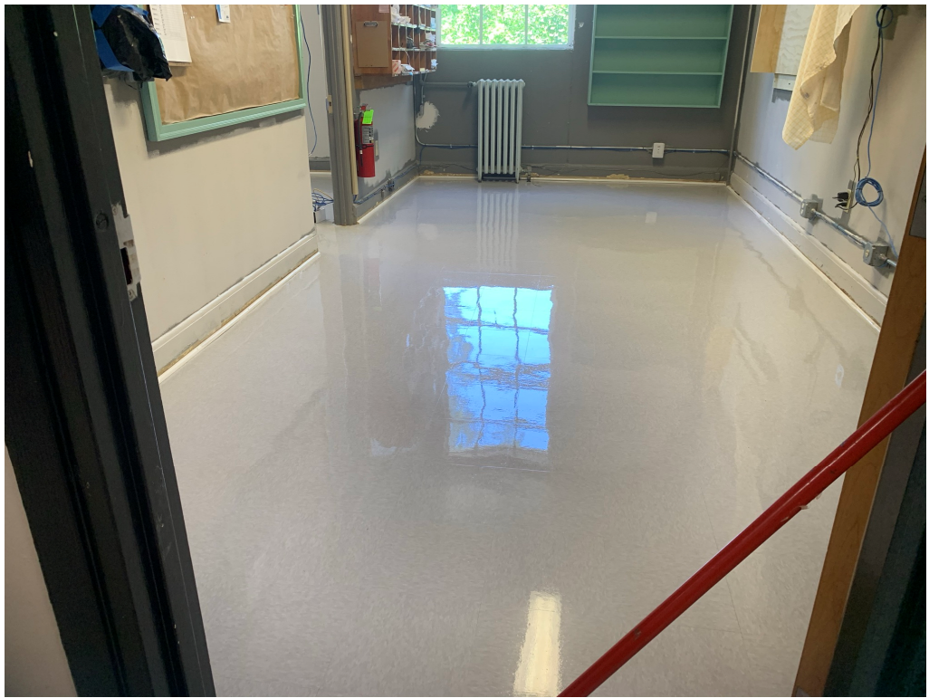
Figure 9 – Floor Wax Installation is Ongoing in Some Rooms
