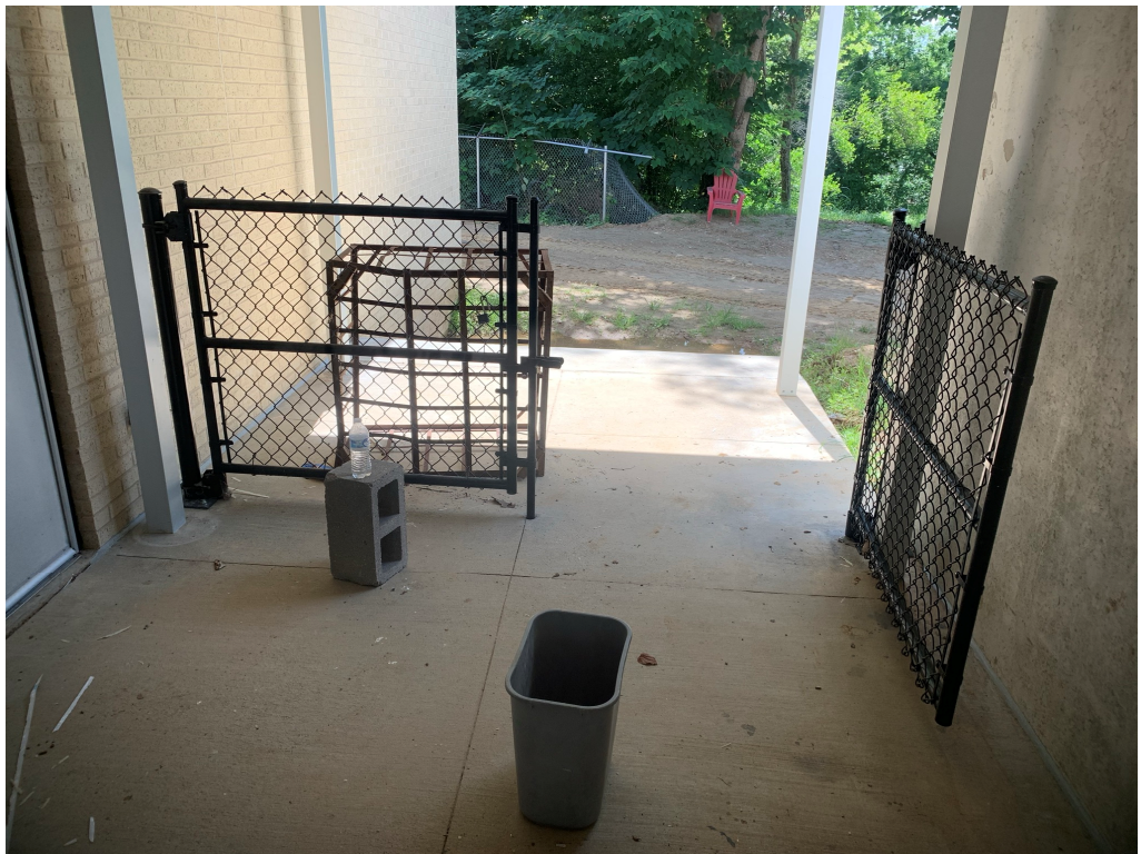
Figure 18 – Gates Installed at Breezeway
