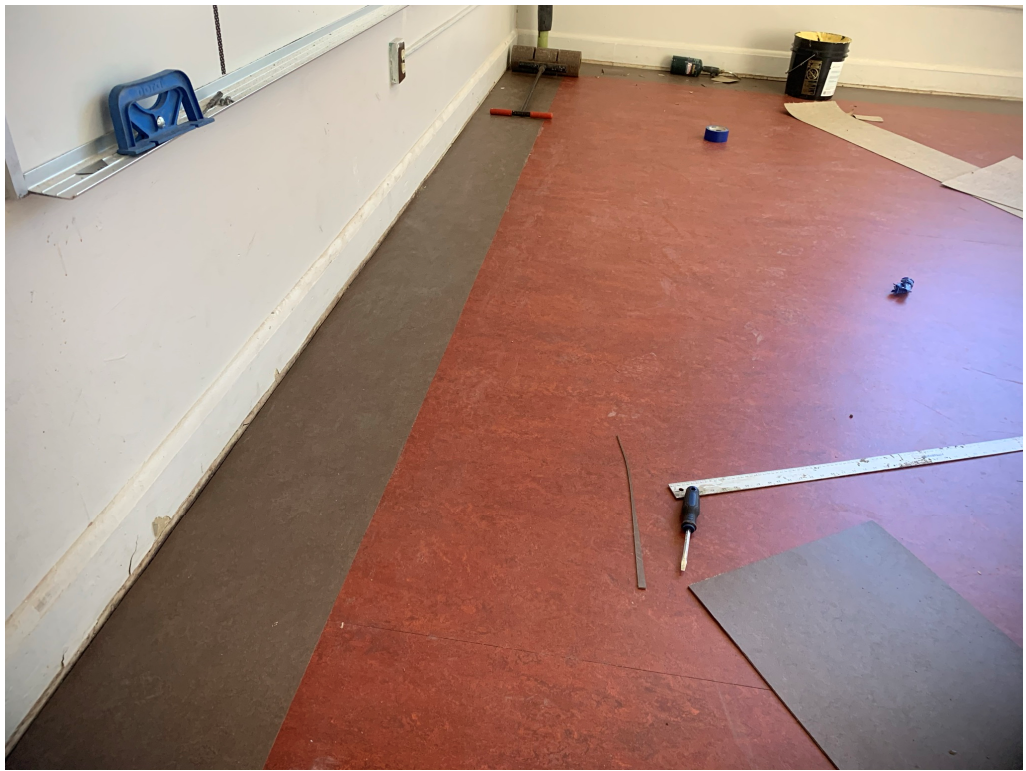
Figure 7 – New Linoleum Floor @ 2nd Floor
