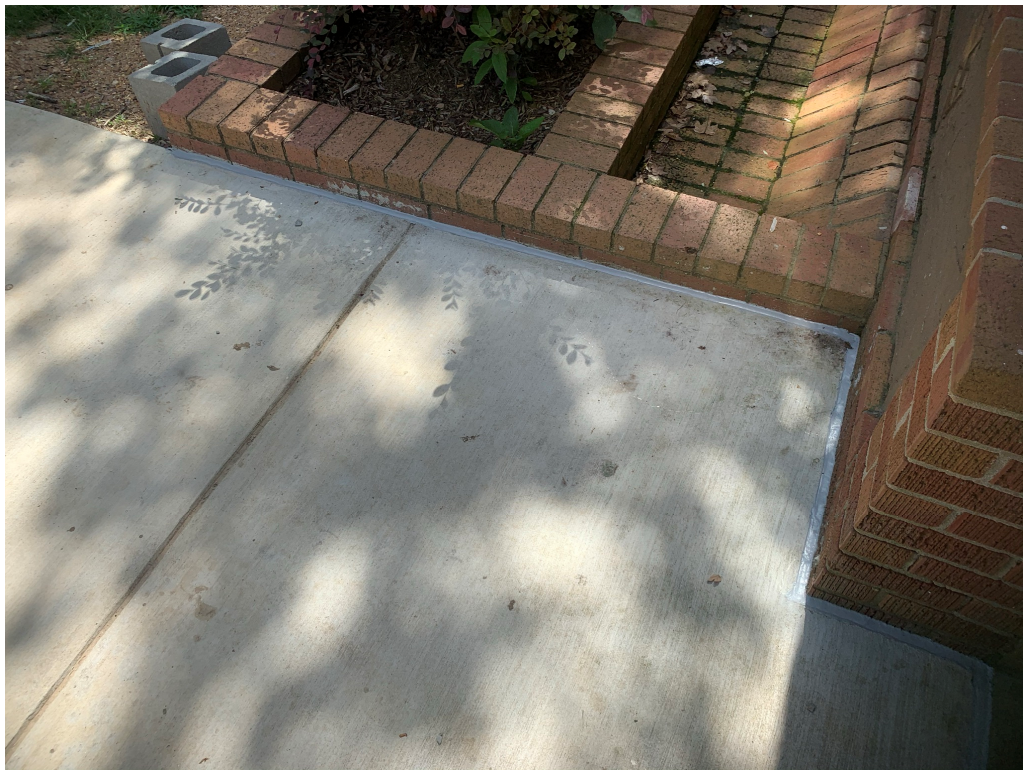
Figure 3 – Caulking at New Concrete
