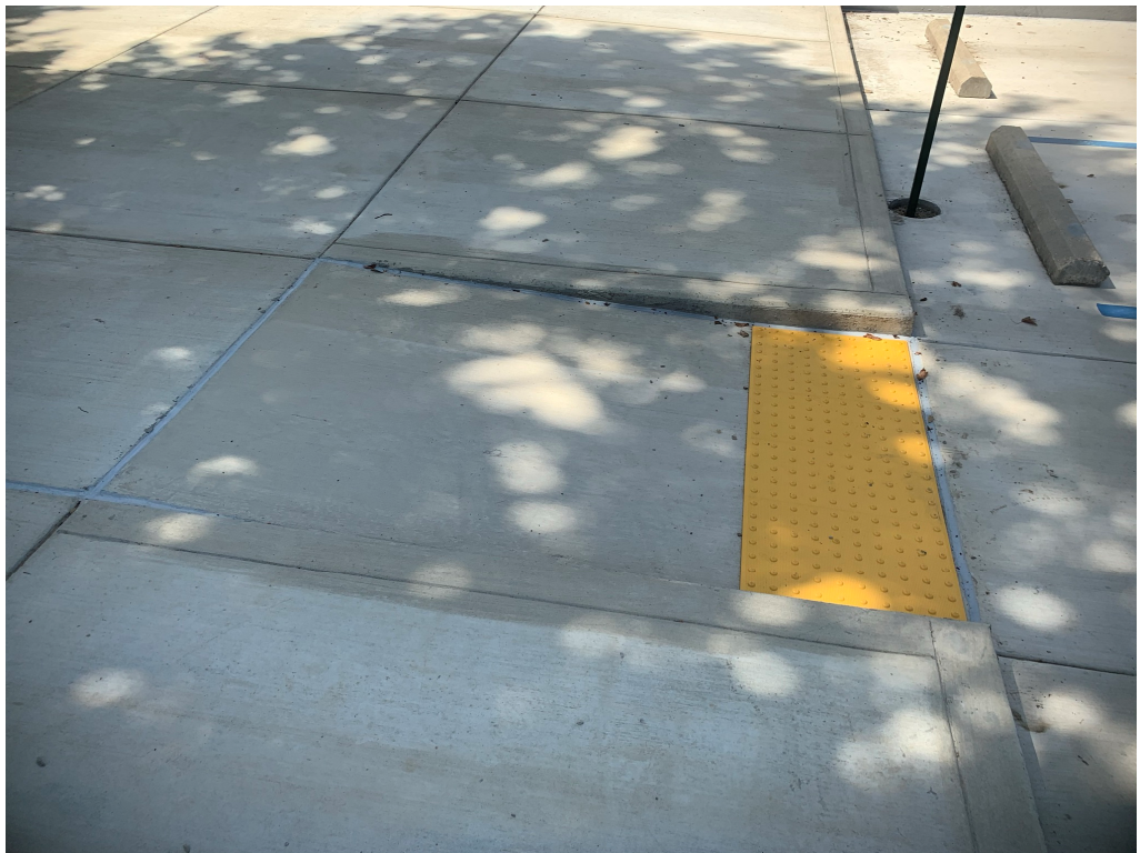
Figure 2 – Caulking at New Concrete
