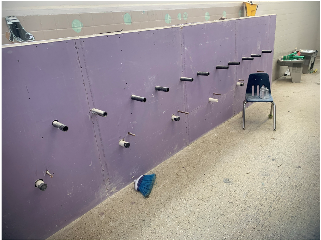
Figure 5 – Drywall Installed at Carrier Wall
