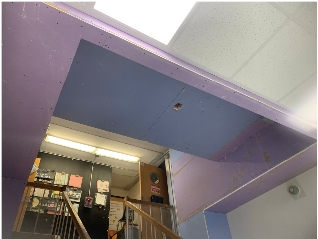
Figure 9 – Drywall Installed at Ducting
