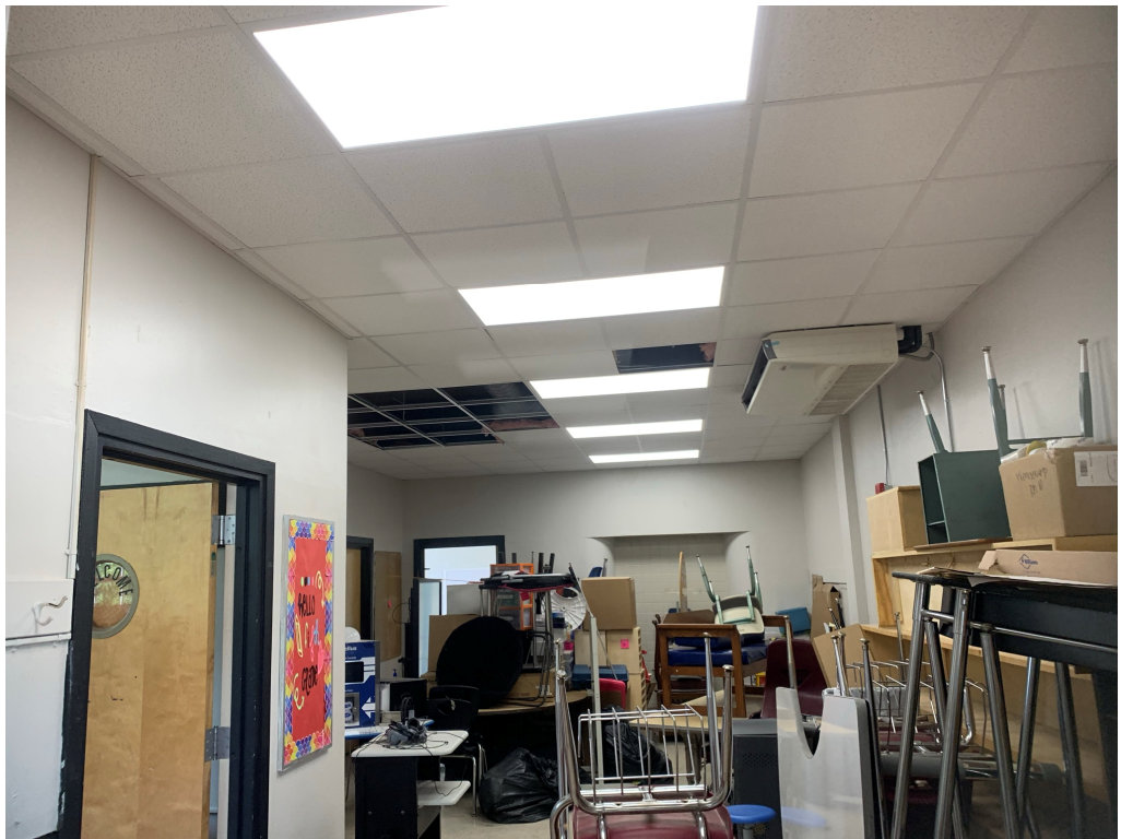
Figure 2 – ACT Installation at 2 nd Floor
