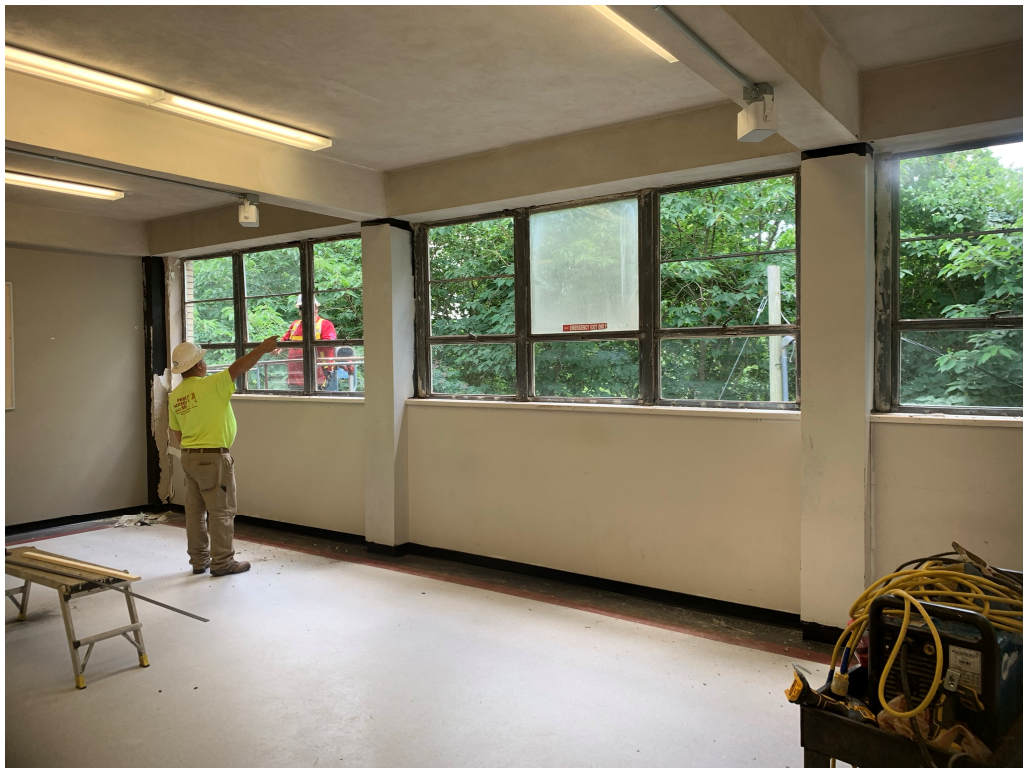
Figure 10 – Window Restoration in Progress
