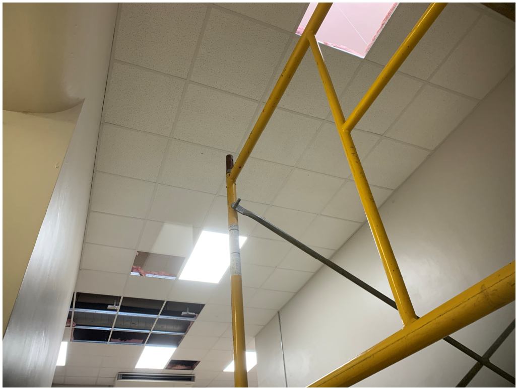
Figure 1 – ACT Installation at 2 nd Floor
