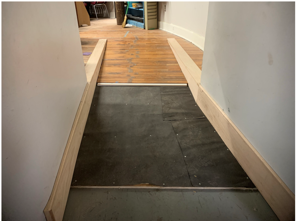
Figure 4 – ADA ramp Installation Progress
