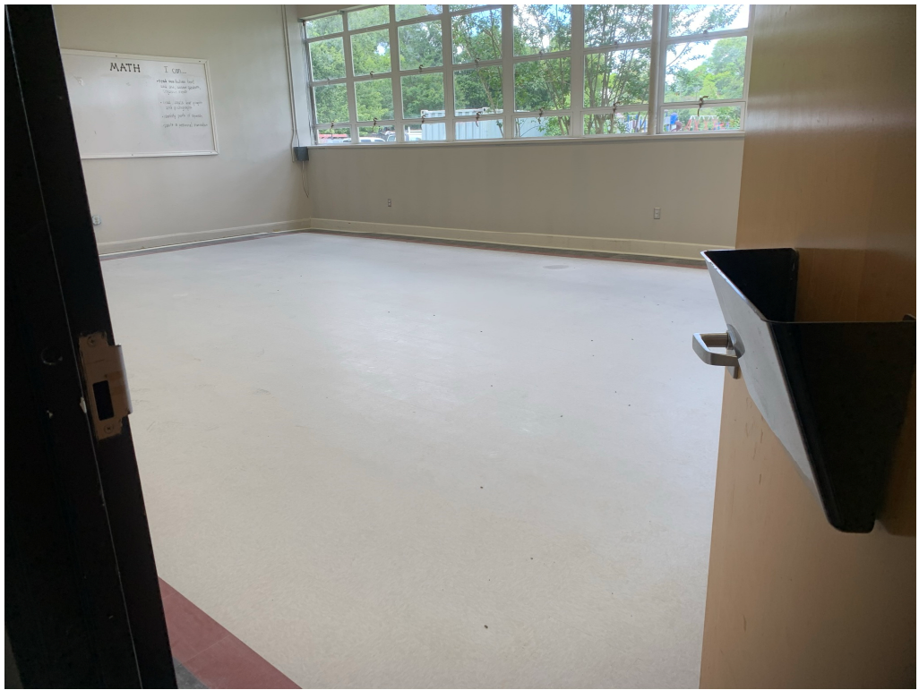
Figure 7 – VCT Installation is Ongoing
