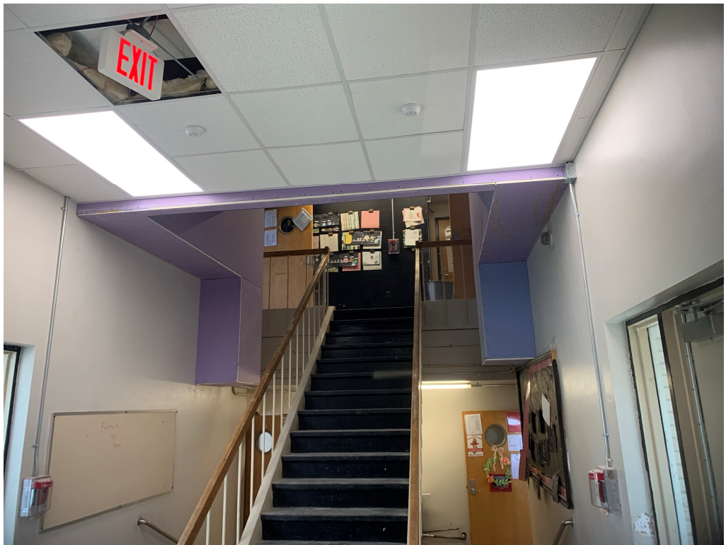
Figure 8 – Drywall Installed at Ducting
