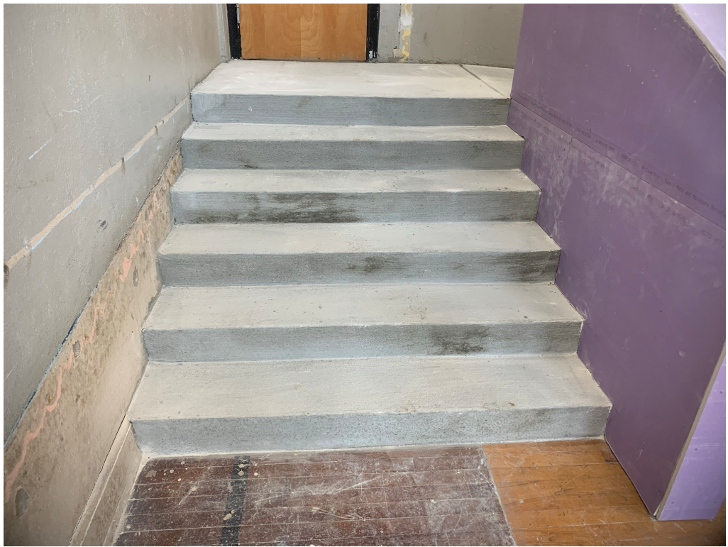
Figure 1 – Stairs at newly installed ADA ramp
