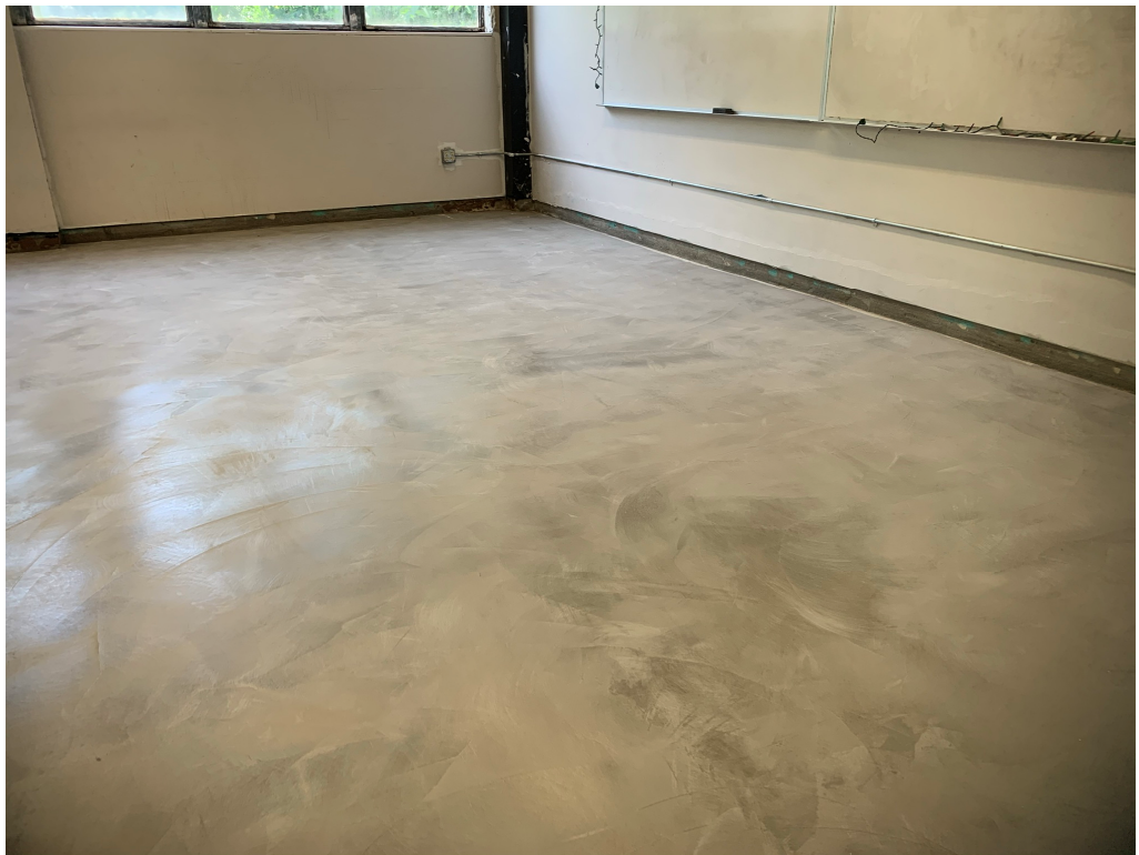
Figure 8 – Floor prep at classroom 24
