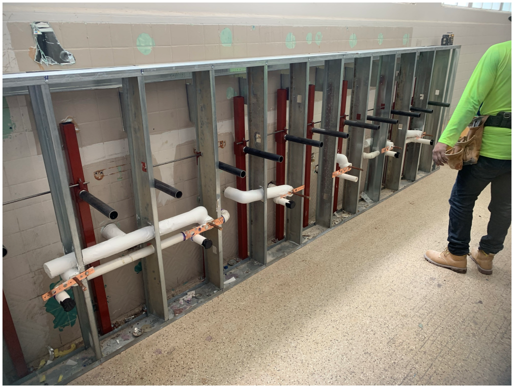
Figure 7 – Plumbing installed at Girls 29
