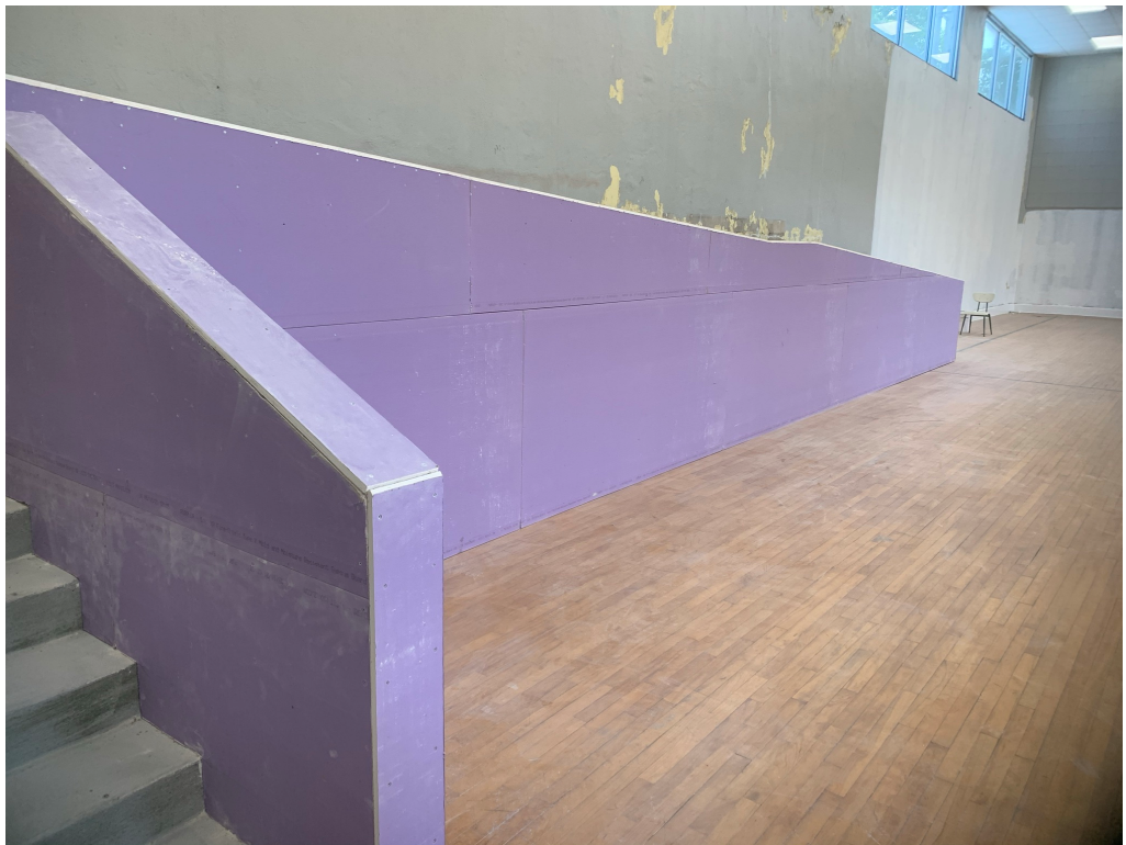
Figure 2 – Drywall installed at ADA ramp
