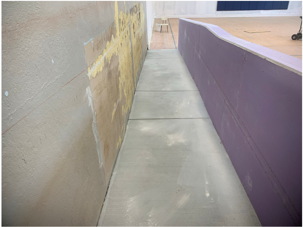
Figure 3 – ADA ramp installed at Playroom
