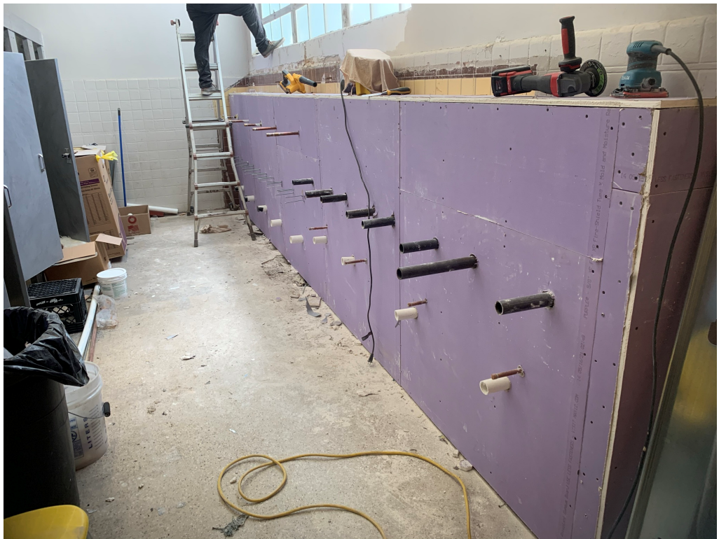
Figure 6 – Drywall Installed at Boys 30
