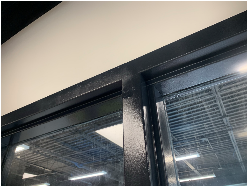
Figure 26 – Paint Build Up needs to be sanded out for smooth finish
