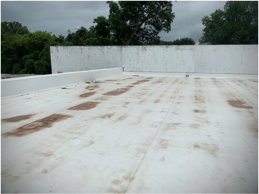
Figure 3 – Roofing Membrane appears in good condition
