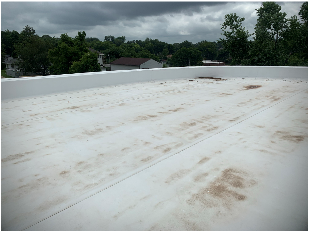
Figure 4 – Roofing Membrane appears in good condition
