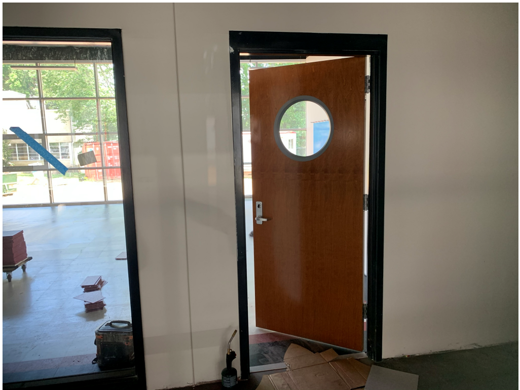
Figure 6 – Door Panels Installed
