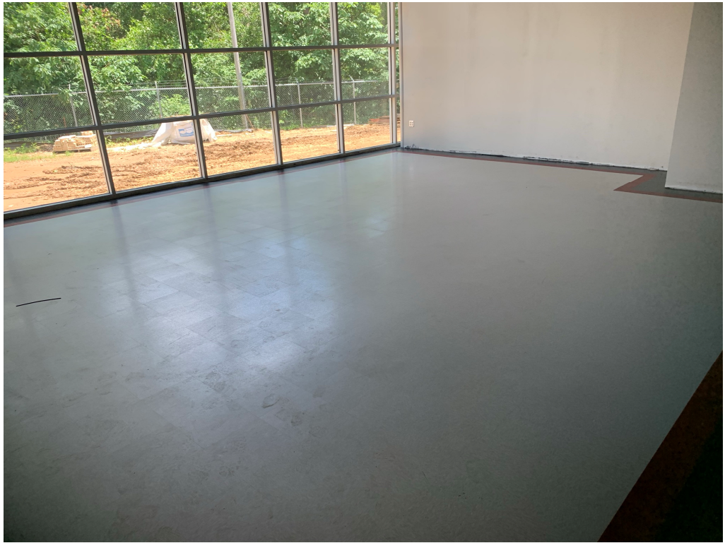
Figure 9 – New VCT Installed
