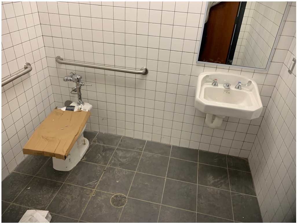
Figure 5 – ADA Bathroom Installed
