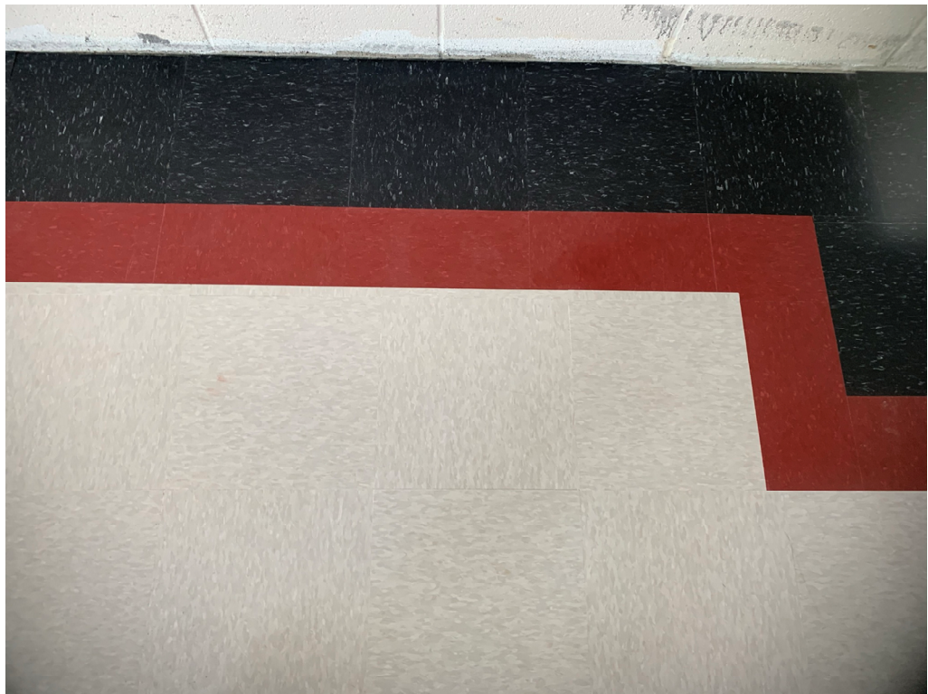
Figure 10 – New VCT Installed
