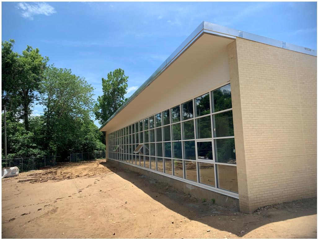
Figure 1 – Roof Trim Replaced to Match
