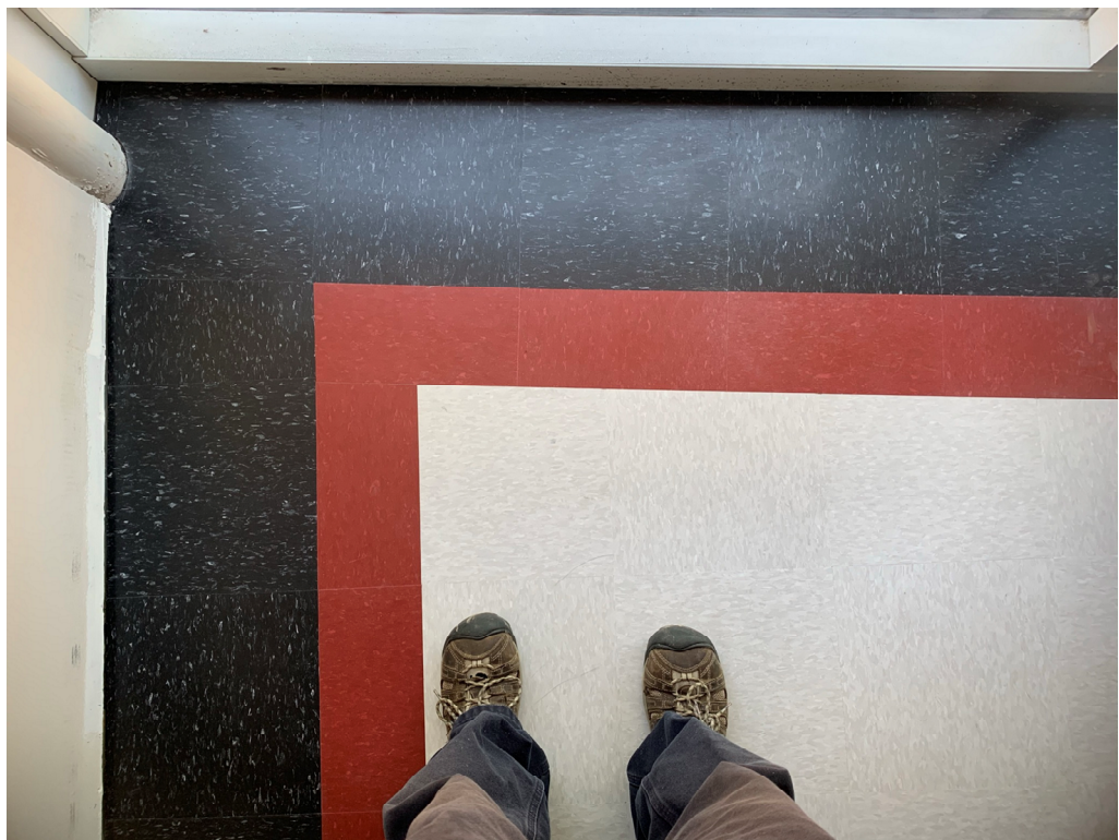
Figure 4 – New VCT Installed
