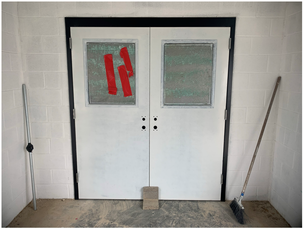
Figure 5 – Windows cut into doors
