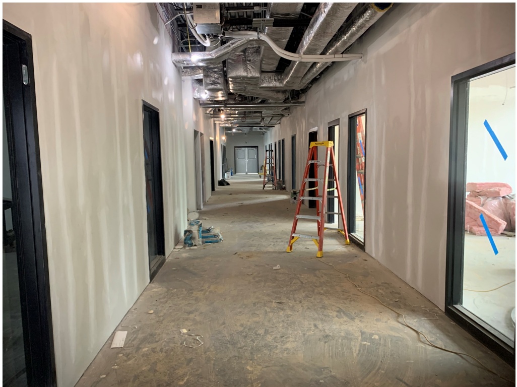
Figure 10 – Mud/Paint is ongoing
