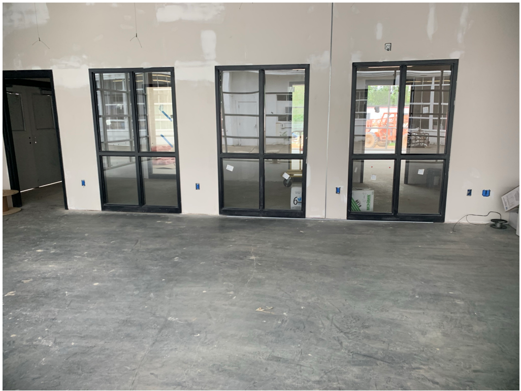
Figure 13 – Glazing Installed at Steel Interior Frames
