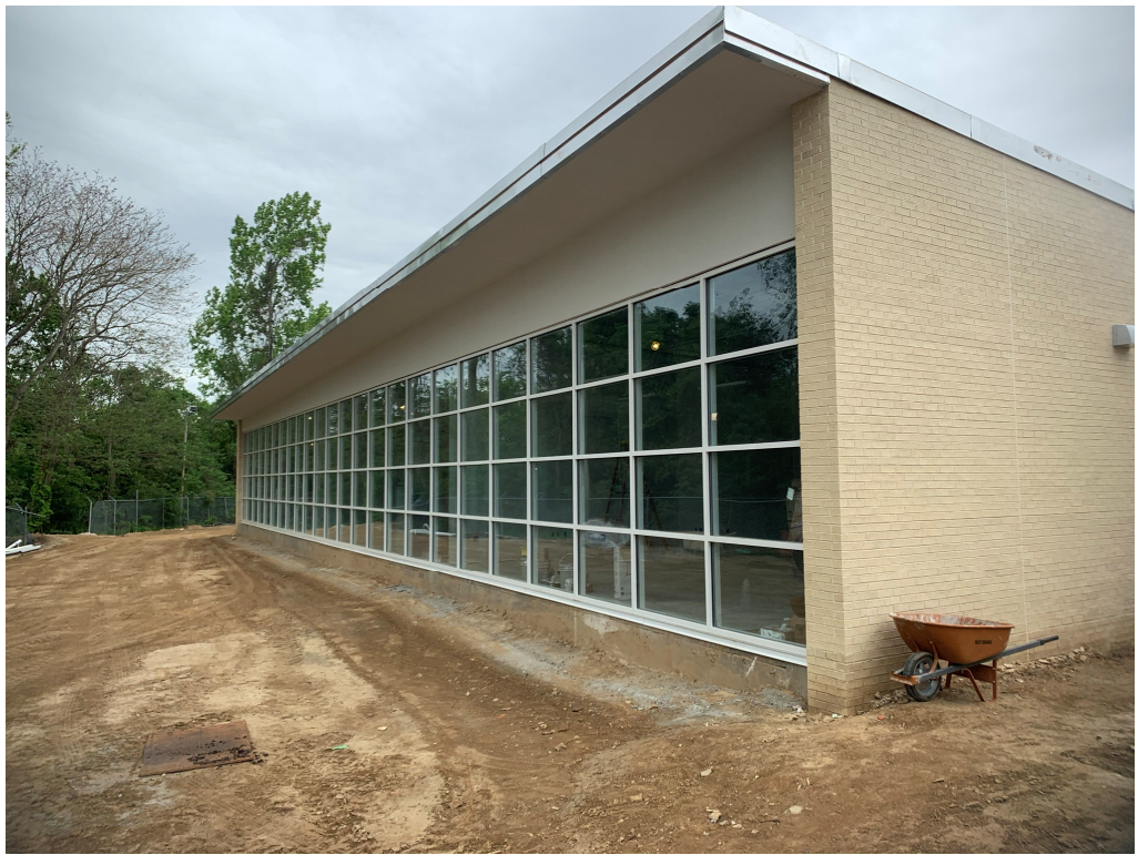
Figure 1 – East facing Facade
