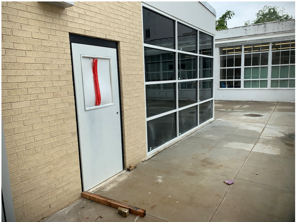
Figure 6 – Windows cut into doors
