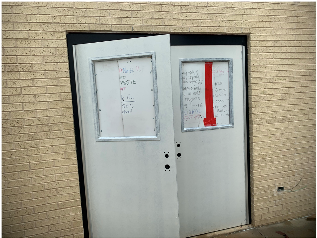
Figure 9 – Windows cut into doors
