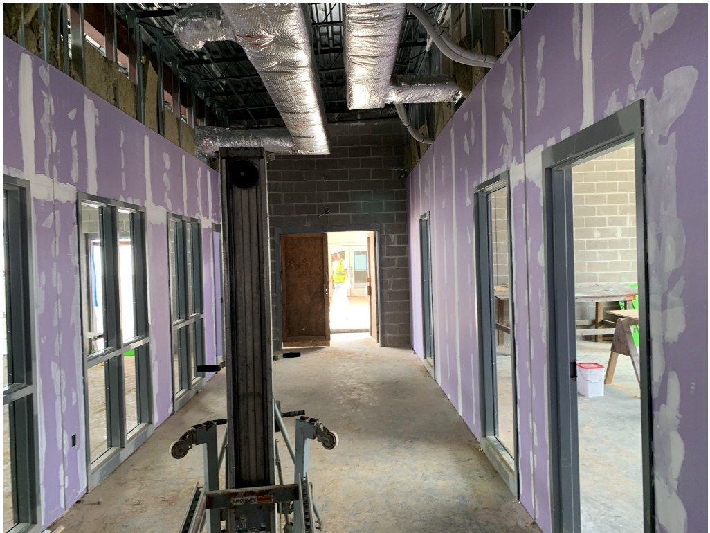
Figure 2 – Hall Looking toward front of School
