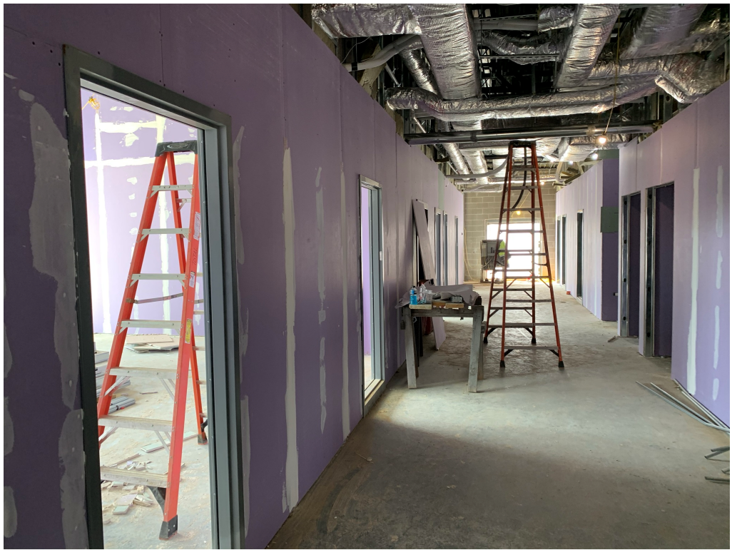
Figure 3 – Hall Looking toward Gym
