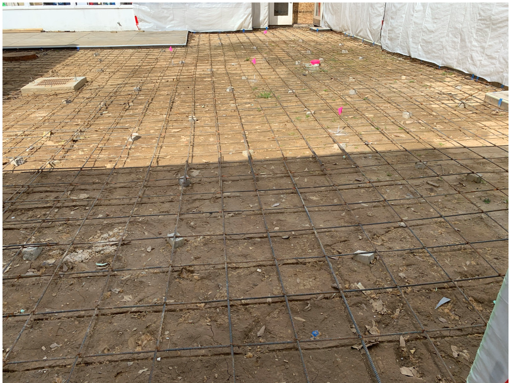
Figure 6 – Rebar lifted in place ready for concrete
