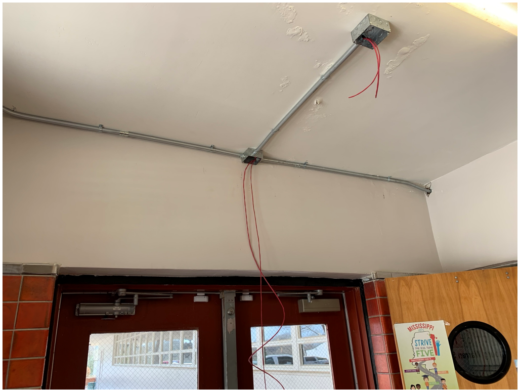
Figure 1 – Alarm Installation wire pulls at Entry Foyer
