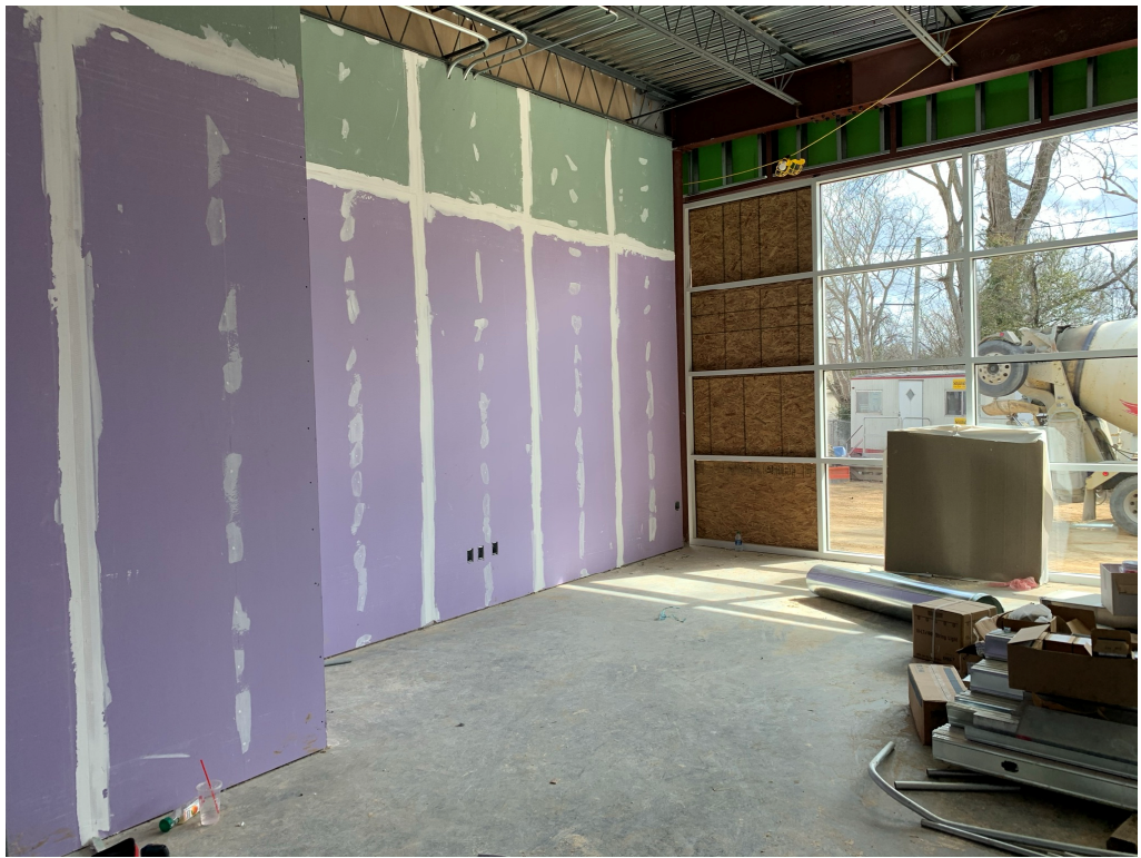
Figure 5 – Top of wall where joist conflict to be boxed in with drywall
