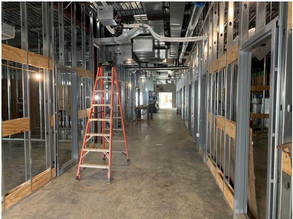
Figure 6 – Service Work is Ongoing
