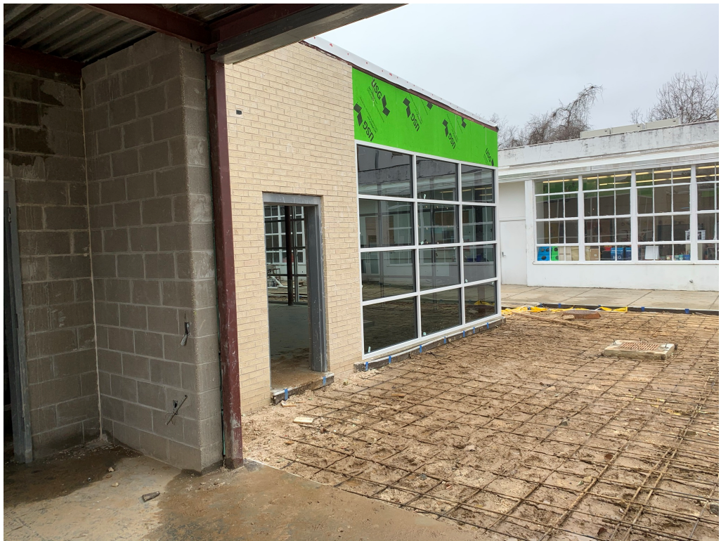
Figure 8 – New Storefront Installed
