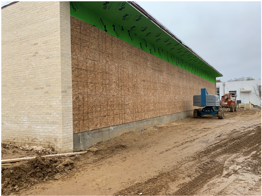
Figure 5 – SE Façade; temporary osb installed
