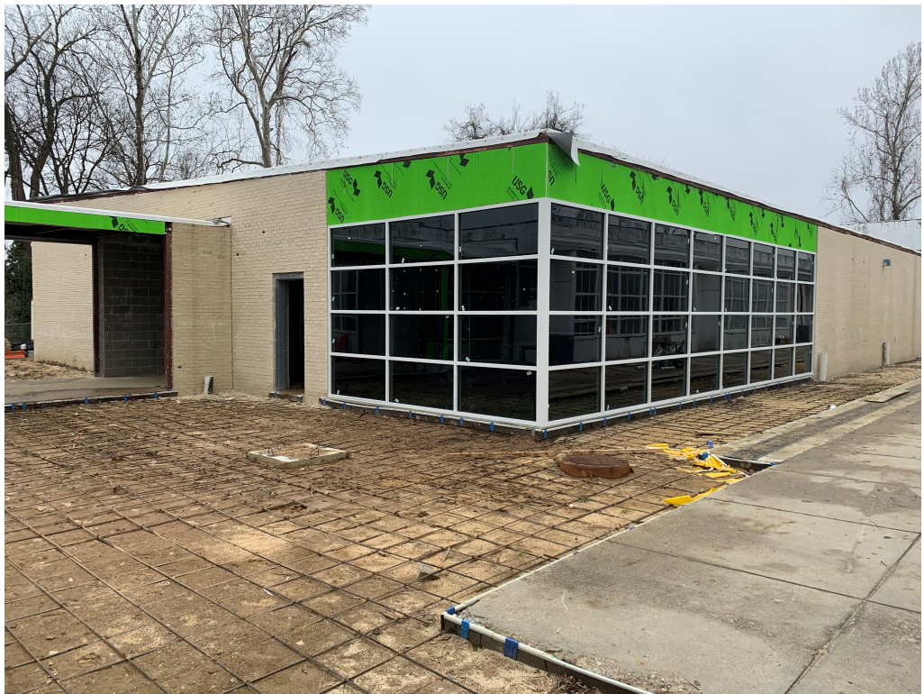
Figure 2 – New Storefront Installed
