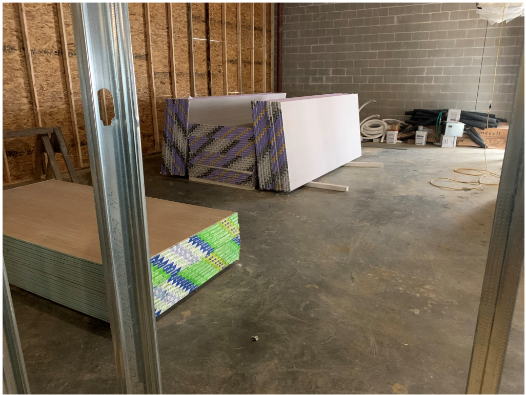
Figure 7 – Drywall On Site
