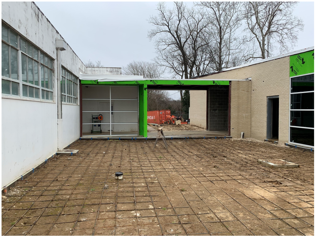
Figure 1 – Courtyard at New Addition
