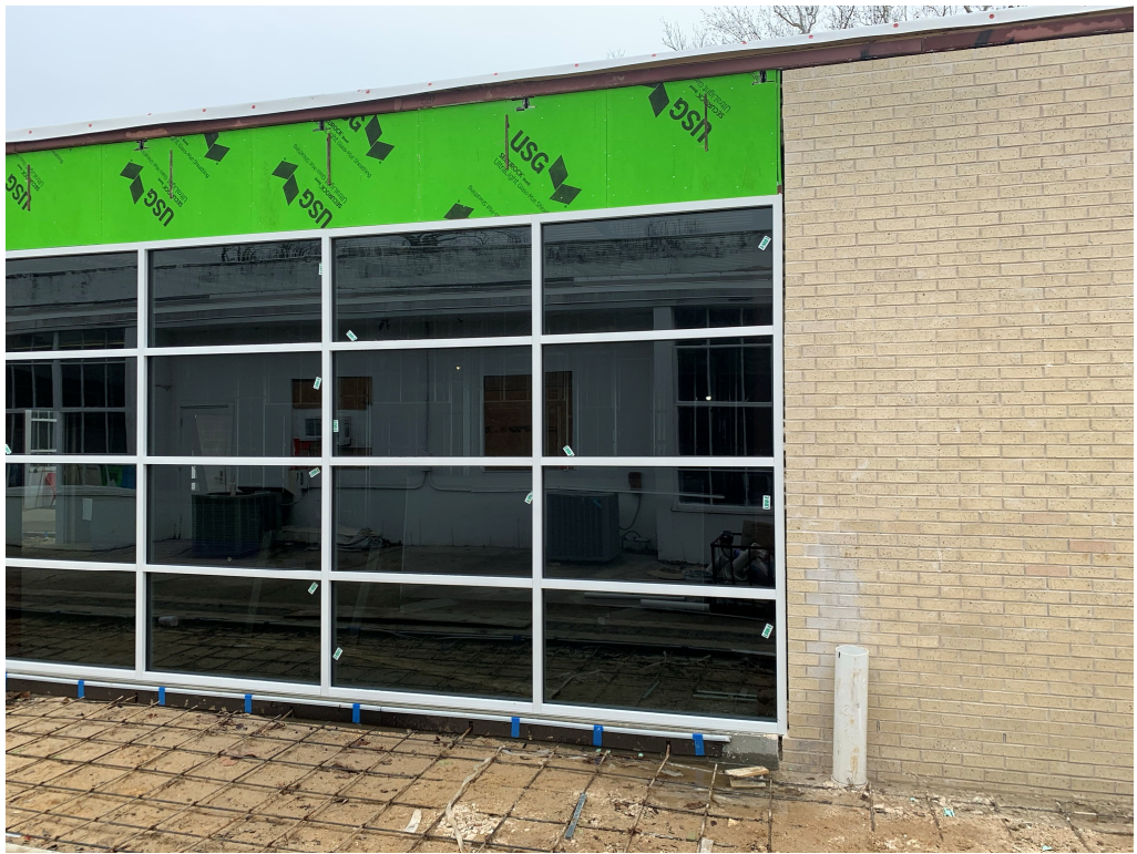
Figure 3 – New Storefront Installed
