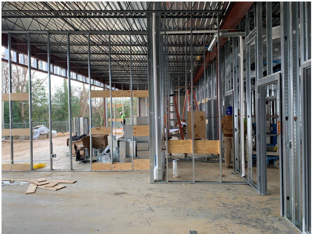
Figure 6 – Plywood Blocking Installed
