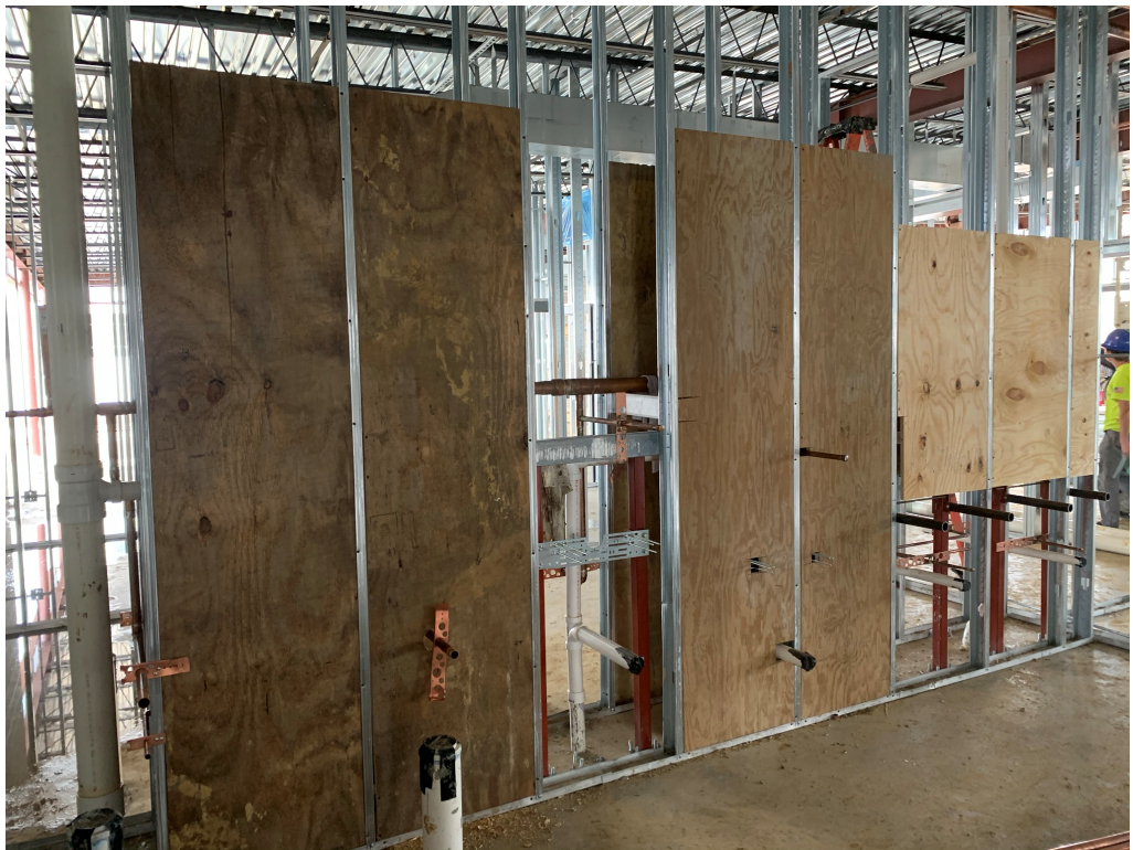
Figure 10 – Plywood Blocking Installed
