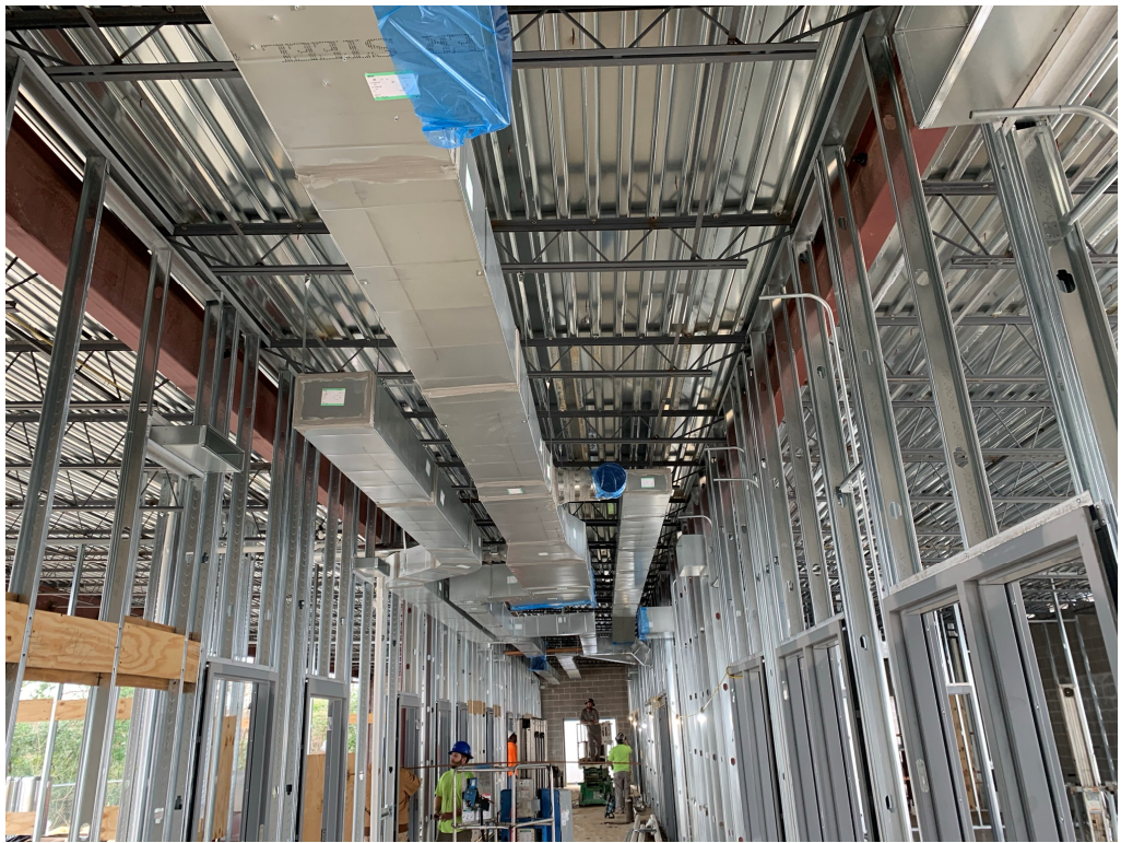
Figure 5 – HVAC Ducting is Ongoing
