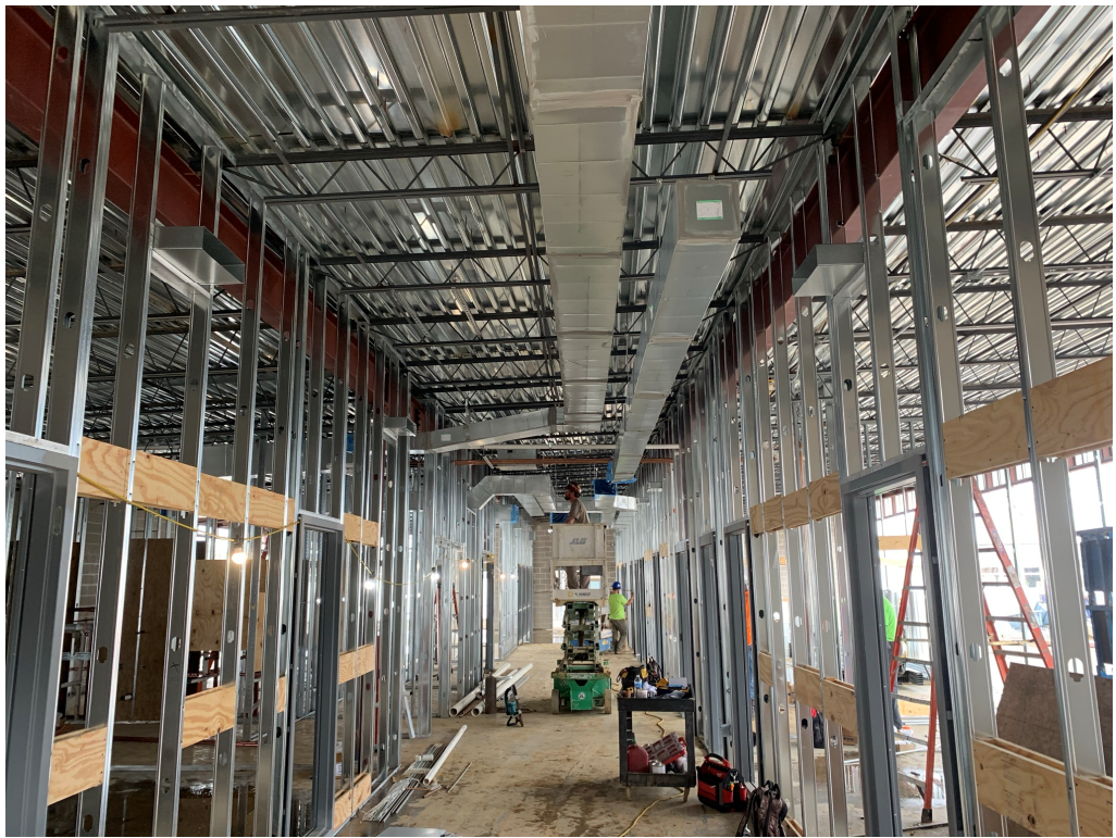
Figure 9 – HVAC Ducting is Ongoing
