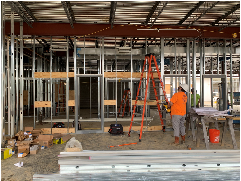
Figure 7 – Plywood Blocking Installed
