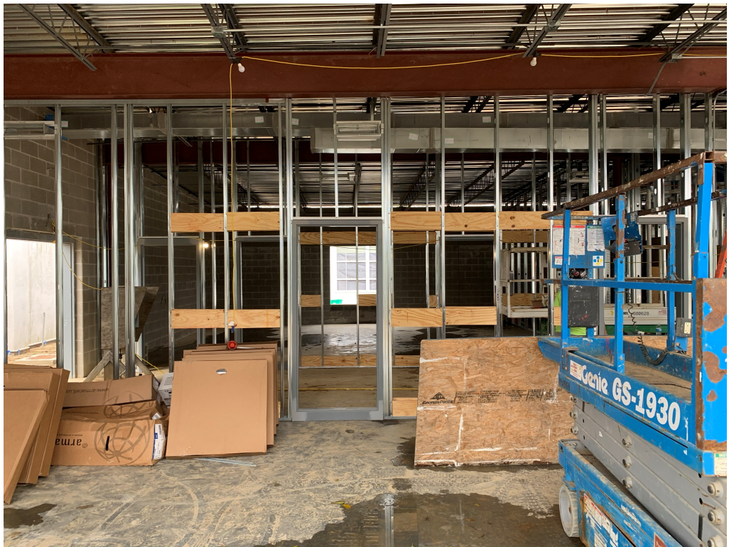
Figure 8 – Plywood Blocking Installed
